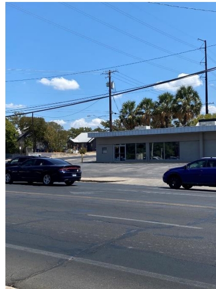
Photo 24: Map ID 12, a Moderate Risk site. Photograph was taken from 38 th St and Guadalupe facing southeast.
