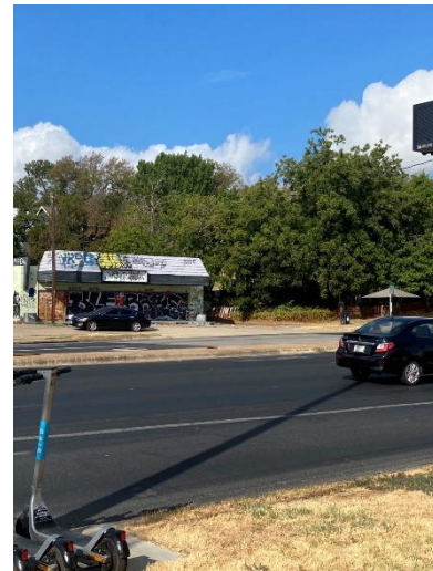
Photo 12: Map ID 457, a Low Risk site. Photograph was taken from E. Riverside Drive, facing southeast.
