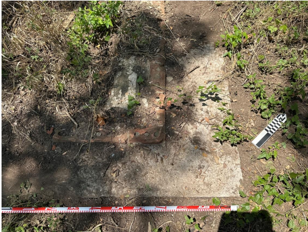
Figure 43: Foundation (F01) close up, facing northwest
