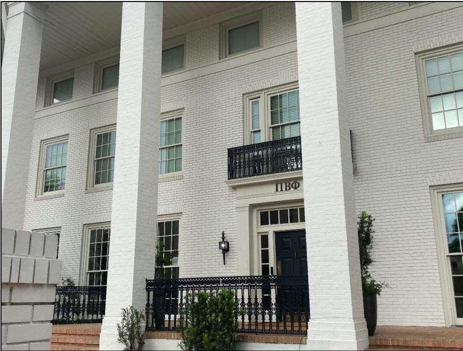
Detail of the primary entry of Resource S158, looking southwest.
