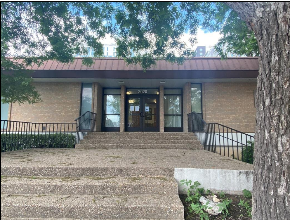
View of the façade entry of Resource S165, looking west.
