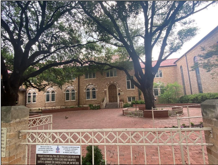
View of the interior of the courtyard and the west elevation of the original building, looking east.
