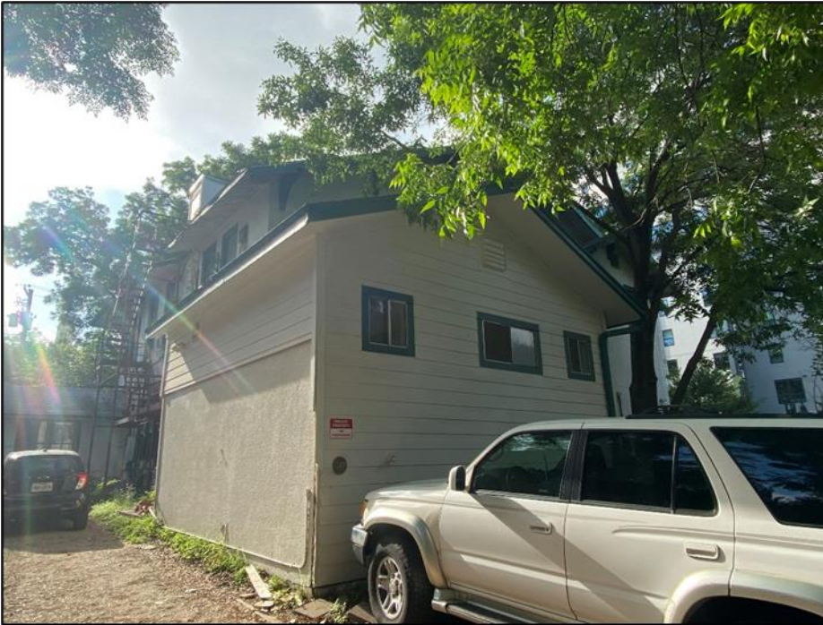
Oblique view of the addition to the west elevation of Resource 159, looking southeast.
