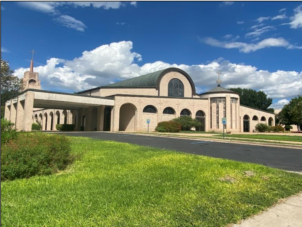
Façade view of Resource S196c, looking north.
