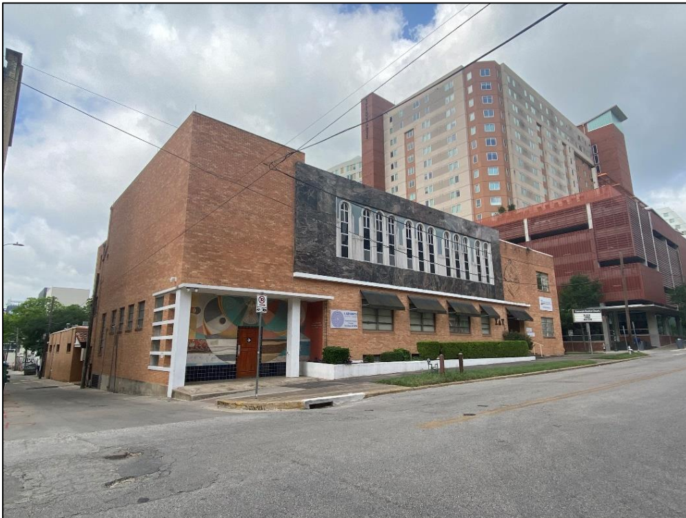
View of the façade of Resource S164, looking southwest.
