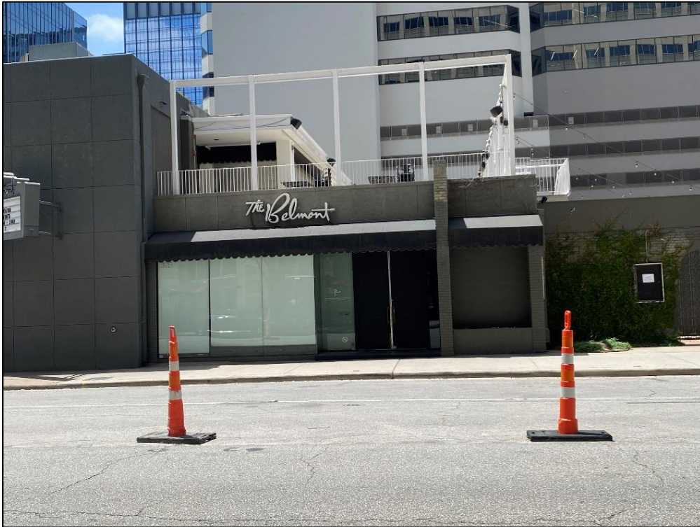
View of center of the façade, looking south (IMG_1731).
