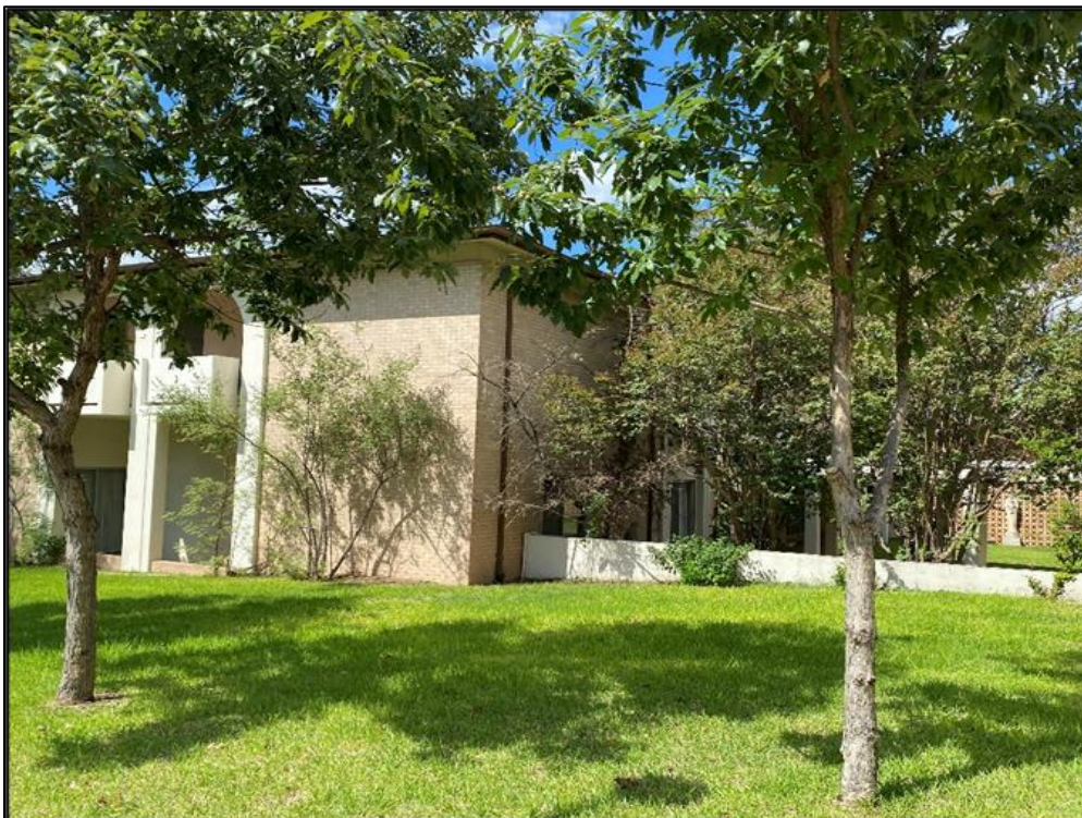
Oblique view of the façade and the south elevation of Resource S196d, looking northeast.
