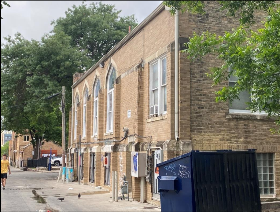
View of the east elevation of Resource S160, looking south.
