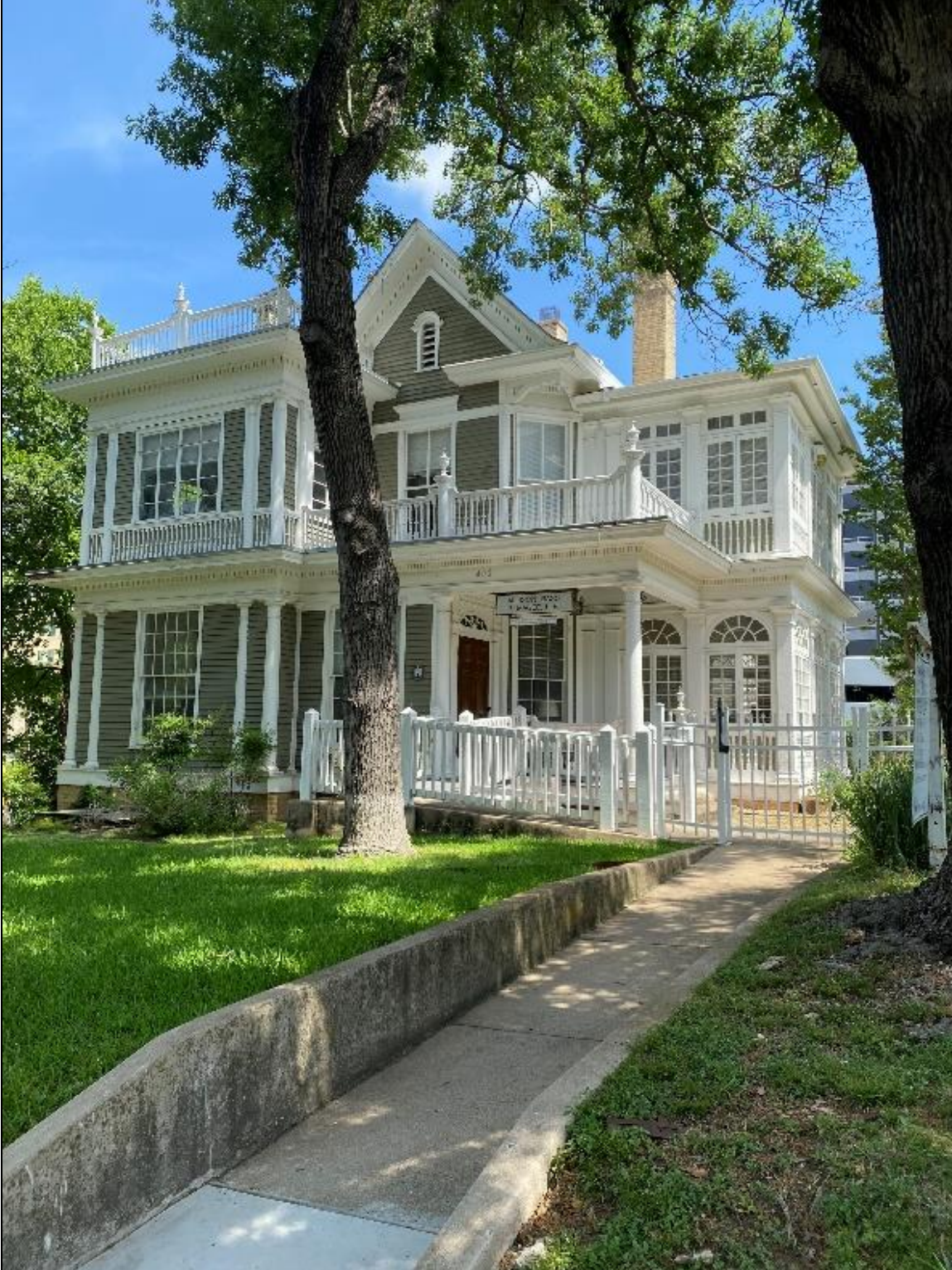
Facade view of Resource S182, looking northwest.
