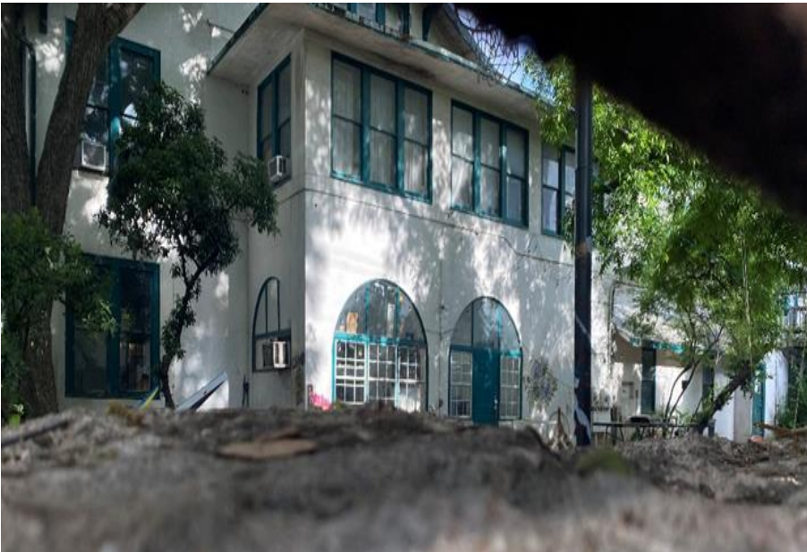
View of the rear (east) elevation of Resource S159, looking northwest.
