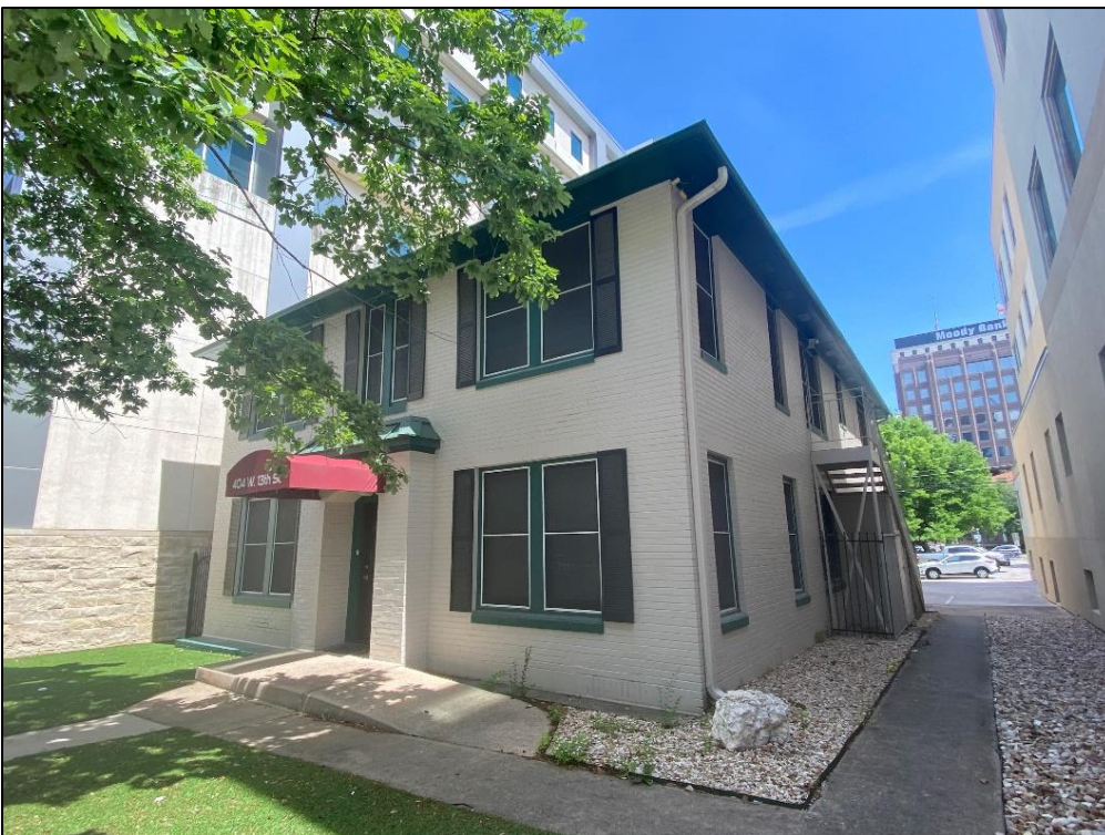
Oblique view of the facade and the east elevation of Resource S176, looking northwest.
