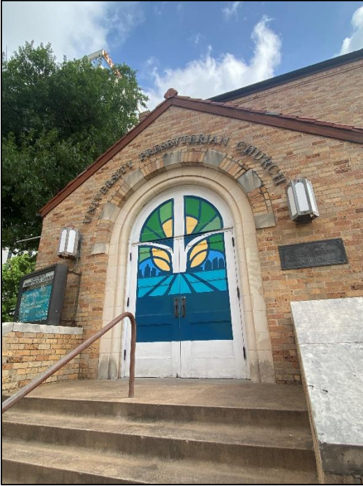
Detail of the sanctuary entrance on the south elevation, looking north.
