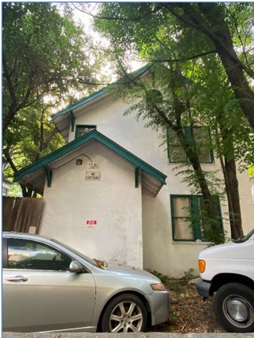
View of the façade of Resource S157, looking east.
