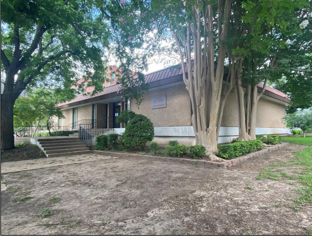
Oblique view of the façade and the north elevation of Resource S165, looking southwest.
