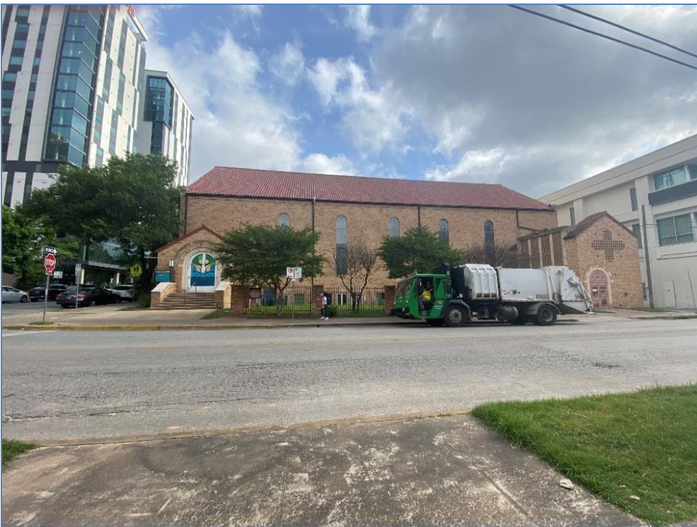
View of the south elevation of Resource S162, looking north.
