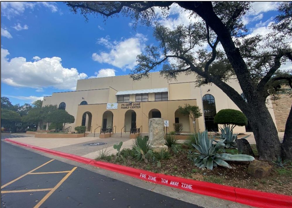
View of the west elevation of Resource S196a, looking east at the 1987 addition.
