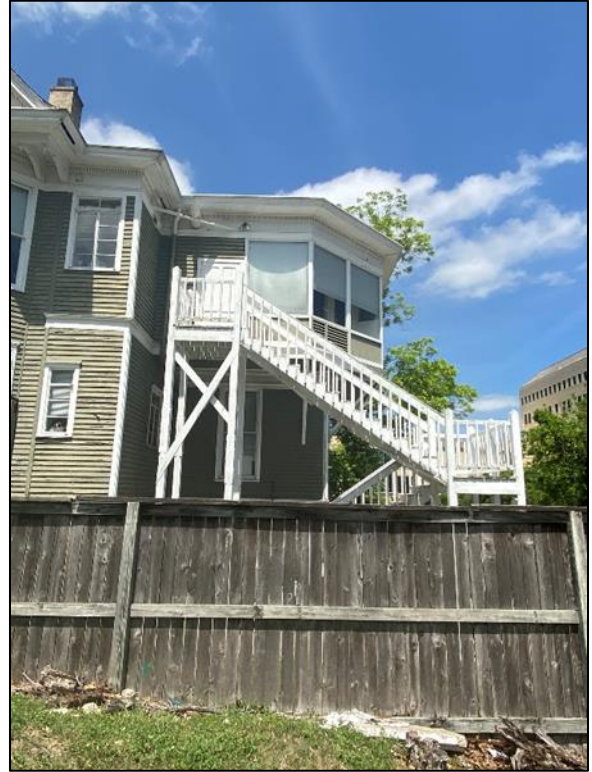
View of the east side of the rear elevation.
