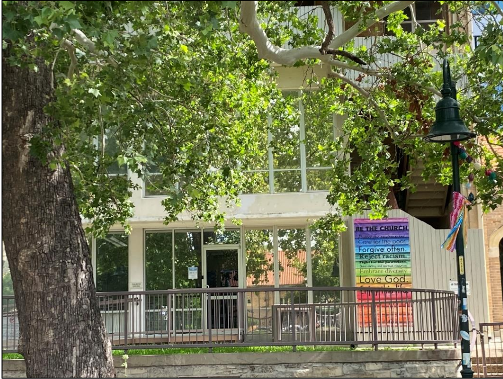
View of the façade of the educational wing of Resource S160, looking north.
