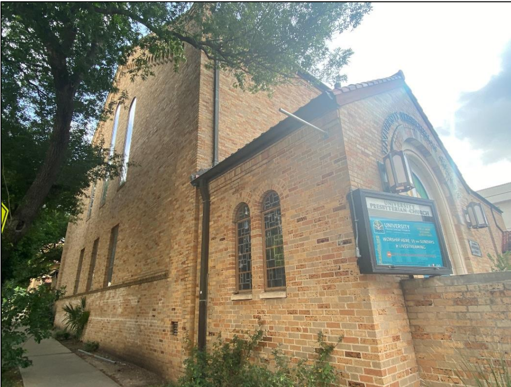
Oblique view of the south and the west elevations, looking northeast.
