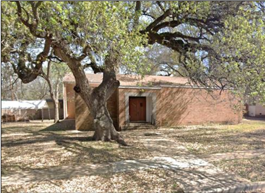
Façade view of Resource S196b, looking east (Google Image 2021).
