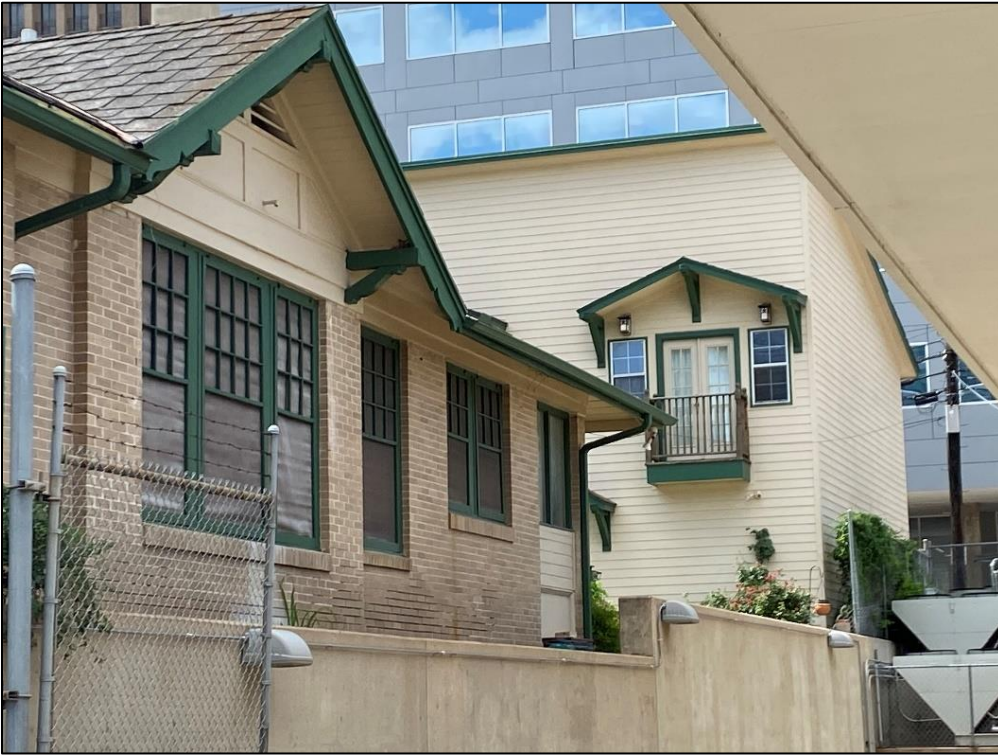
View of the ancillary building at the rear of Resource S181, looking south.
