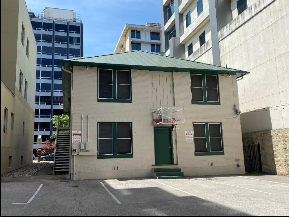
View of the rear (north) elevation of Resource S176, looking south.
