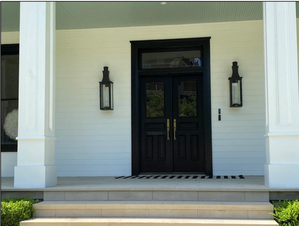
Detail of the entry Resource S172, looking south.
