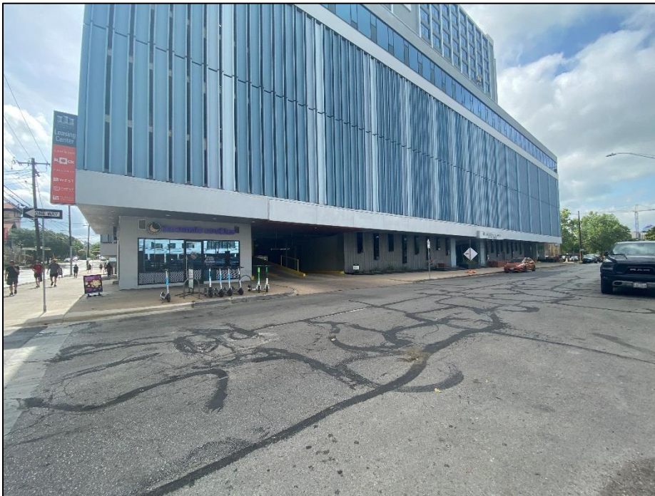
View of the ground level of the façade of Resource 155, looking southeast.
