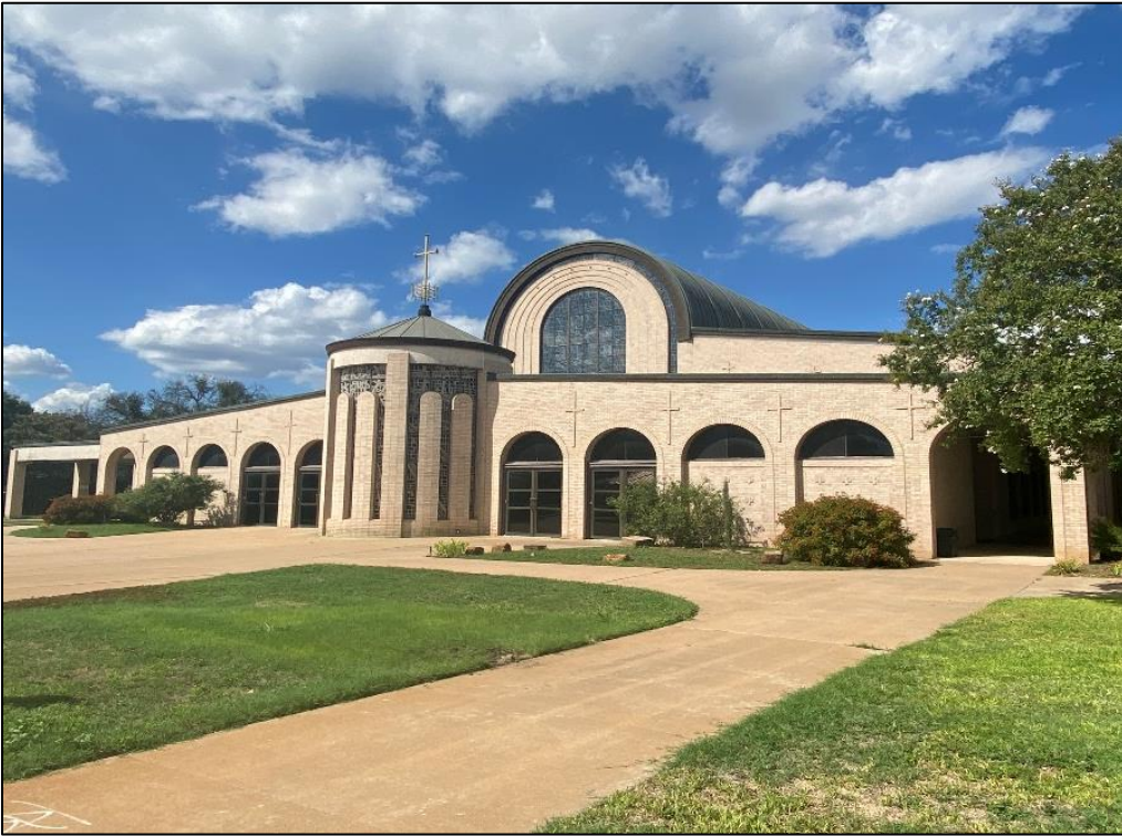
Oblique view of the façade and the east elevation of Resource S196c, looking northwest.
