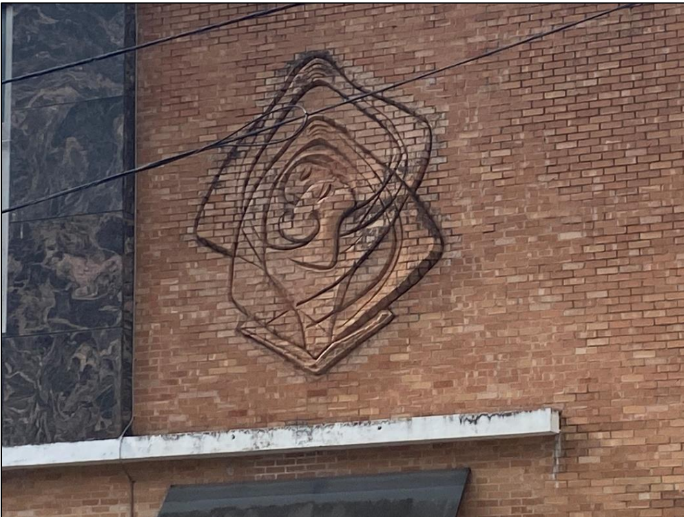
Detail of Umlauf brick intaglio sculpture on Resource S164, looking southeast.
