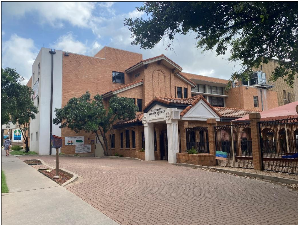
View of the rear (south) elevation of Resource S164 where the non-historic-age addition is attached.
