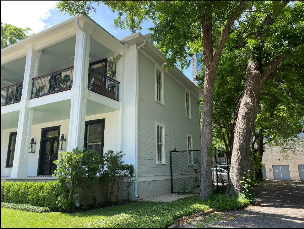
Oblique view of the façade and the west elevation of Resource S172, looking southeast.
