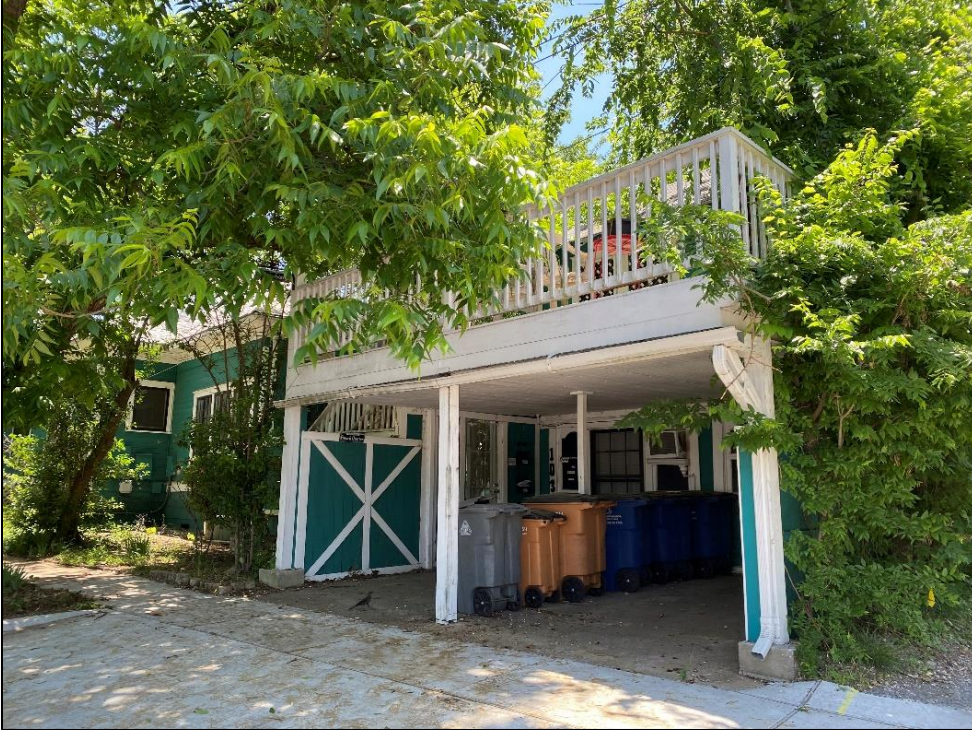
View of the rear addition of Resource S190, looking northeast.
