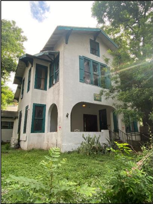
Oblique view of the façade and the west elevation of Resource S159, looking northeast.
