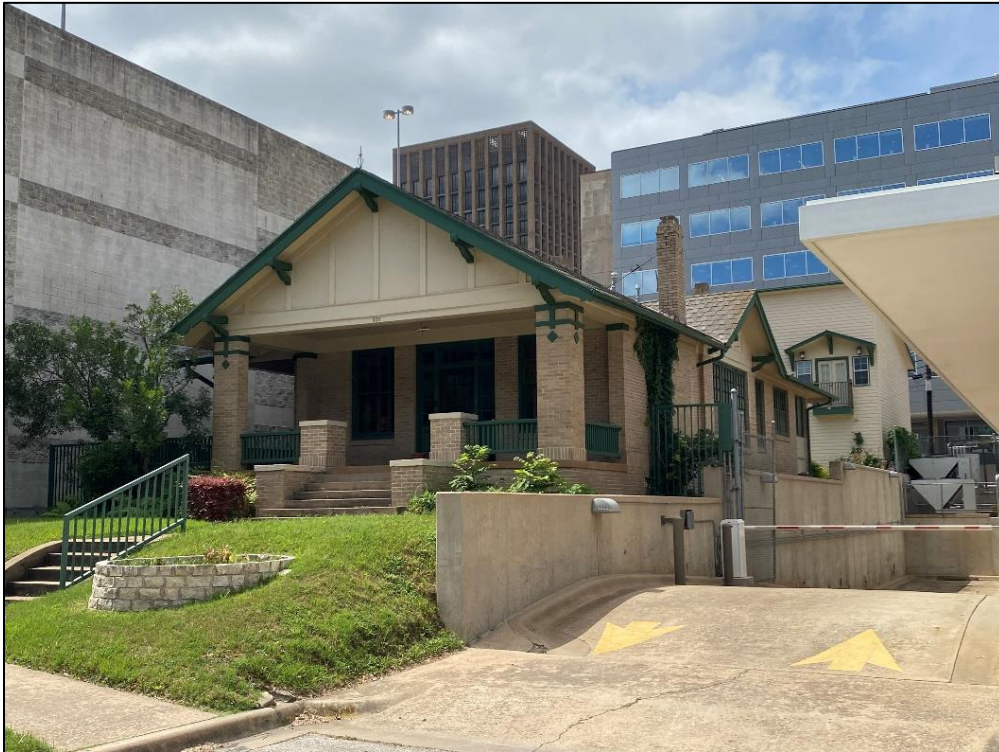
Oblique view of the façade and the west elevation of Resource S181, looking southeast.
