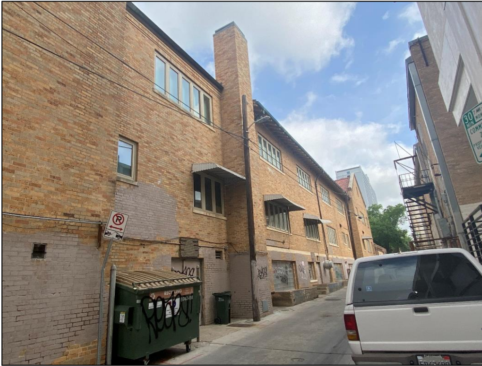
View of the north end of the east elevation of Resource S162, looking northwest.
