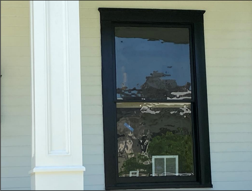
Detail of first floor façade window Resource S172, looking south.
