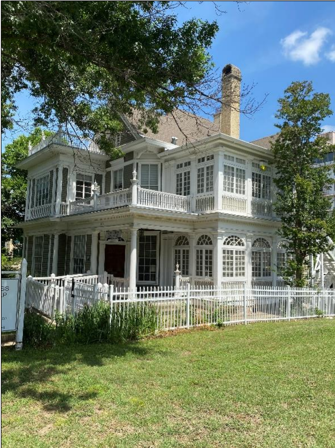
Oblique view of the façade and the east elevation of Resource S182, looking west.
