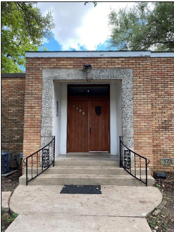
Detail of the façade entry of Resource S196b, looking east.
