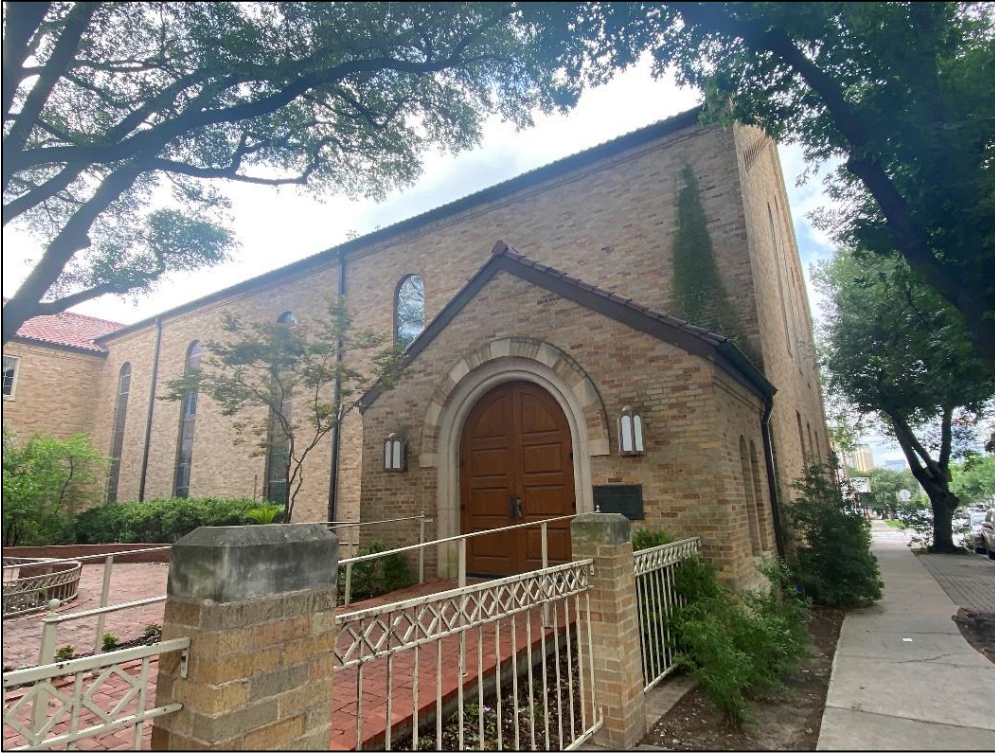
View of the north elevation of the sanctuary, looking southeast.
