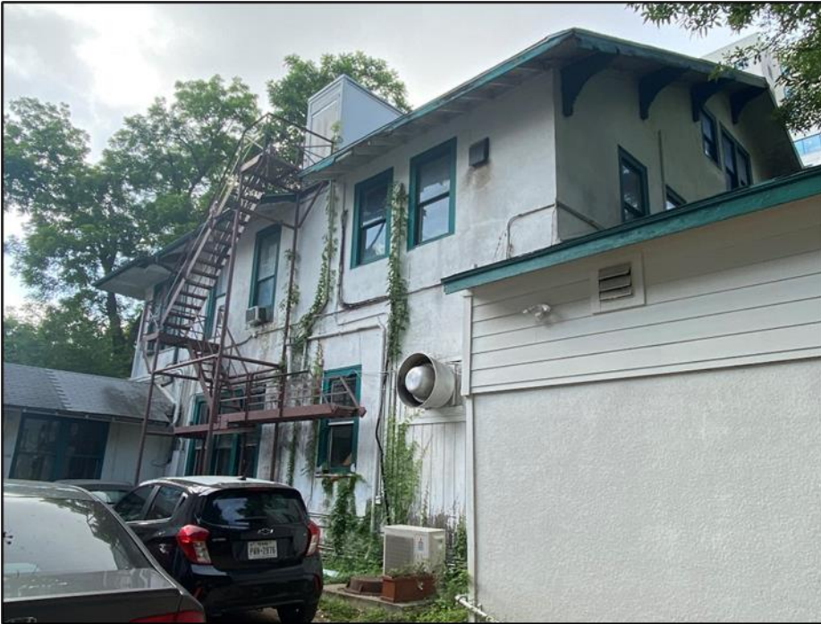
View of the north elevation of Resource S159, looking southeast.
