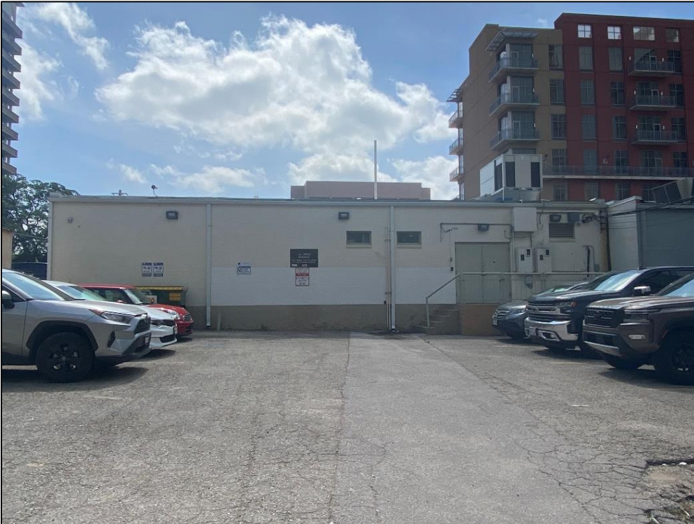
View of rear (west) elevation of Resource S167, looking east.
