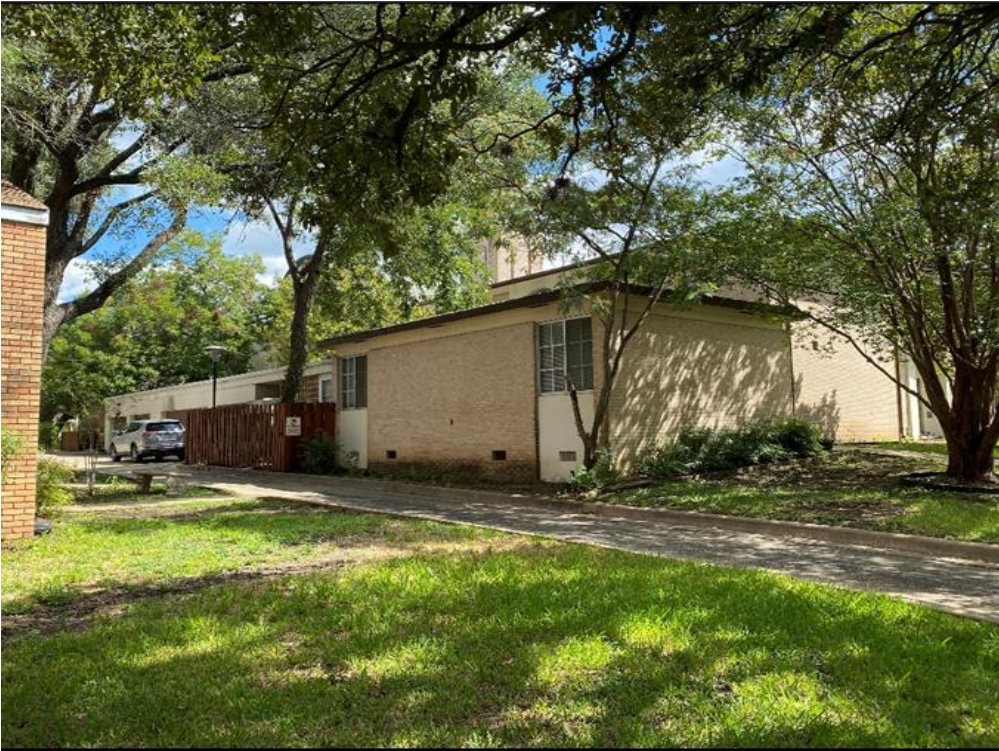
View of the north elevation of Resource S196d, looking southeast.
