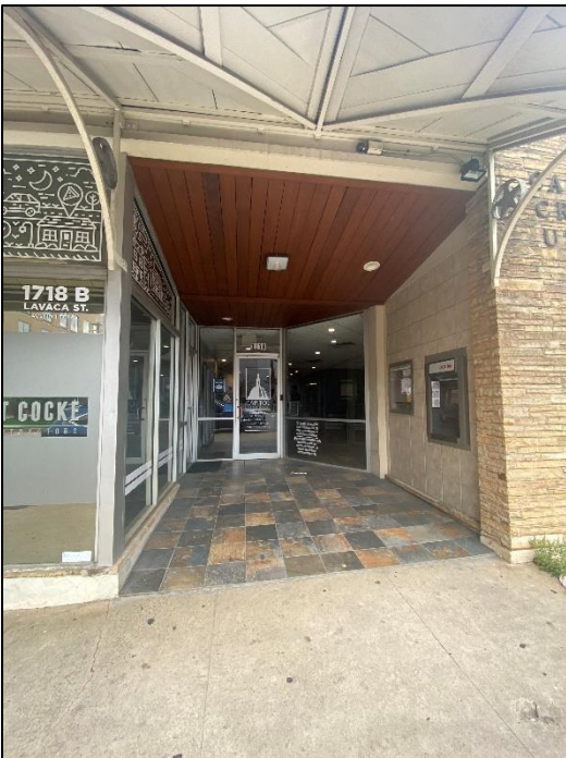
Detail of entry of Resource S166, looking west.
