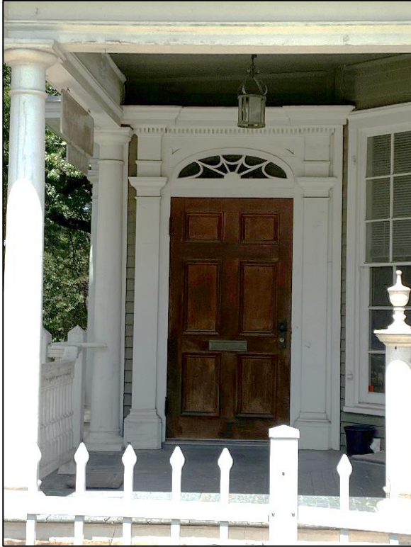
Detail of entry, looking west.
