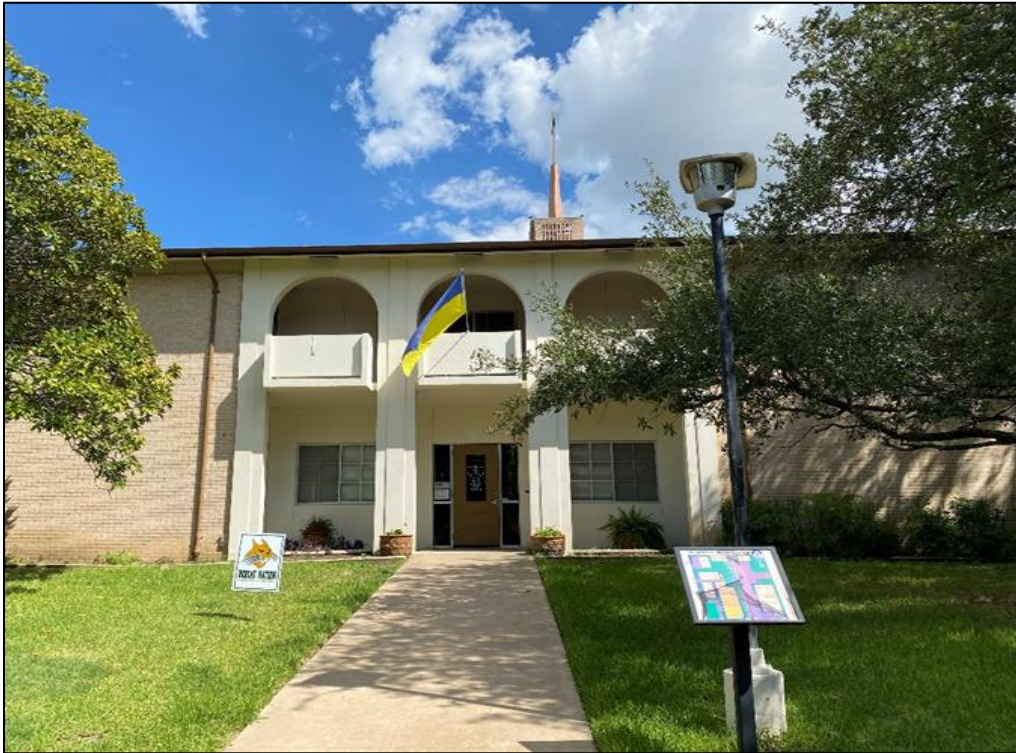
Façade view of Resource S196d, looking east.
