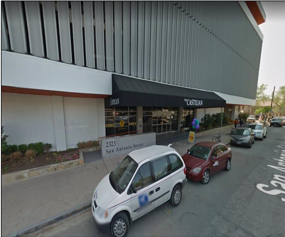
View of the ground level façade prior to ca 2015 remodeling, looking southeast (Google March 2011).
