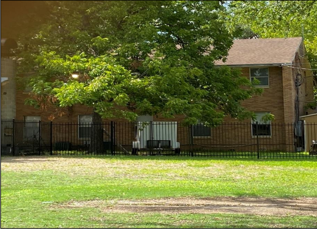
View of the rear elevation of Resource S196b, looking west.
