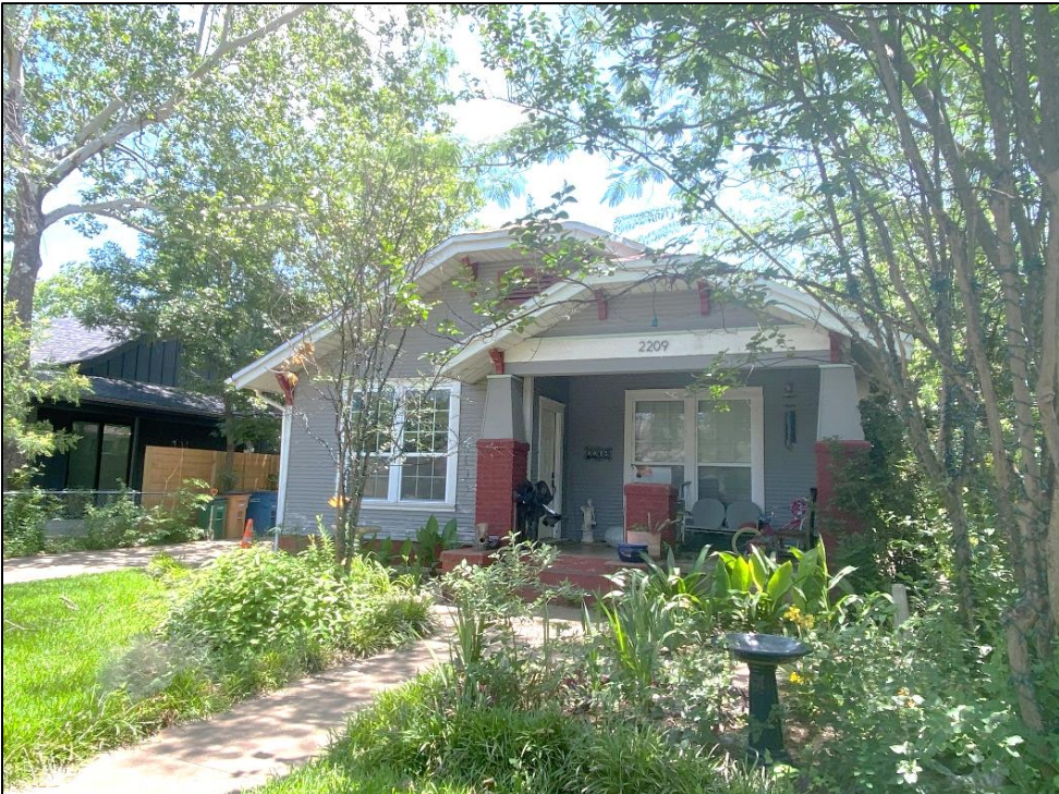
Façade view of Resource S191, looking east.
