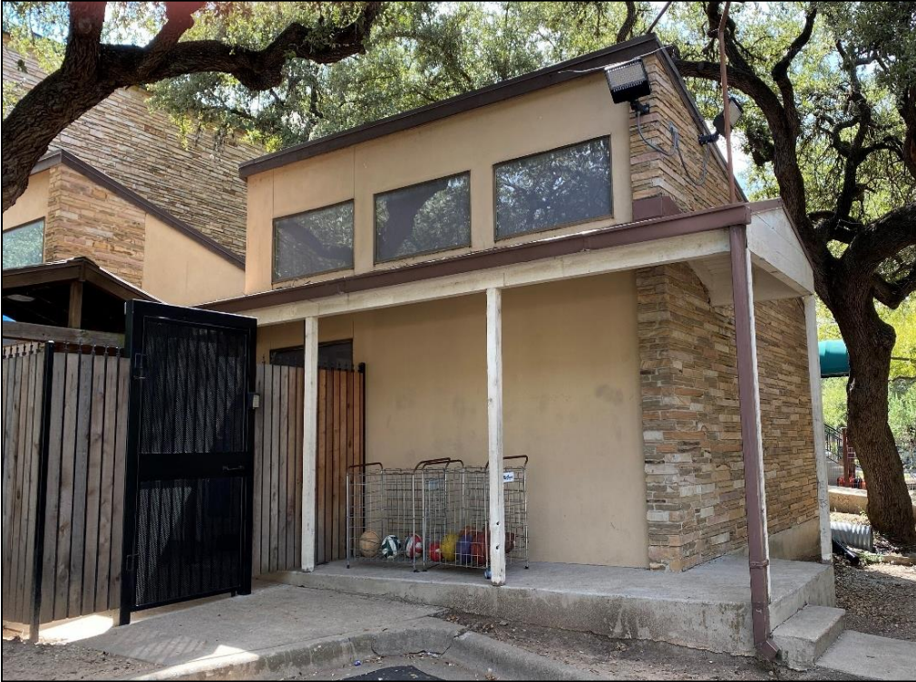
View of the north end of the east elevation of Resource S196a, looking southwest .
