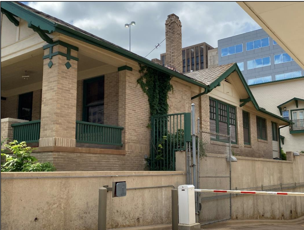
View of the west elevation of Resource S181, looking southeast.
