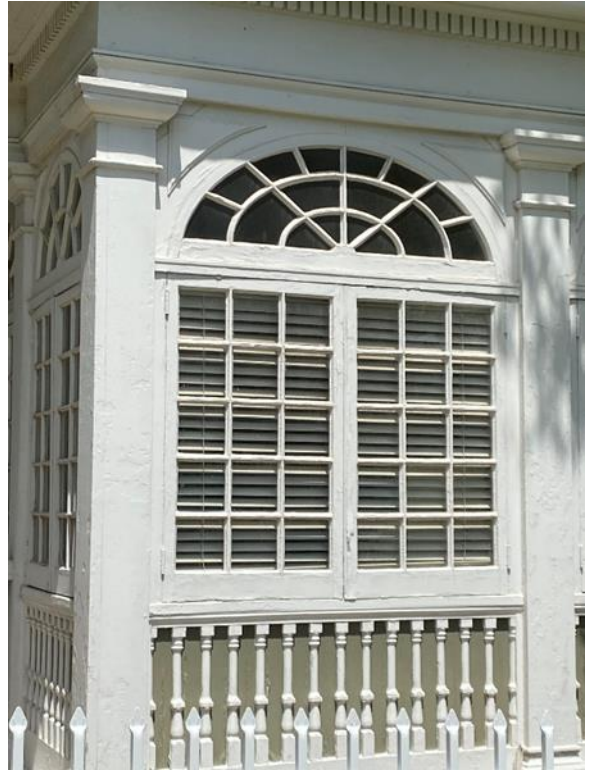
Detail of first-story porch, looking west.
