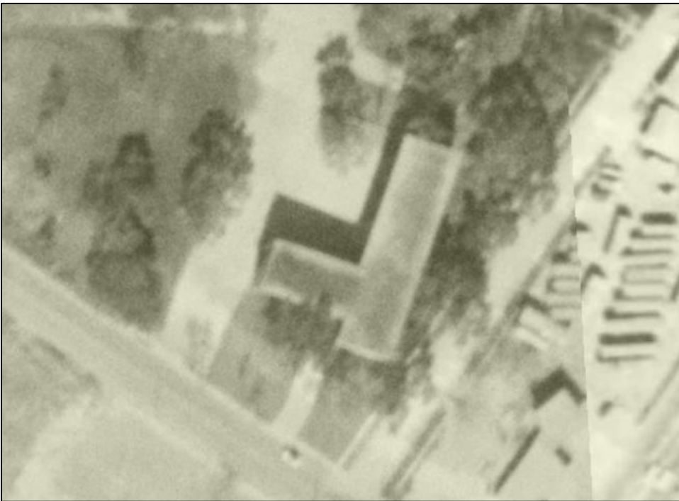
1958 aerial photograph of Resource S196a ( https://maps.austintexas.gov/GIS/PropertyProfile/ ).
