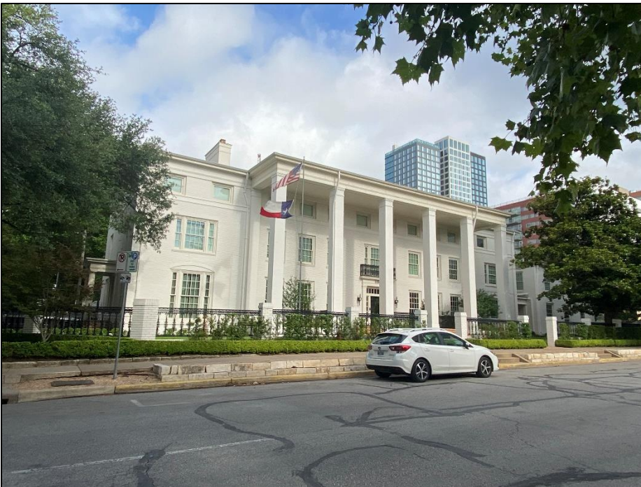
View of the façade of Resource S158, looking northwest.
