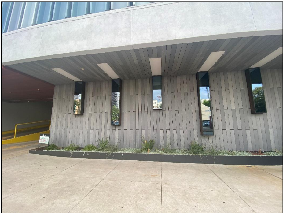
View of the left side of the ground level of the façade of Resource 155, looking east.
