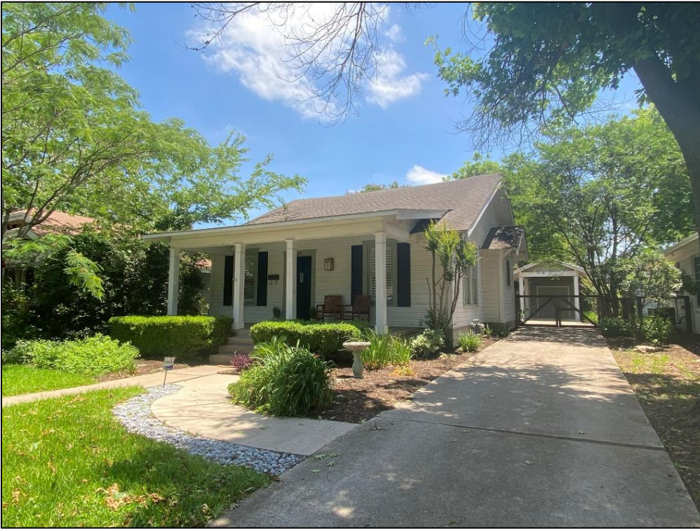
Oblique view of façade and south elevation of Resource S192, looking northeast.
