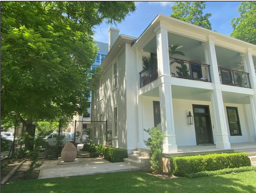
Oblique view of the façade and the east elevation Resource S172, looking southwest.
