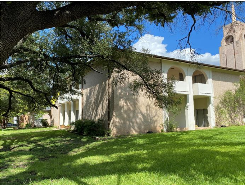
Oblique view of façade and south elevation of Resource S196d, looking northeast.
