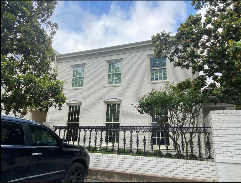
View of the north addition of Resource S158, looking southwest.
