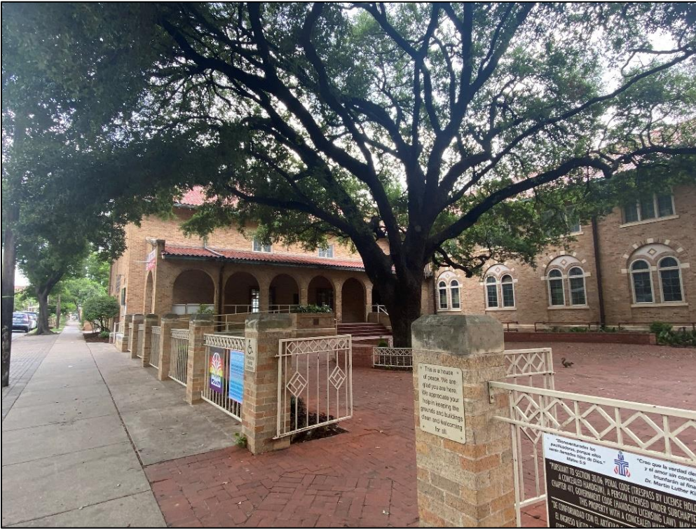
View of the south and west elevations of the original church building, looking northeast.
