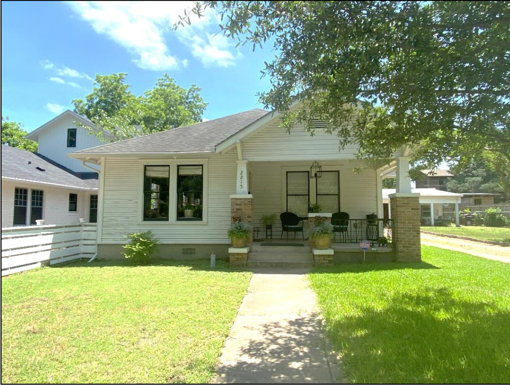
Façade view of Resource S194, looking east.
