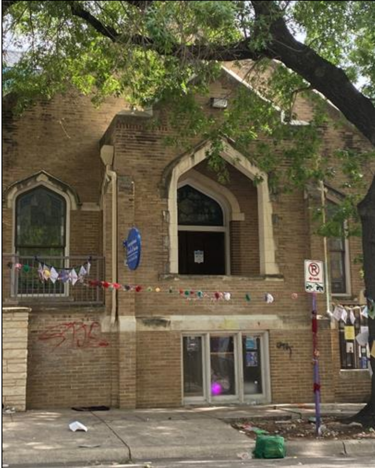
View of the façade of Resource S160, looking north.
