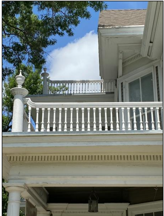
Detail of the façade roof balcony.
