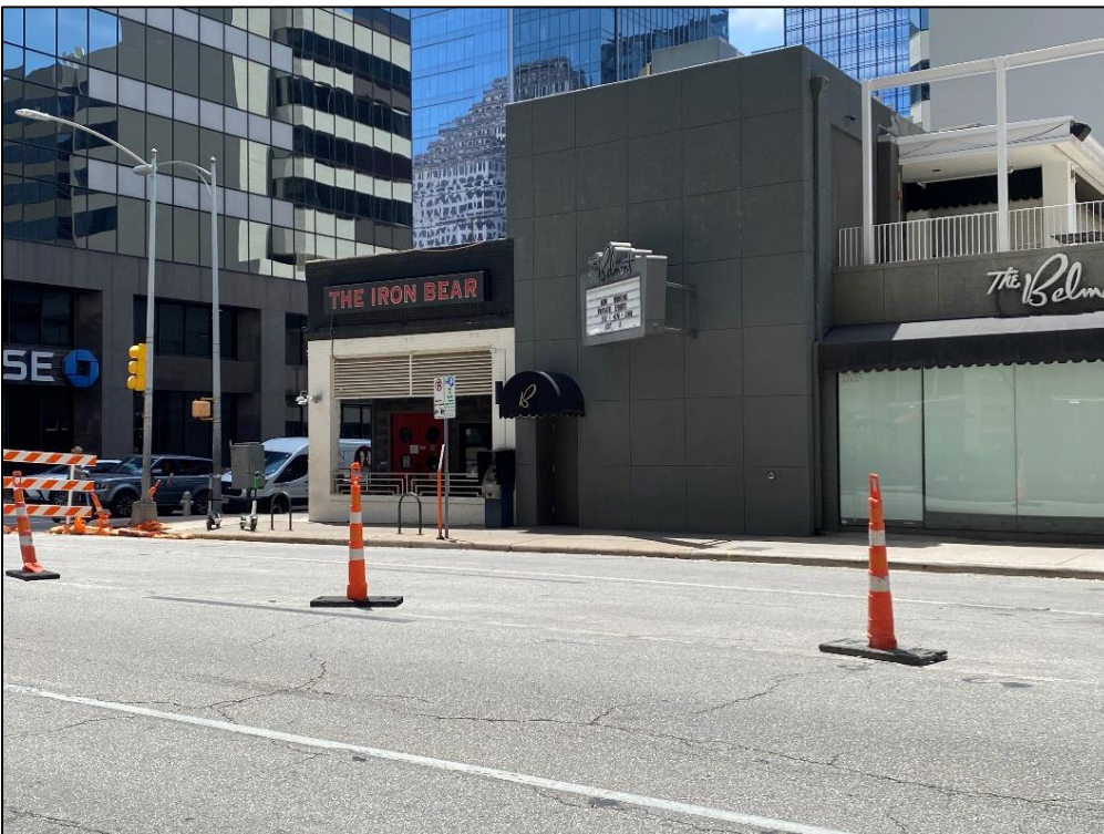
View of east side of façade, looking southeast (IMG_1730).
