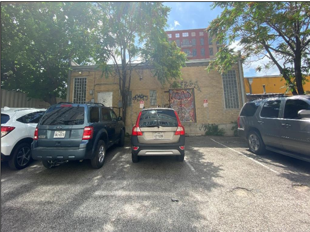
View of the rear (west) elevation of Resource S168, looking east.
