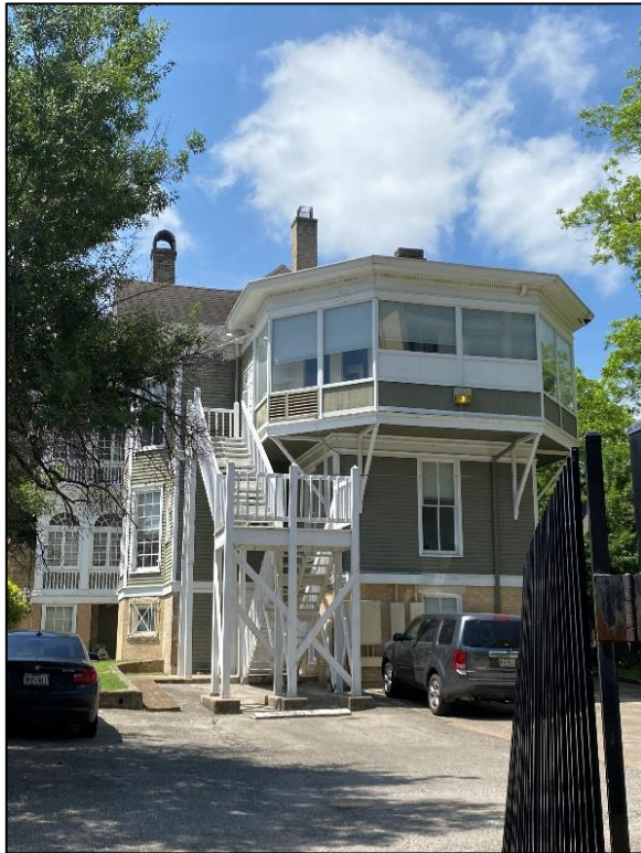
View of the rear elevation, looking south.
