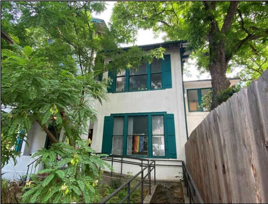
View of the east side of the façade of Resource 159, looking north.
