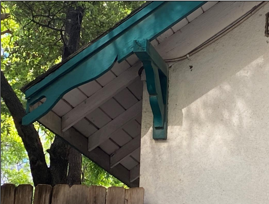
Detail of the bargeboard of the original entry, looking east.
