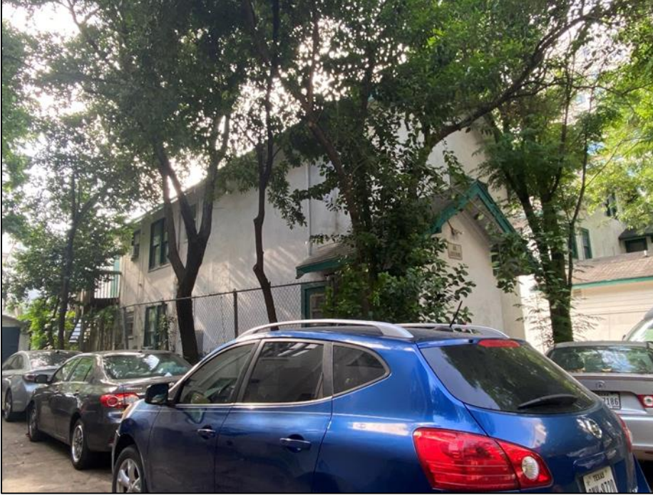
View of the north elevation of Resource S157, looking southeast.
