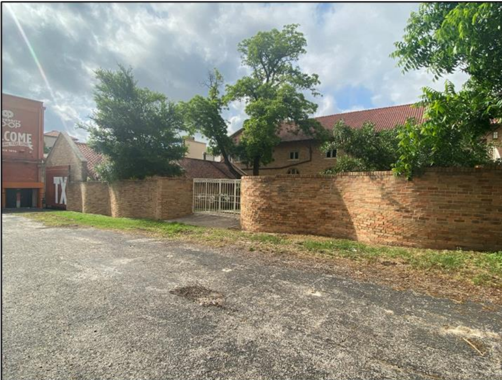
View of the garden wall and the north elevation of Resource S162, looking southeast.
