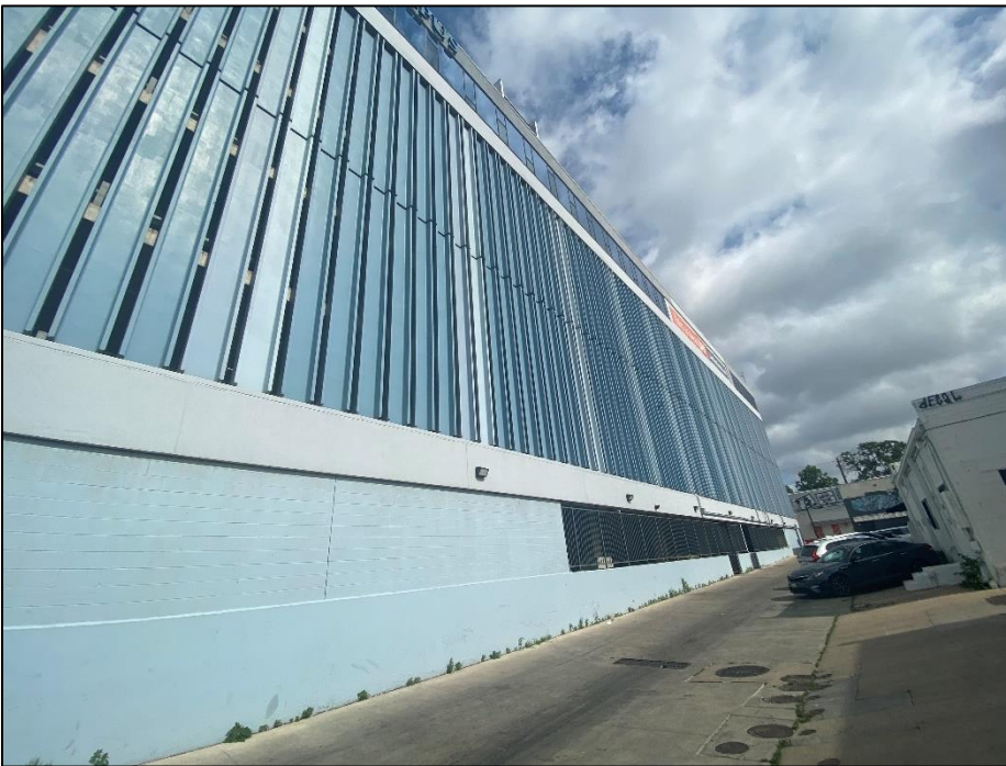
View of the first-story, rear (east) elevation, looking northwest (IMG_1551).
