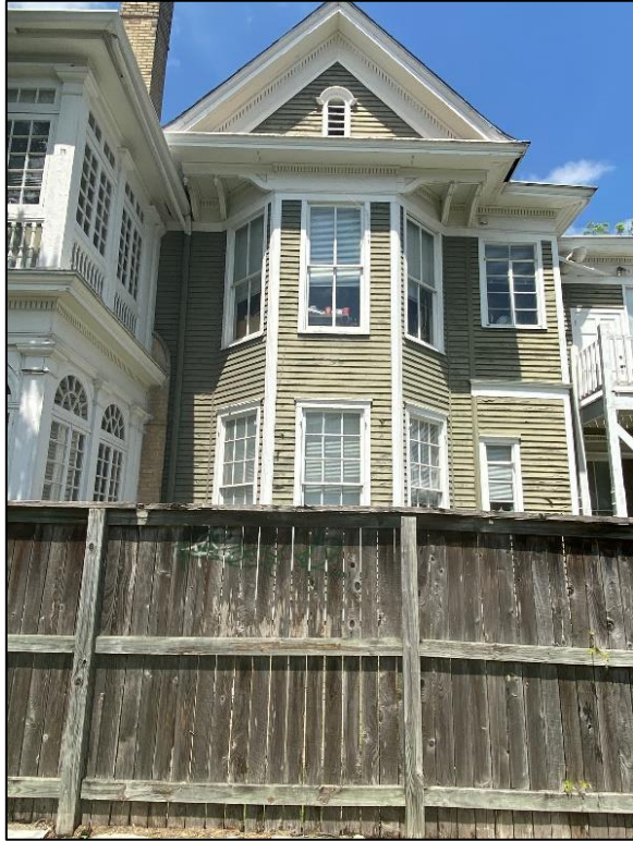
View of the east elevation, looking west.
