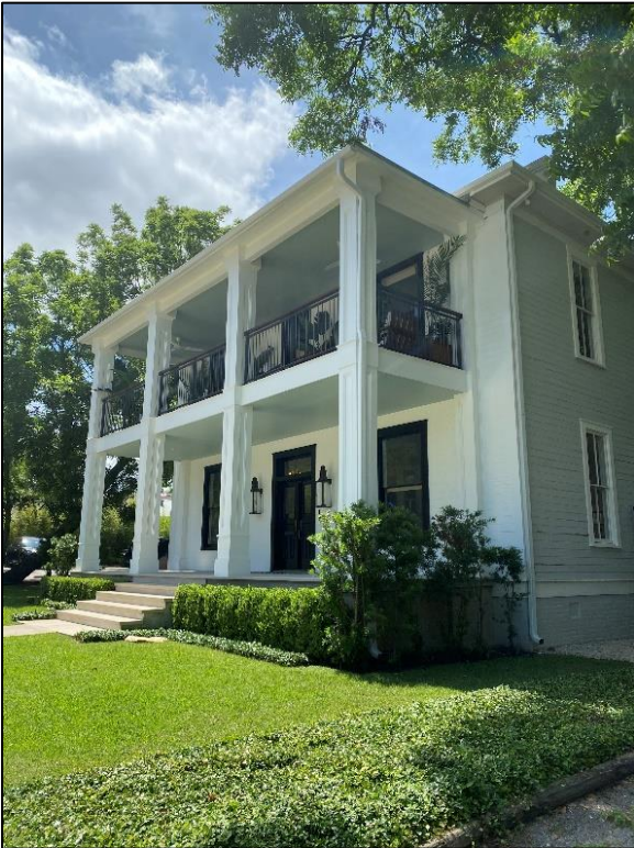
Oblique view of the façade of Resource S172, looking southeast.
