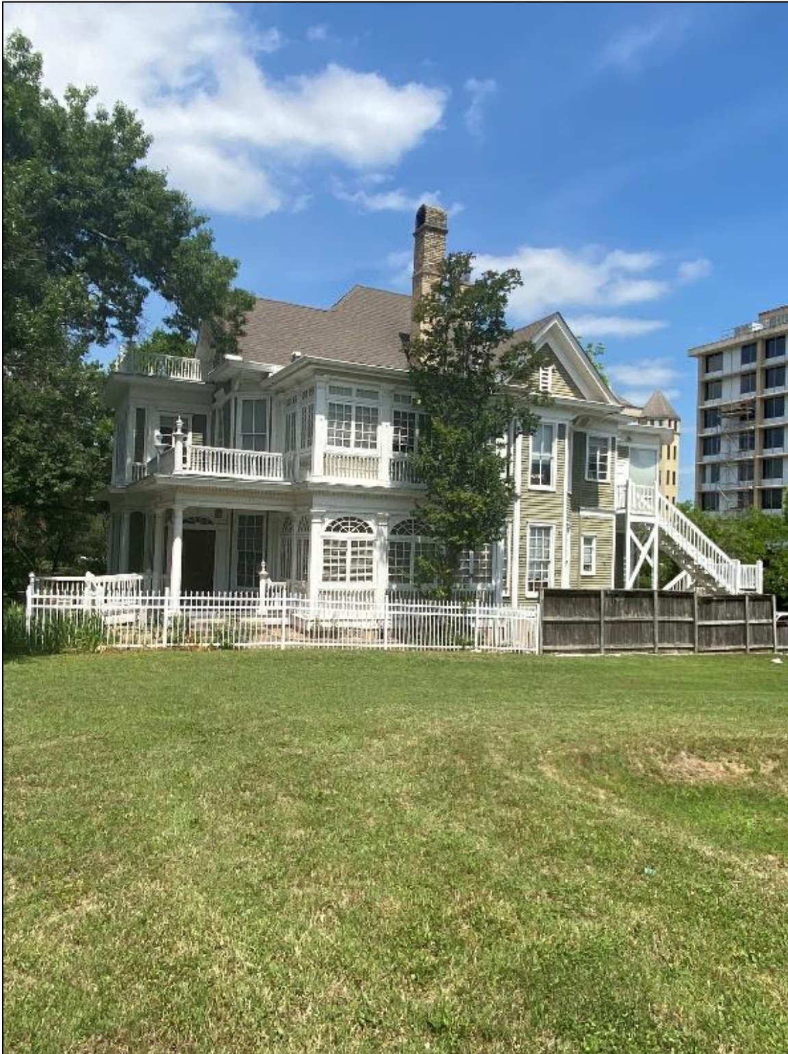
View of the east elevation of Resource S182, looking west.
