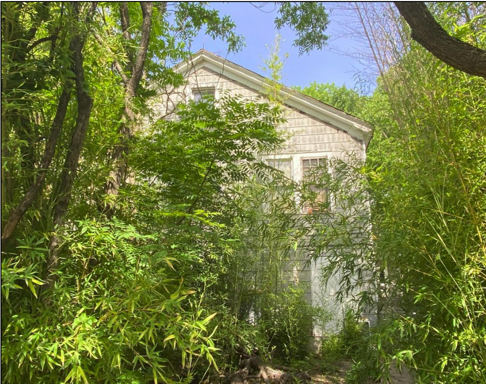
View of the southeast elevation of Resource S118, looking northwest.
