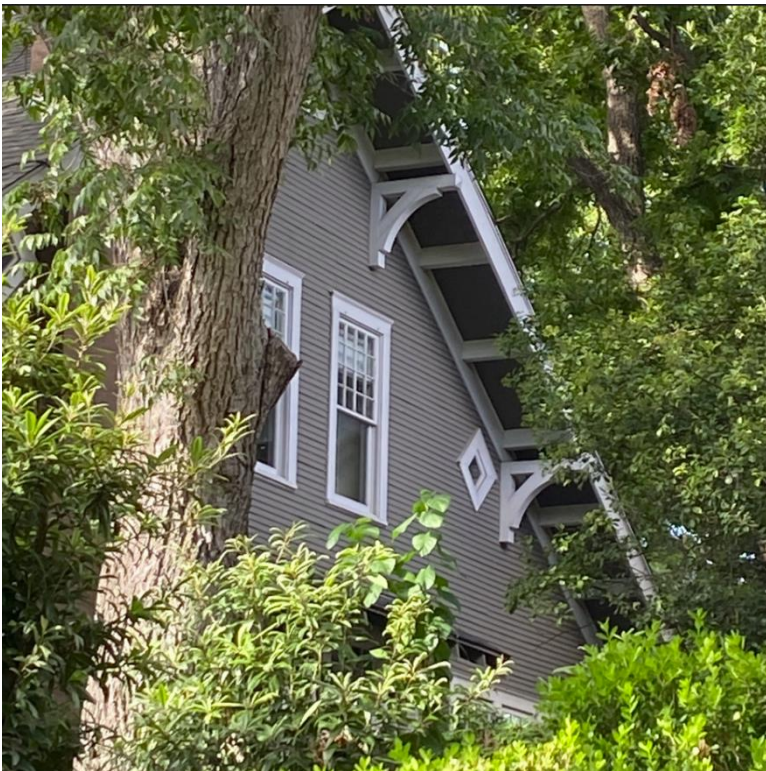
View of the north elevation of Resource S110, looking southwest.
