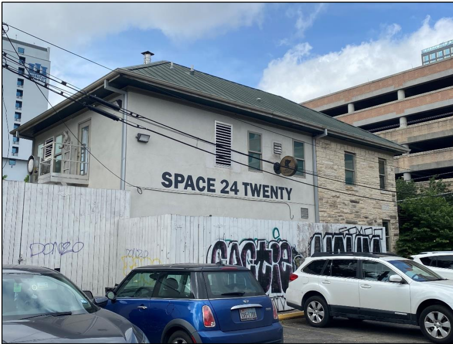
Oblique view of the rear (east) elevation and the north elevation of Resource S150, looking southwest.
