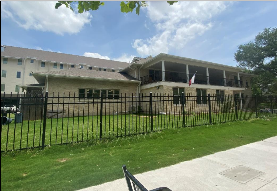
Façade view of Resource S142, looking southeast.
