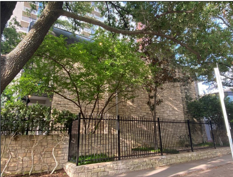
View of the north elevation of Resource S149, looking southwest.
