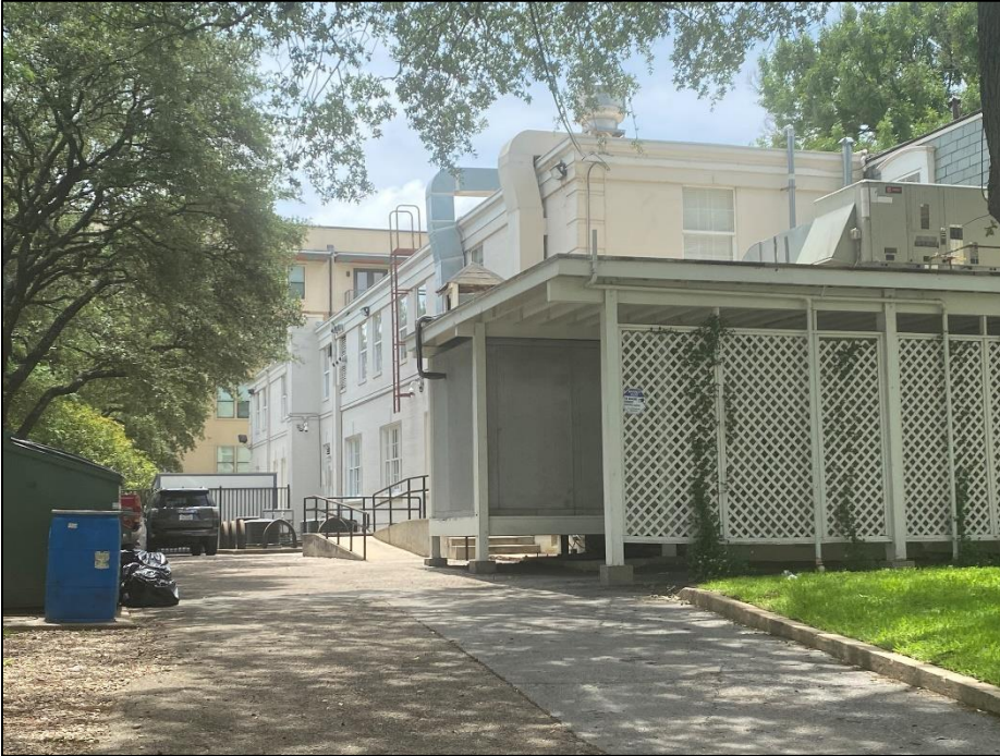
View of the east elevation, looking south (IMG_1316).
