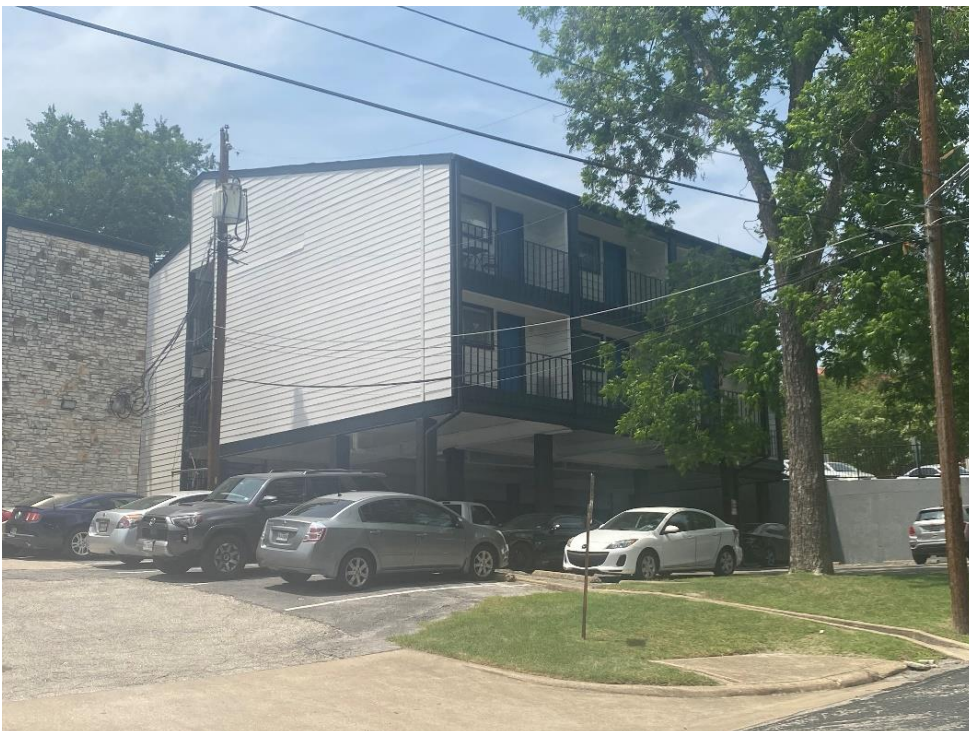
Oblique view of the rear (south) and east elevations of Resource S128, looking northwest.
