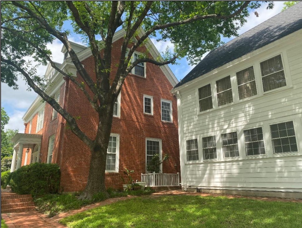
Oblique view of the façade and north elevation of Resource S108a and the east elevation of Resource S108b, looking west-southwest.
