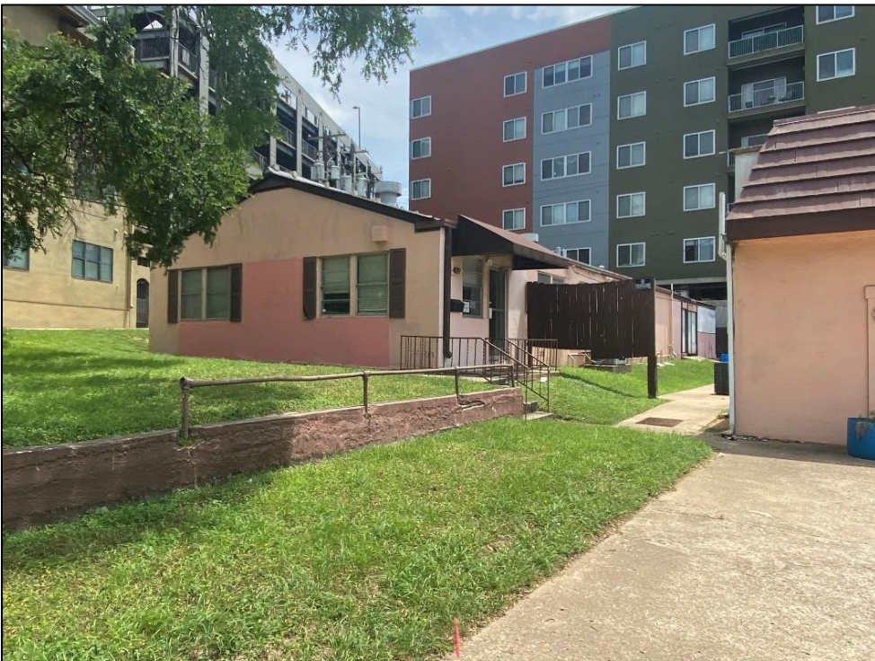
Oblique view of the northeast elevation and façade of Resources S127b, looking south-southeast.
