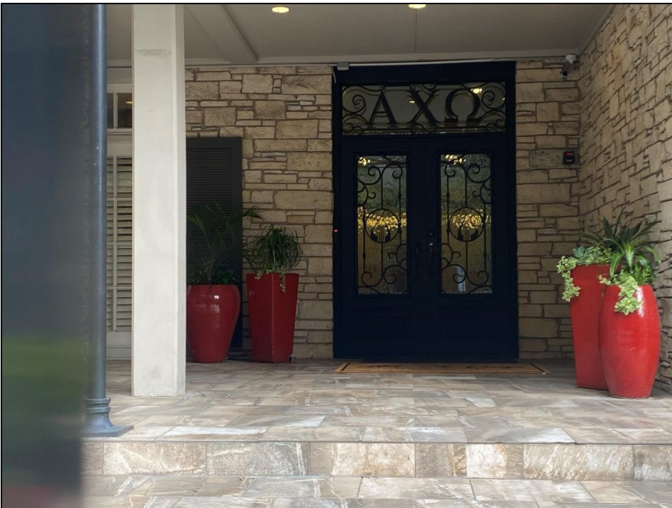
Detail of the primary entrance, Resource S149, looking west.
