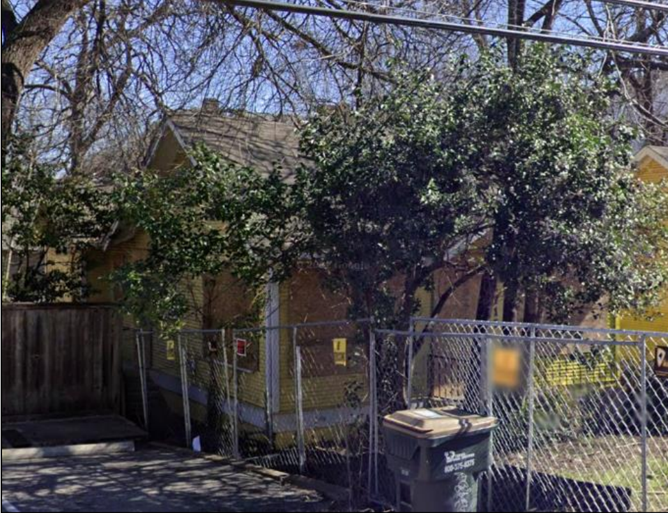
Oblique view of the north elevation and façade of Resource S137a, looking southeast (Google Image Capture 02/2022).
