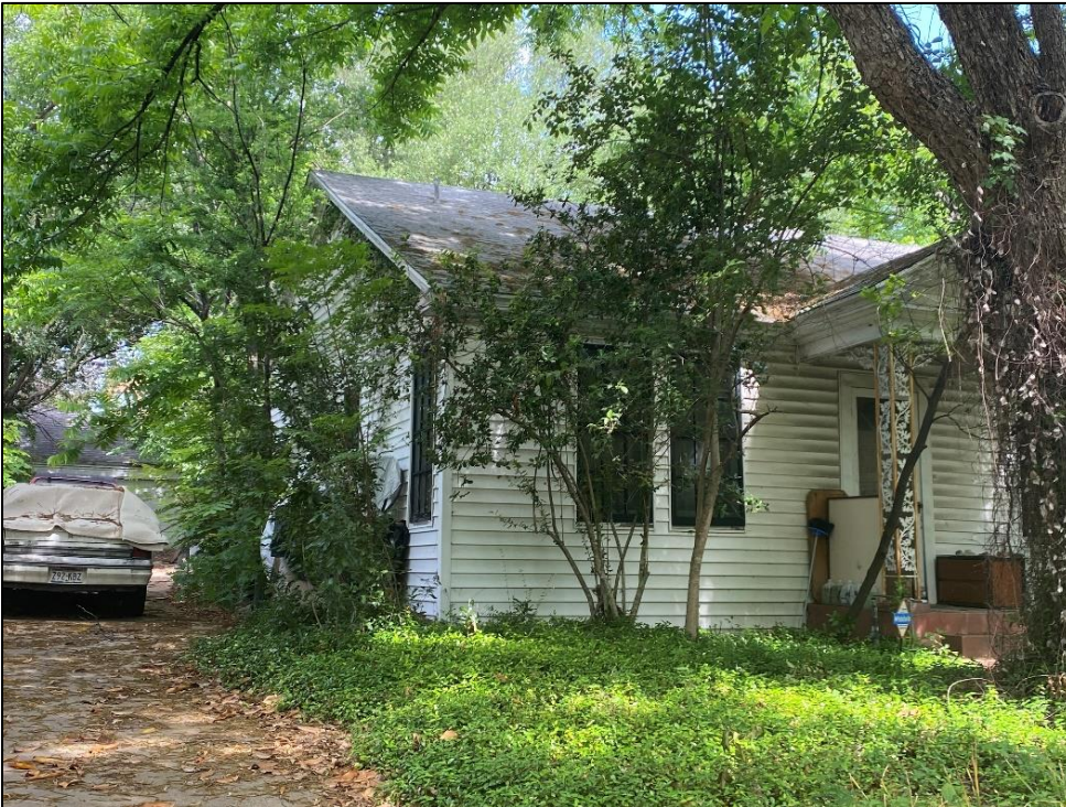
Oblique view of the southwest elevation and the façade of Resource S115a, looking north-northwest.
