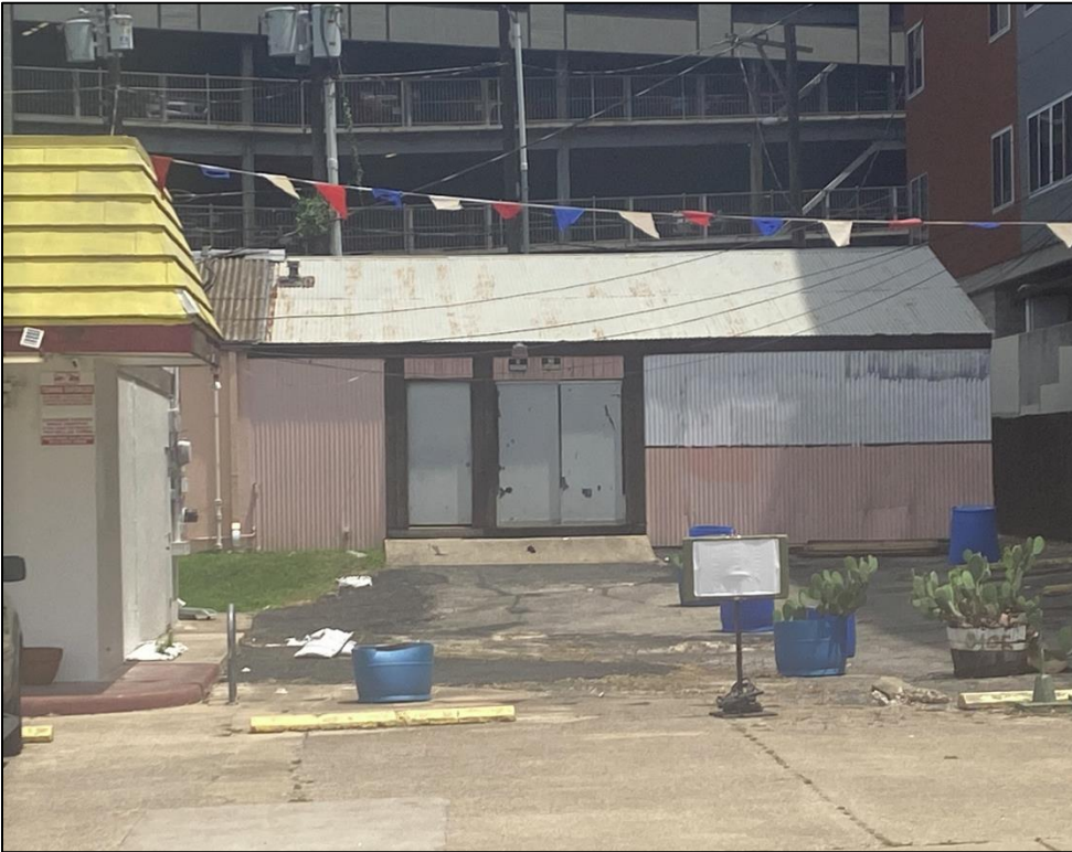
Façade view of the southwestern addition to Resource S127b, looking southeast.
