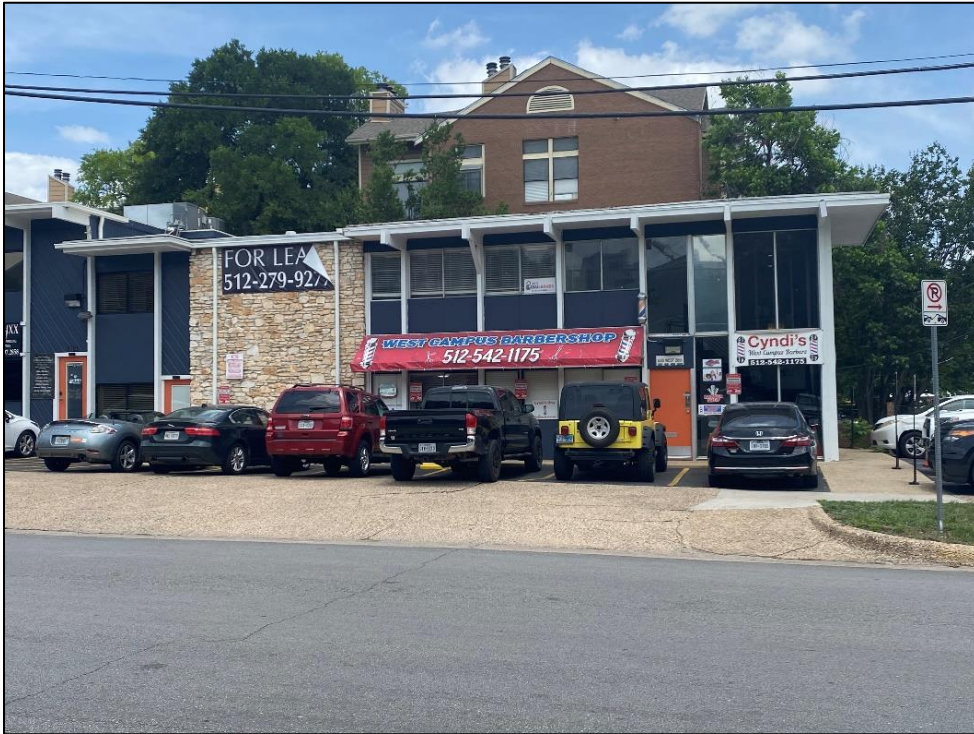
View of the east end of the façade of Resource S133, looking north.
