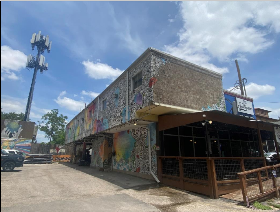
View of the façade and the west elevation of Resource S145, looking northwest.
