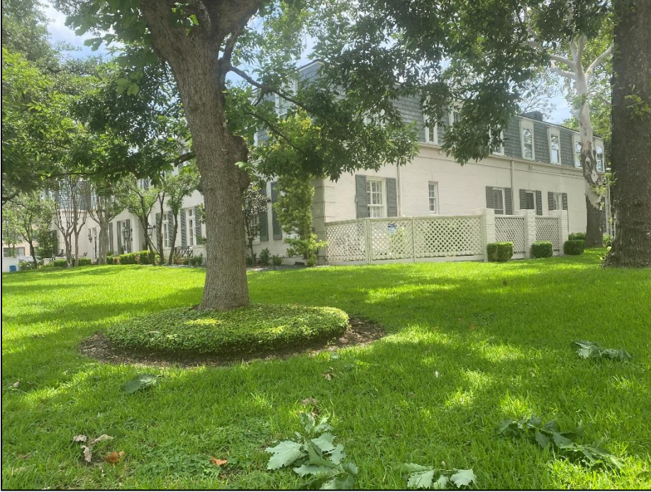
Oblique view of the façade and the west elevation, looking southeast (IMG_1313).
