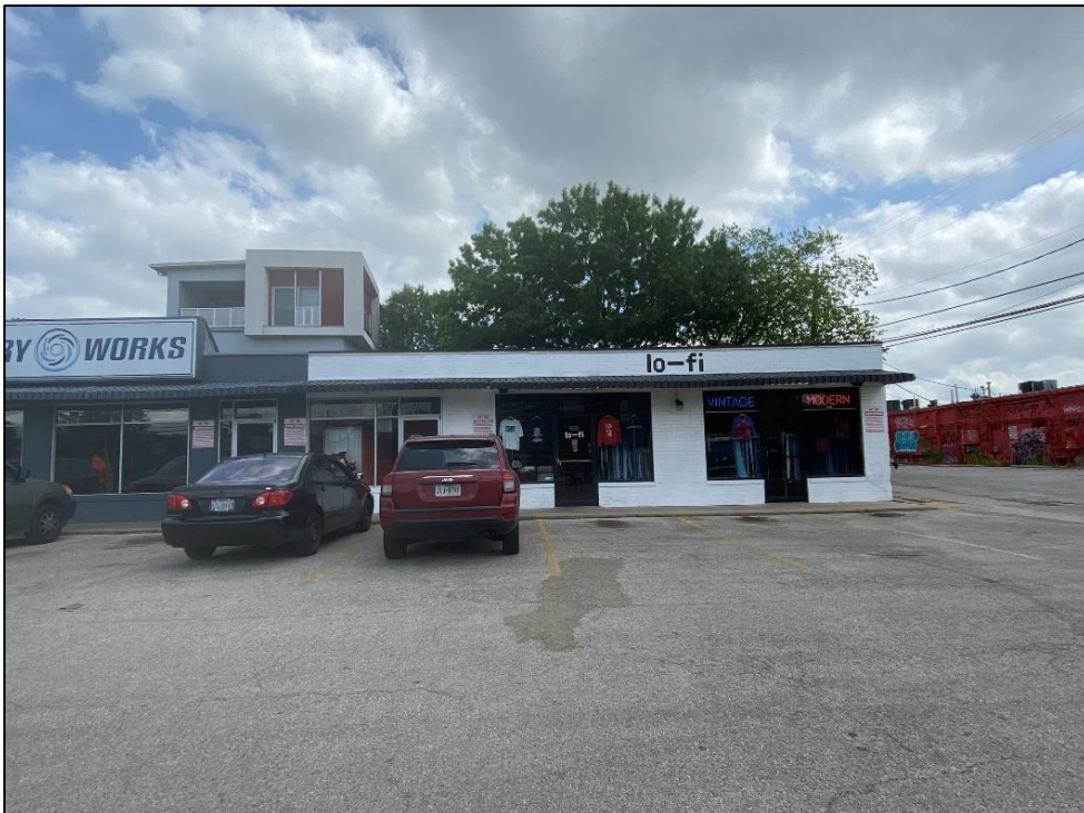
View of the southeast end of the façade of Resource S120, looking north-northeast.
