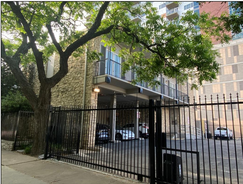
Oblique view of the north and rear (west) elevations of Resource S149, looking southeast.
