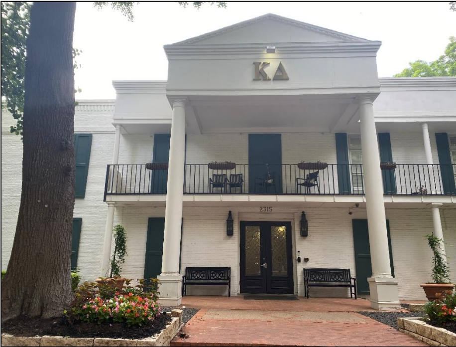
Detail of the façade entry of Resource S154, looking east.
