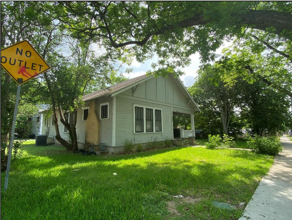
Oblique view of the northwest elevation and façade of Resource S119a, looking northeast.
