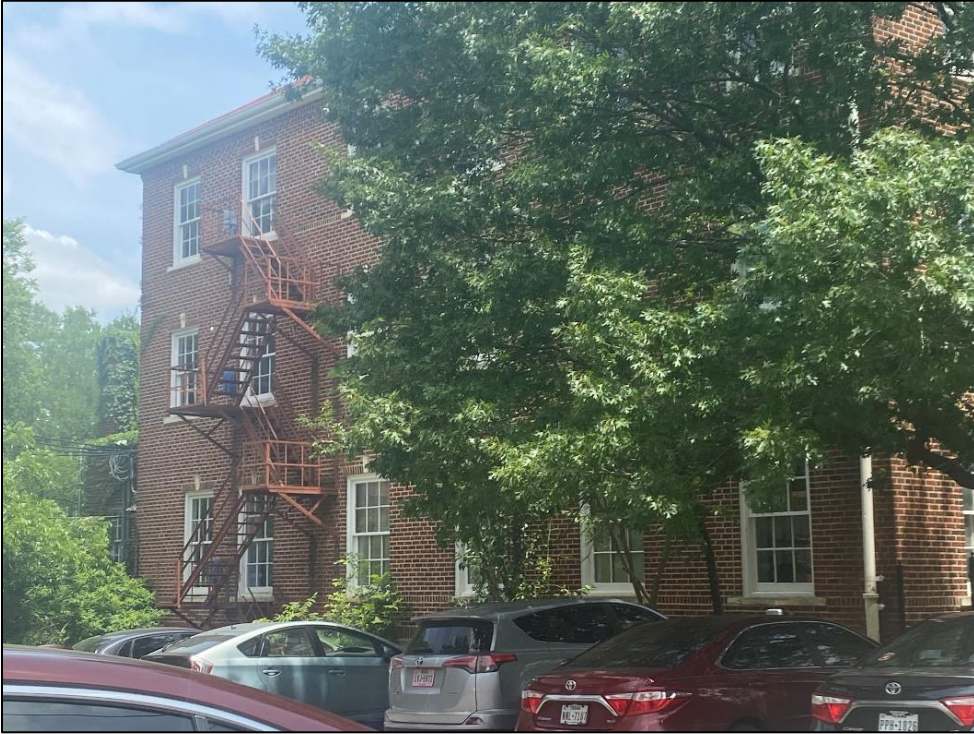
View of the northwest elevation of Resource S126, looking north-northeast.
