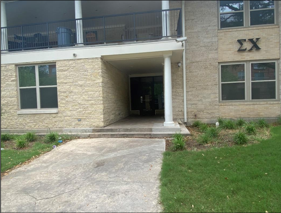
Detail of primary entrance to Resource S142, looking east.
