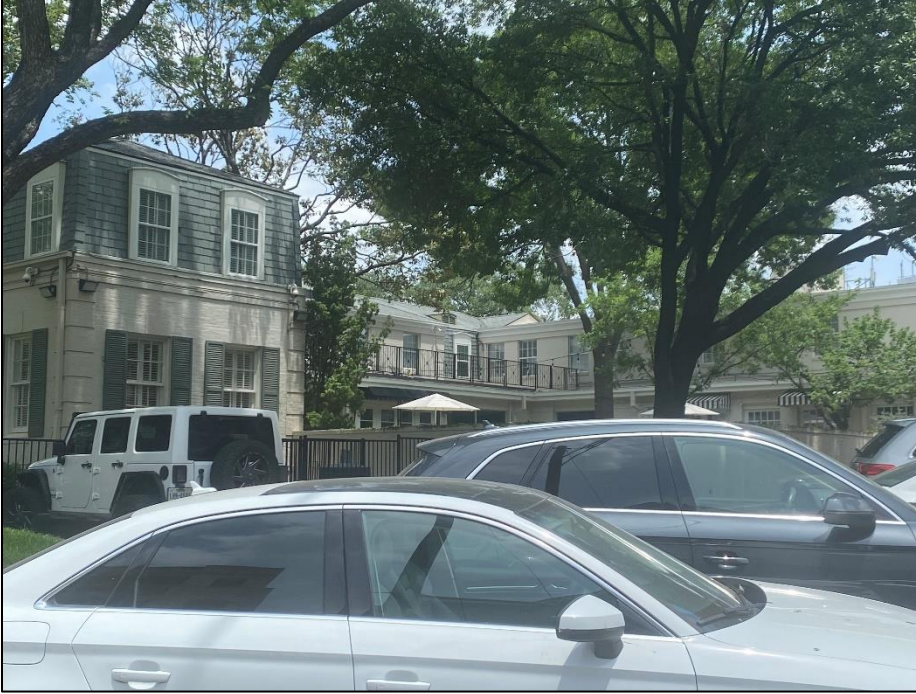
View of the south elevation, looking northeast (IMG_1311).
