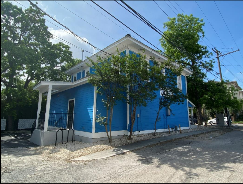
Oblique view of the rear (northeast) and northwest elevations of Resource S117, looking southeast.
