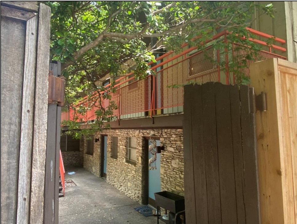
View of the north elevation of the east/west wing of Resource S140, looking southeast.
