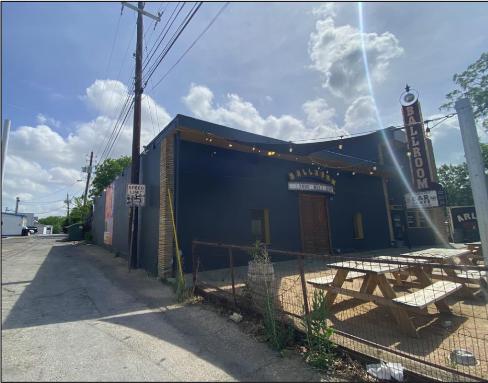
Oblique view of the northwest elevation and façade of Resource S125, looking north-northeast.
