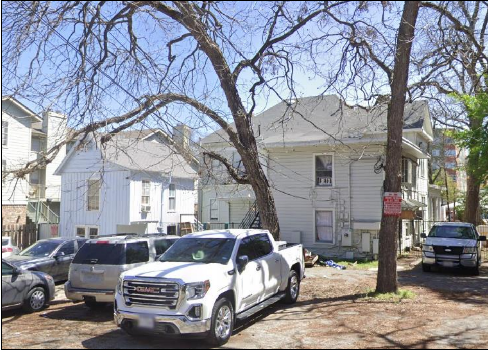
Oblique view of the rear (west) and south elevations of Resources 129a-b, looking east (Google Image Capture 03/2022)
