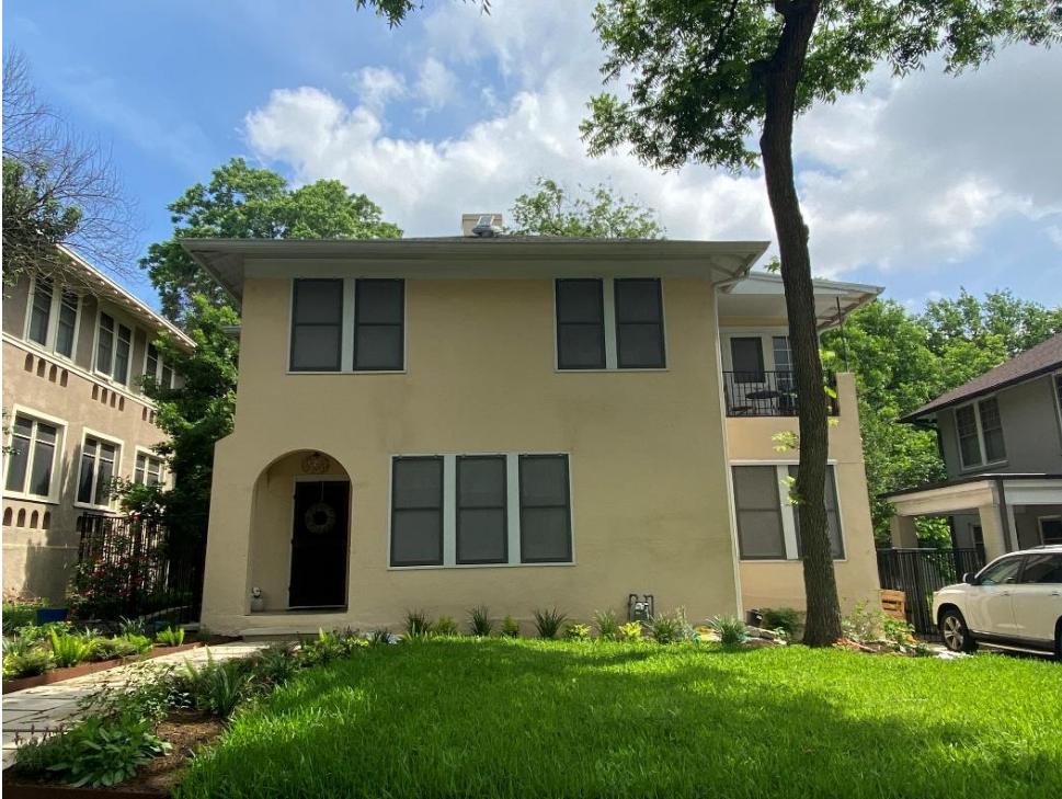
Façade view of Resource S107, looking northeast.
