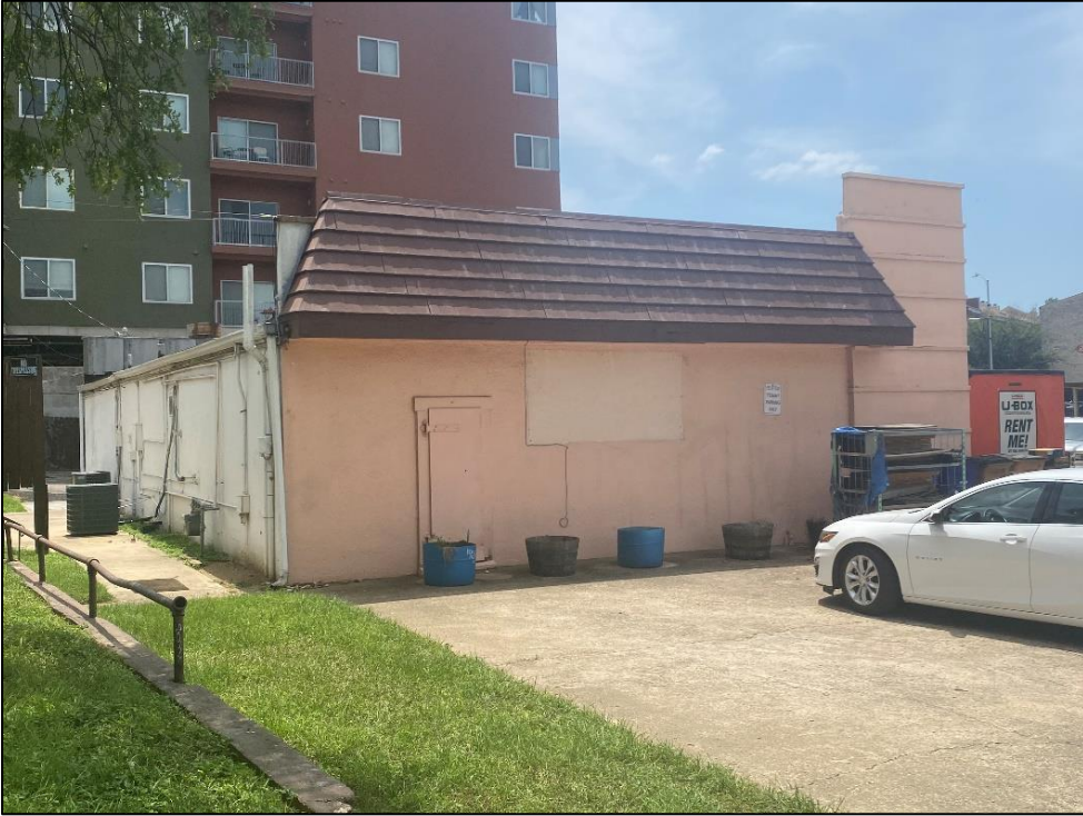
Oblique view of the rear (southeast) and northeast elevations of Resource S127a, looking southwest.
