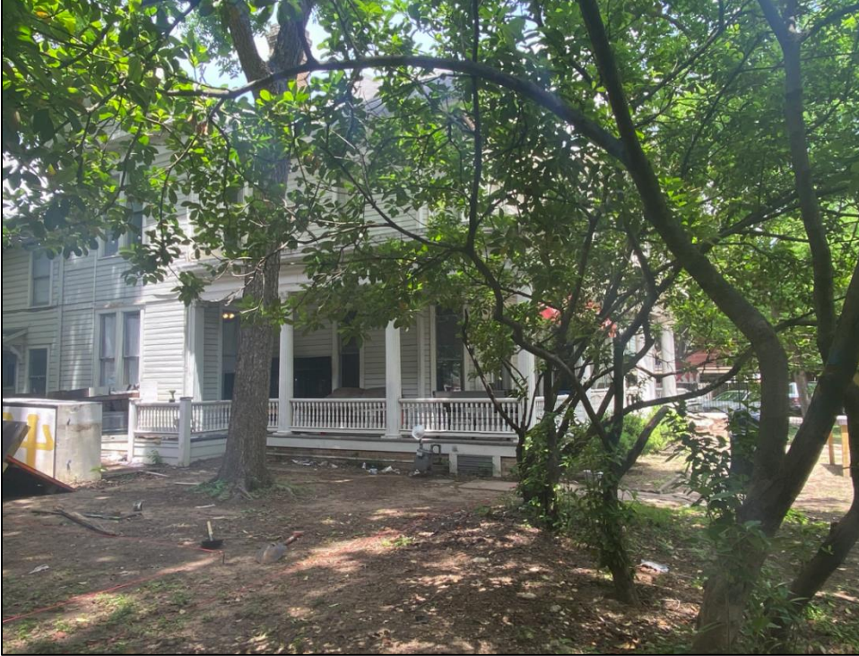
Oblique view of the south elevation and façade of Resource S129a, looking northwest.
