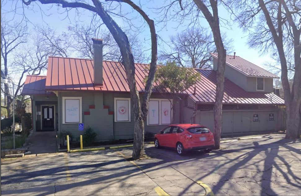
View of the northwest elevation of Resource S121, looking southeast (Google Image Capture 02/2022).
