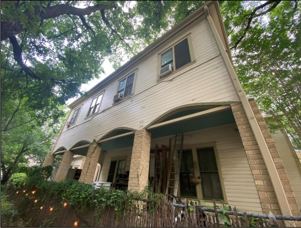
View of the south elevation of Resource S148, looking north.
