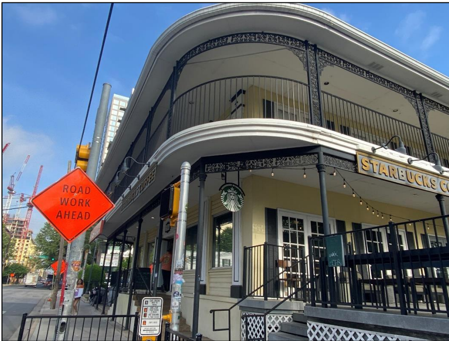
View of the southeast corner, looking northwest.
