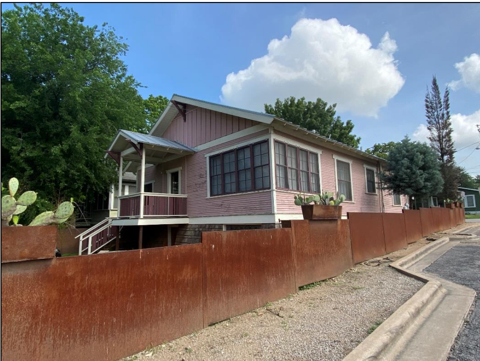
Oblique view of the rear (southwest) and southeast elevations of Resource S109, looking north-northwest.
