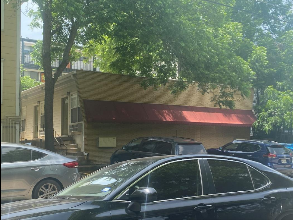
Oblique view of the south elevation and façade of Resource S135, looking northwest.
