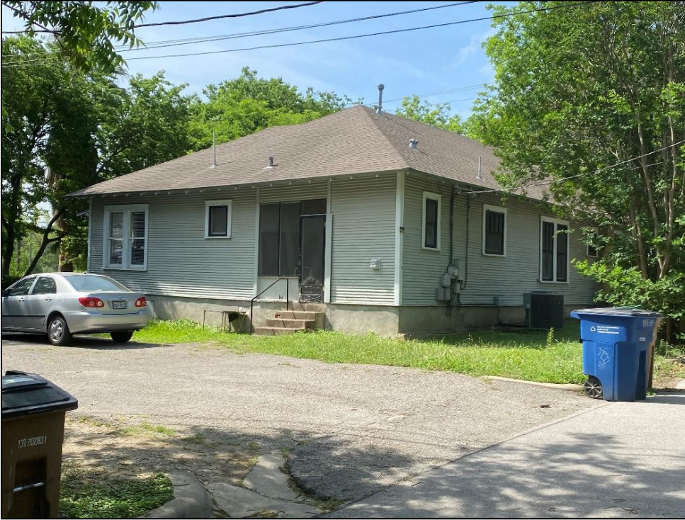
Oblique view of the rear (northeast) and northwest elevations of Resource S119, looking south.
