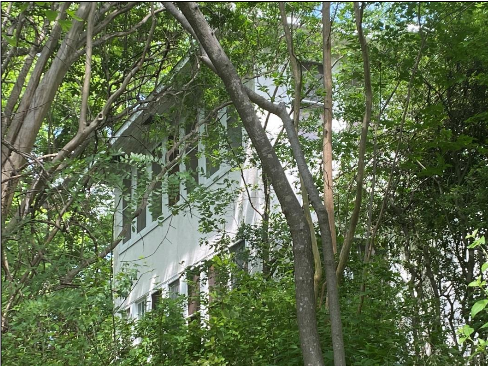
View of the south elevation of Resource S111, looking northwest.
