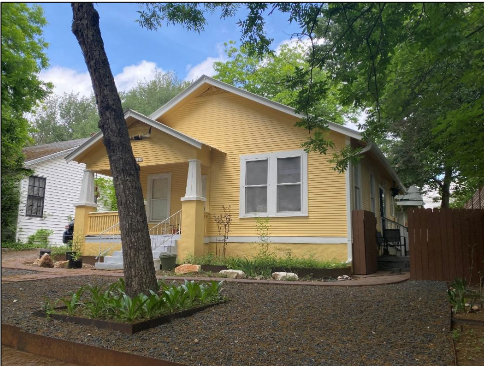
Oblique view of the façade and northeast elevation of Resource S114a, looking west.
