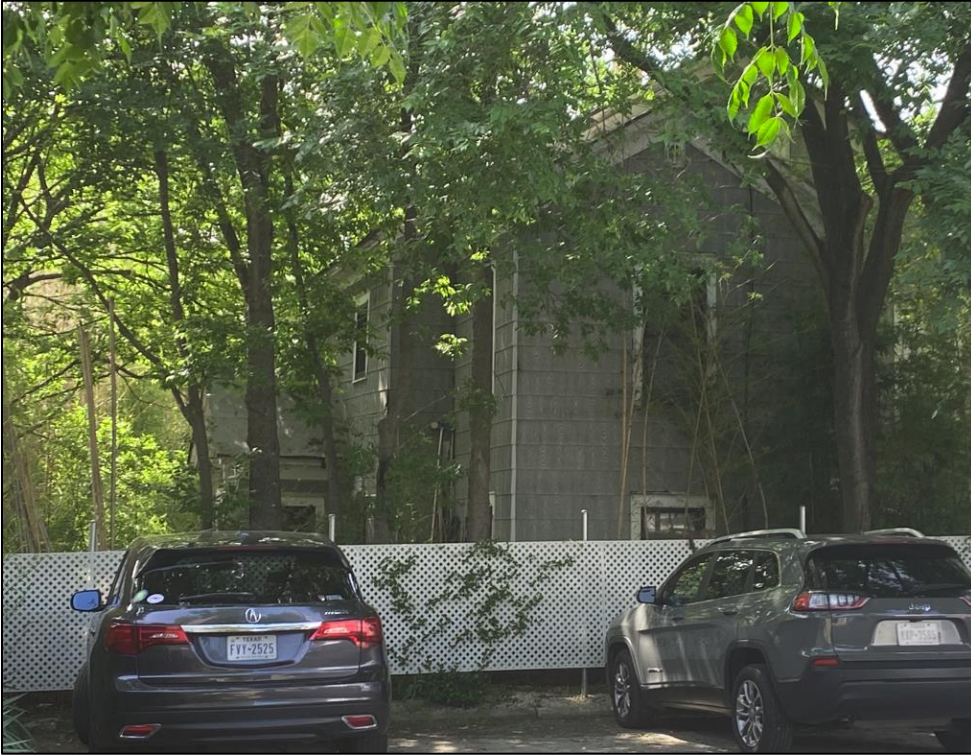
Oblique view of the rear (northeast) and northwest elevations of Resource S118, looking southeast.
