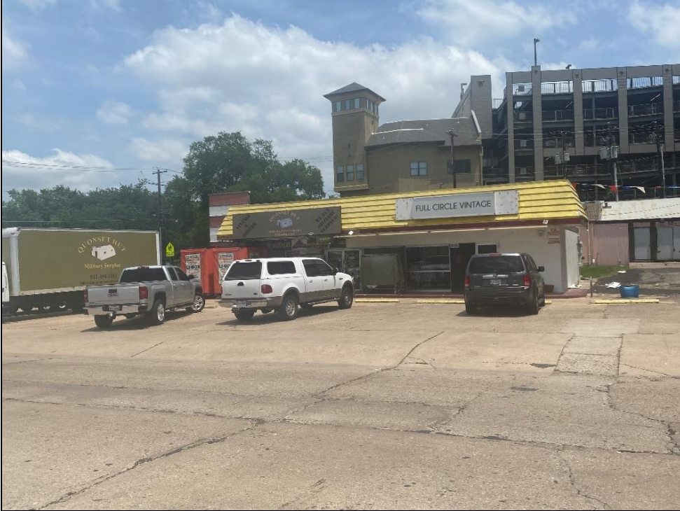
View of façade and southwest elevation of Resource S127a, looking southeast.
