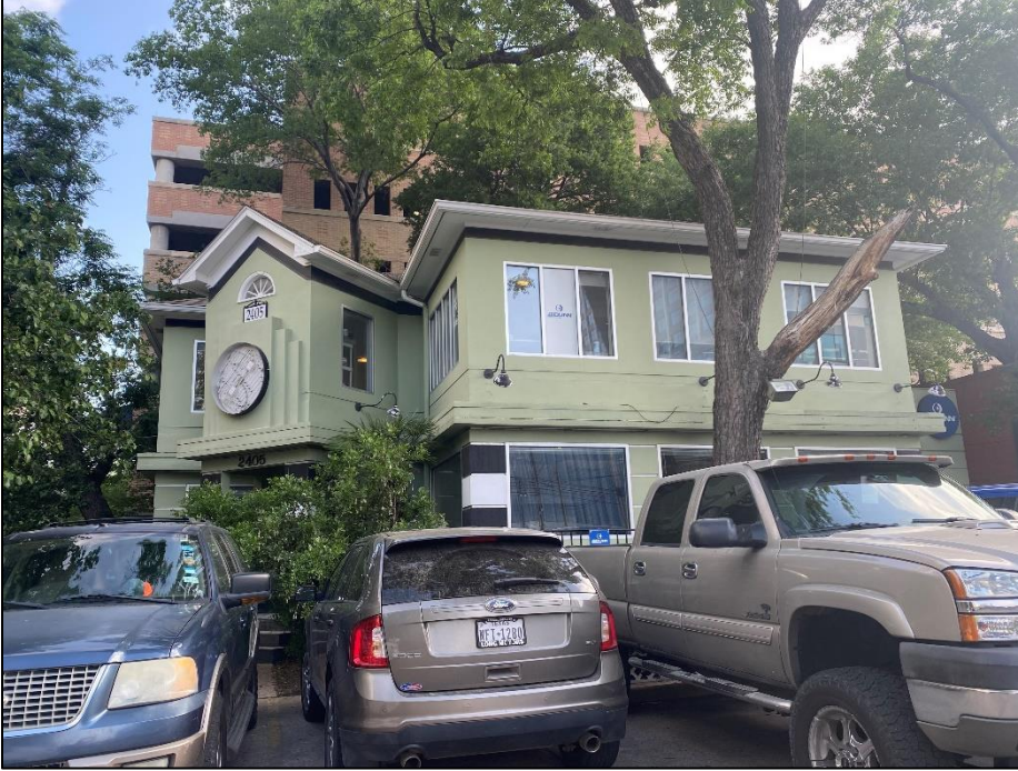
View of the south and southwest elevations, looking north.
