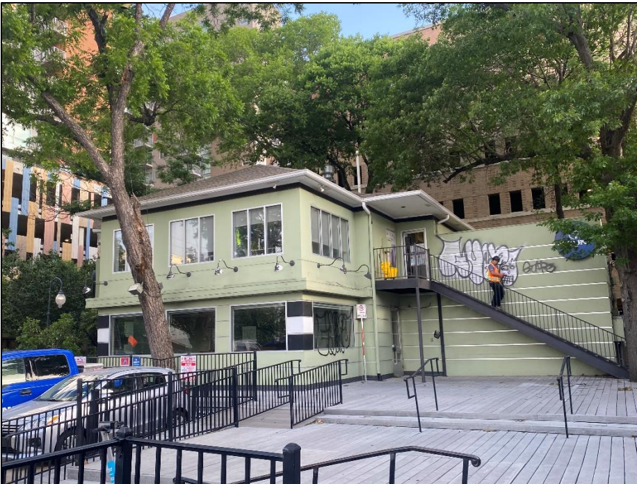
View of the south elevation, looking northwest.
