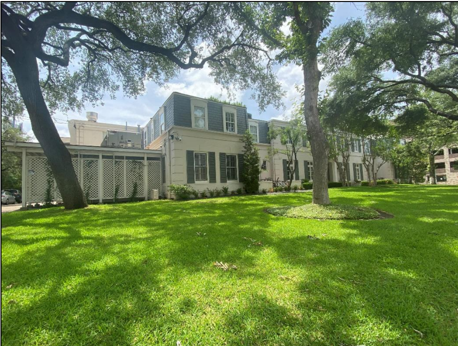
View of the façade, looking southwest (IMG_1315).
