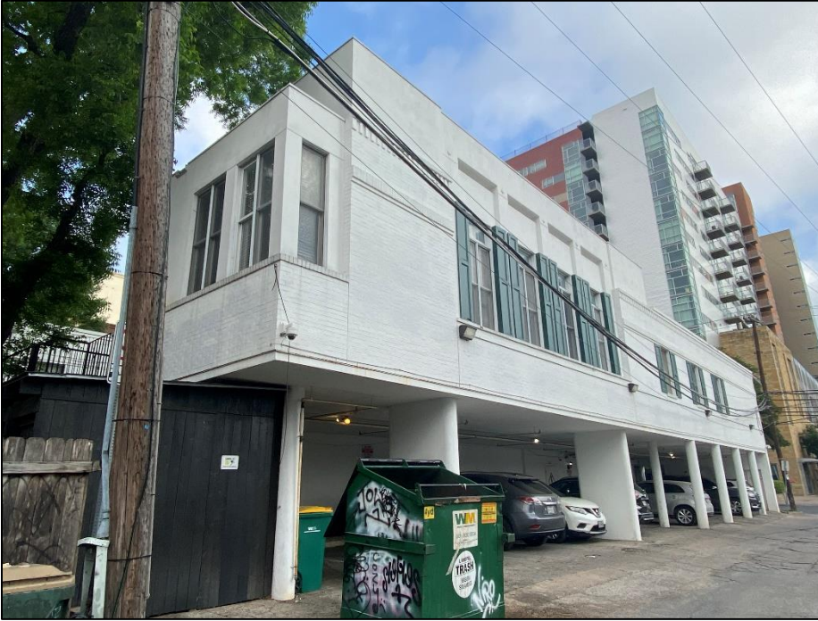
View of the rear (east) elevation of Resource S154, looking northwest.
