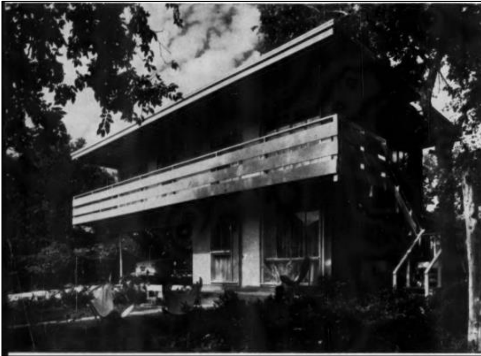
Oblique view of the façade and northeast elevation of Resource S114b in 1955, looking west (American Builder 1955).
