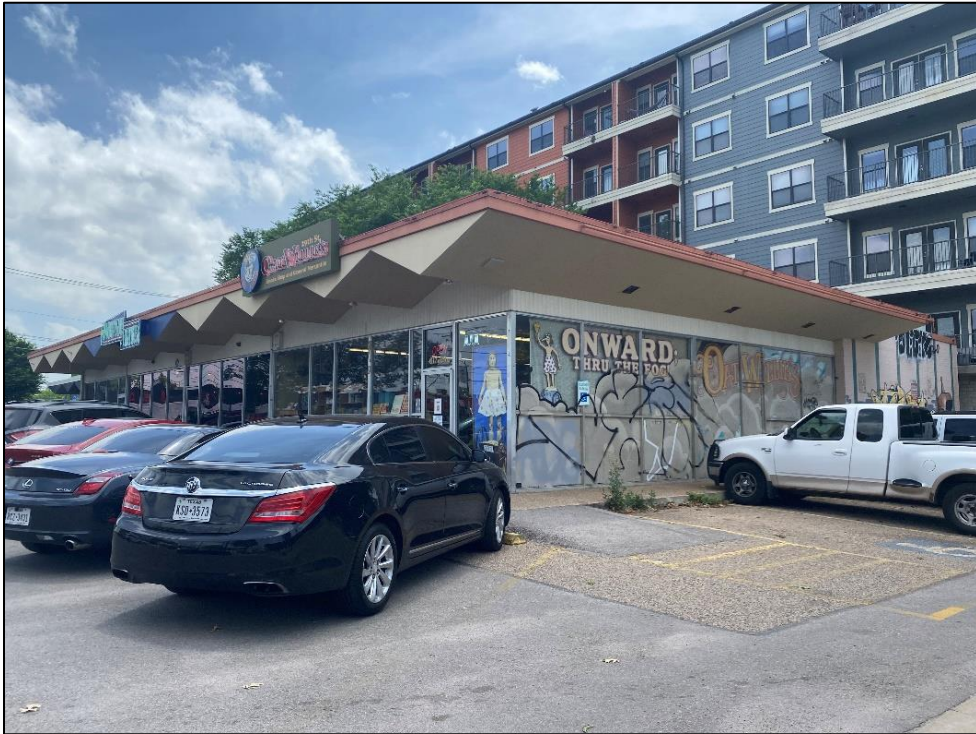
Oblique view of the west end of the façade and the west elevation of Resource S124, looking southeast.
