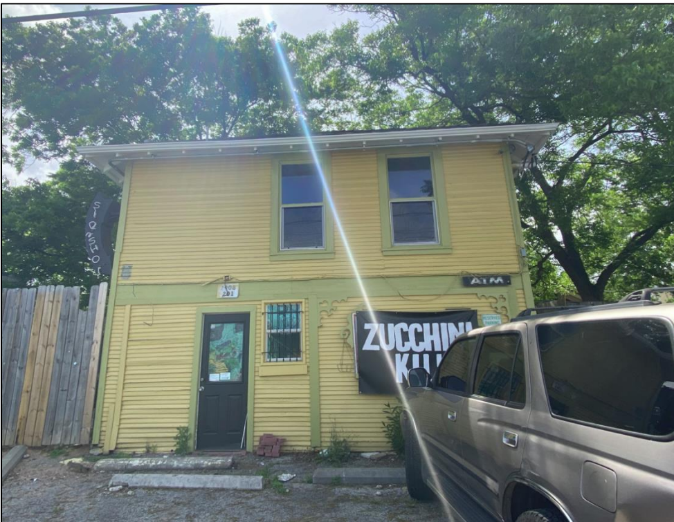
View of the rear (northwest) elevation of Resource S123b, looking southeast.
