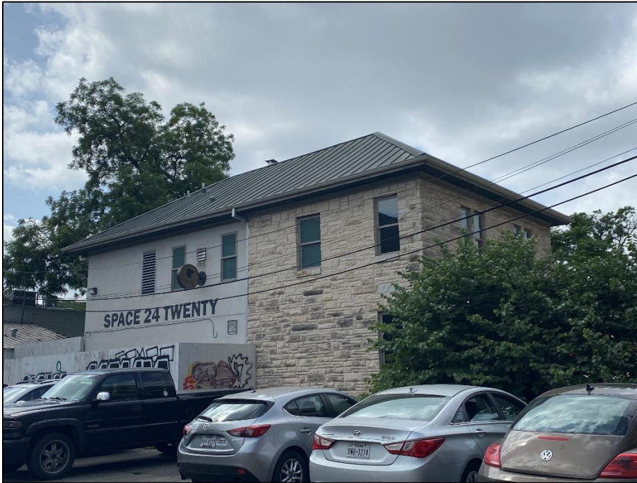
View of the north elevation of Resource S150, looking southeast.
