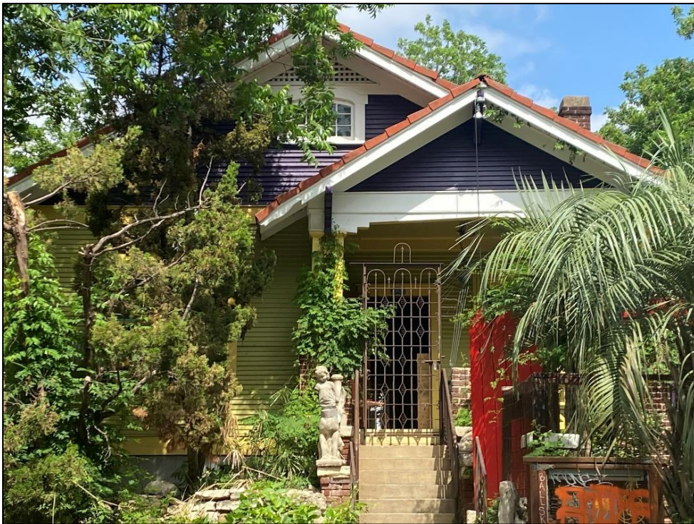
Façade view of Resource S123a, looking northwest.
