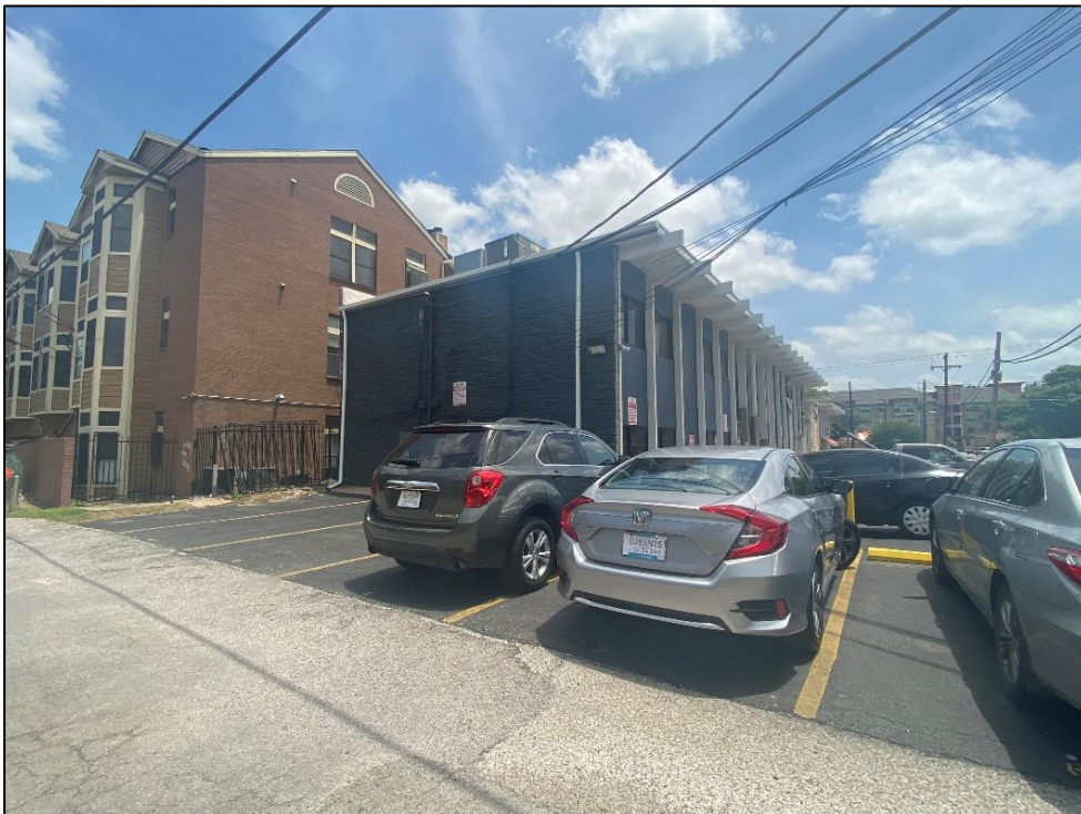
Oblique view of the west elevation and façade of Resource S133, looking east.
