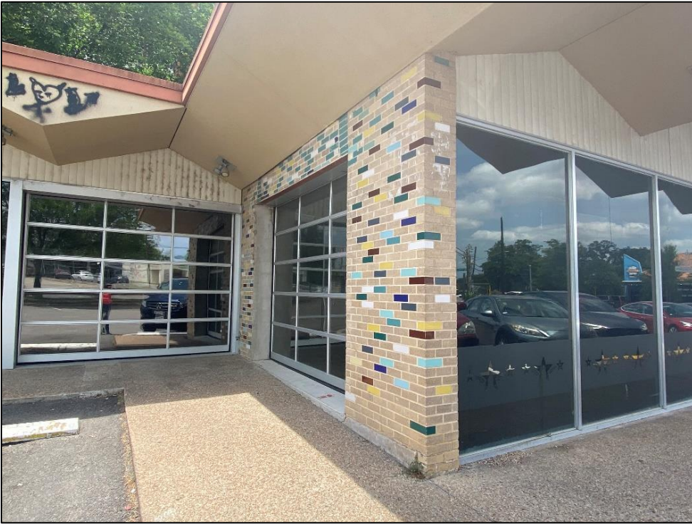
View of the replacement glazed roll-up doors on the façade of Resource S124, looking south.
