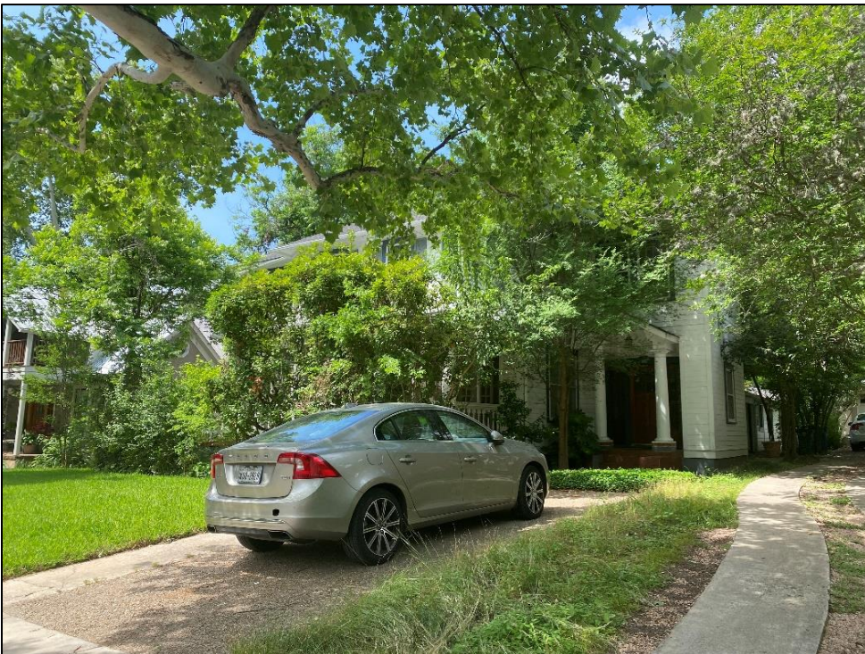
Façade view of Resource S113, looking southwest.
