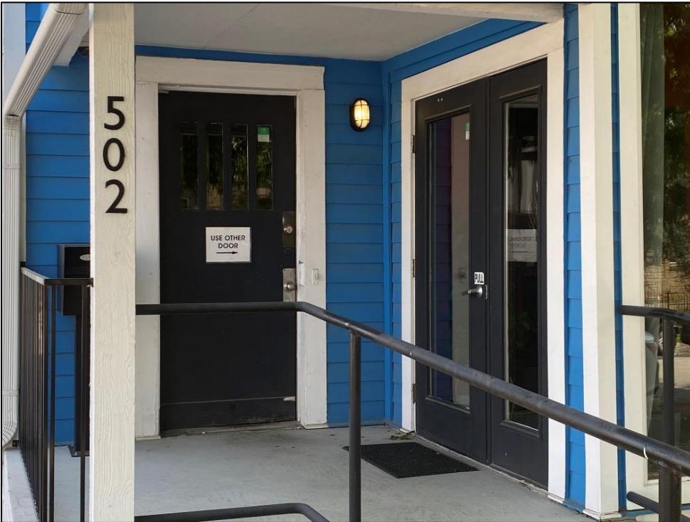
Detail of façade entry, Resource S117, looking north-northeast.
