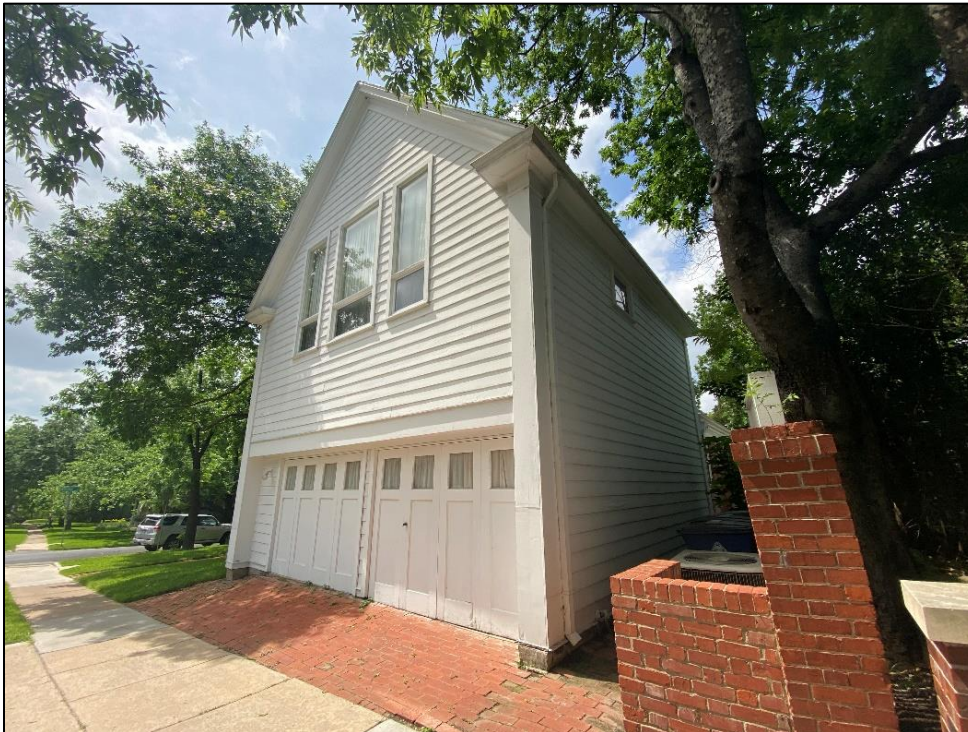
Oblique view of the façade and west elevation of Resource S108b, looking south-southeast.
