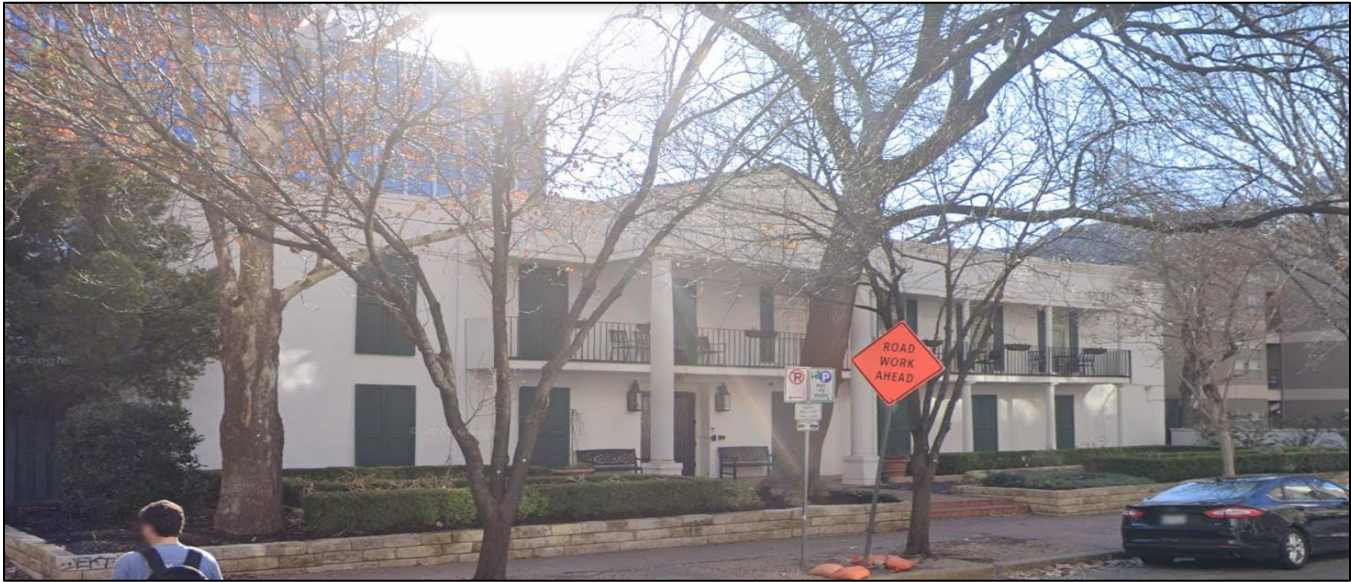
2022 view of the façade of Resource S154, looking southeast (Google Image 2022).
