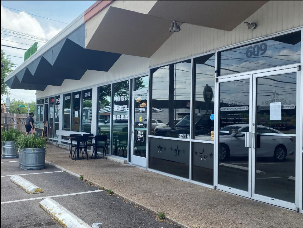
View of the east end of the façade of Resource S124, looking southeast.
