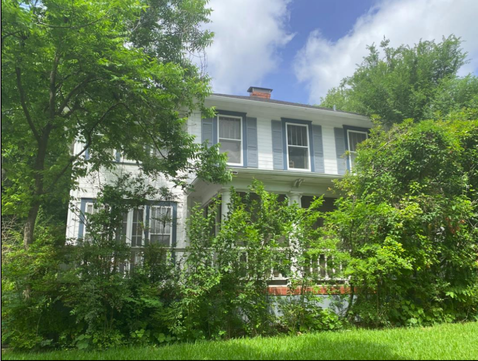
Façade view of Resource S113, looking southwest.
