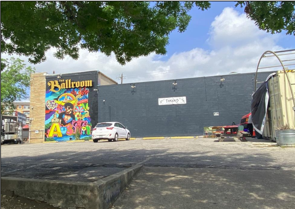
View of the southeast elevation of Resource S125, looking northwest.
