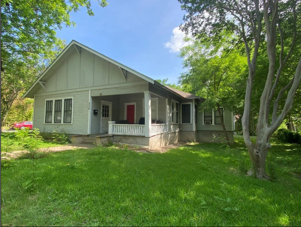
Oblique view of the façade and southeast elevation of Resource S119a, looking north.
