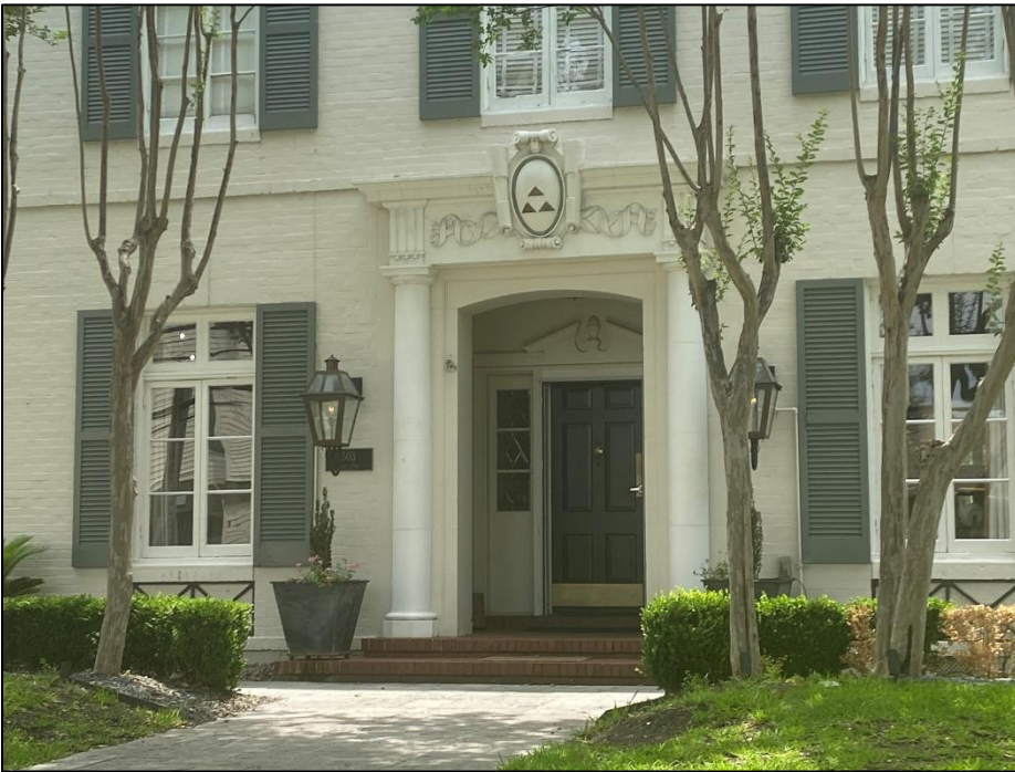
Detail of the façade entry, looking south (IMG_1319).
