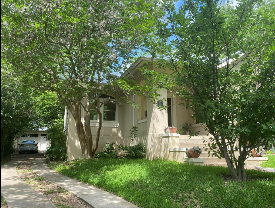
View of the façade of Resource S112b and an oblique view of the south elevation and façade of Resource S112a, looking west-southwest.
