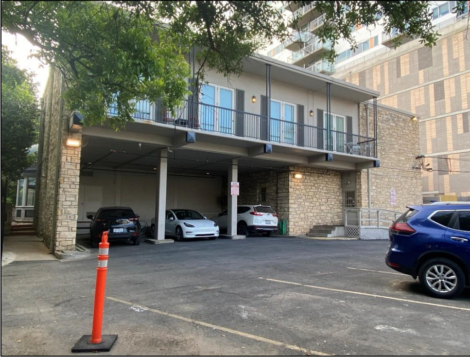
View of the rear (west) elevation of Resource S149, looking southeast.
