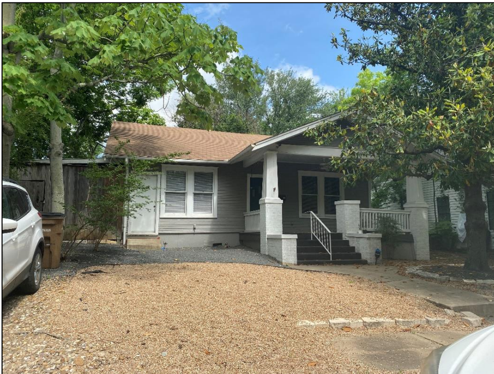
Façade view of Resource S116a, looking northwest.
