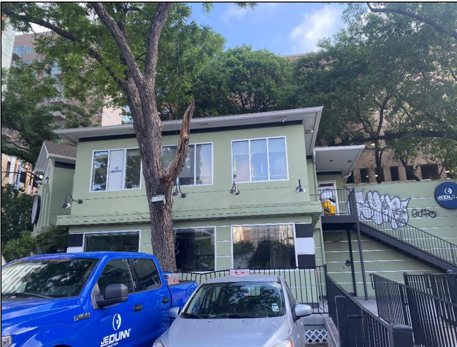
View of the south elevation, looking north.
