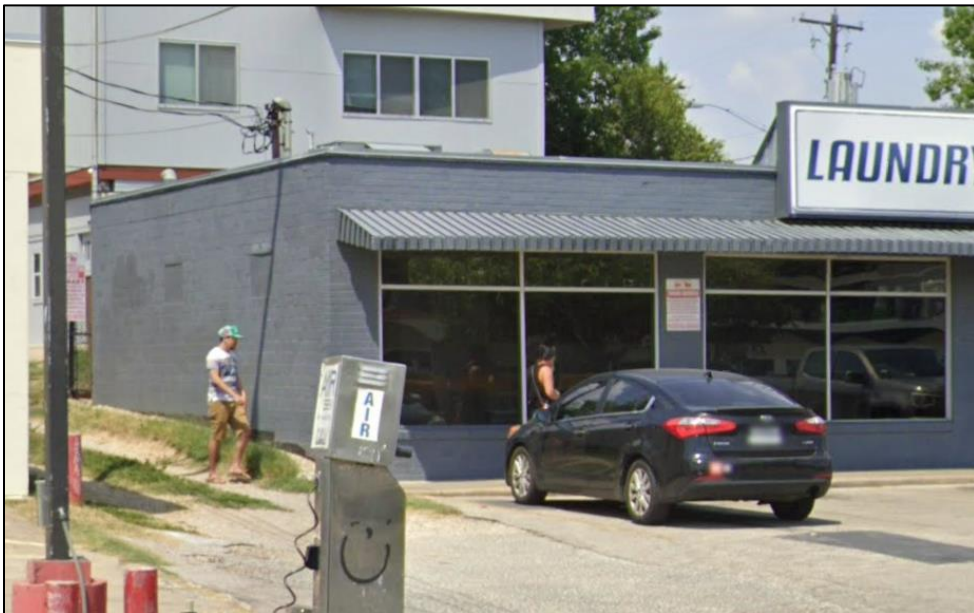
Oblique view of the northwest elevation and façade of Resource S120, looking north-northeast (Google Image Capture 07/2022).
