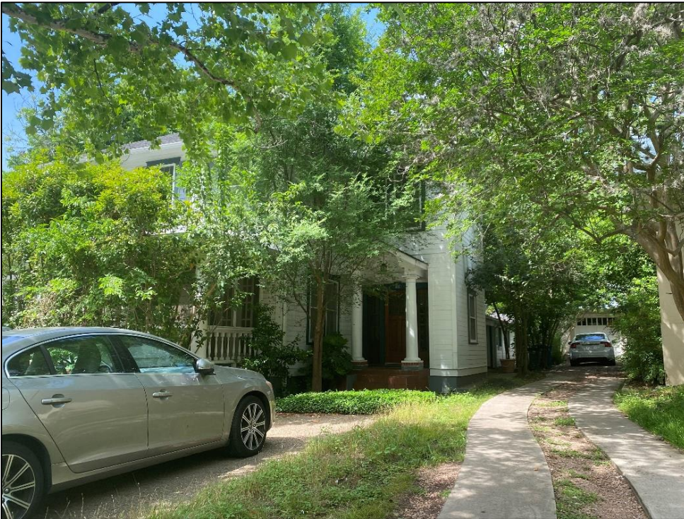
Oblique view of the façade and northwest elevation, looking southwest.
