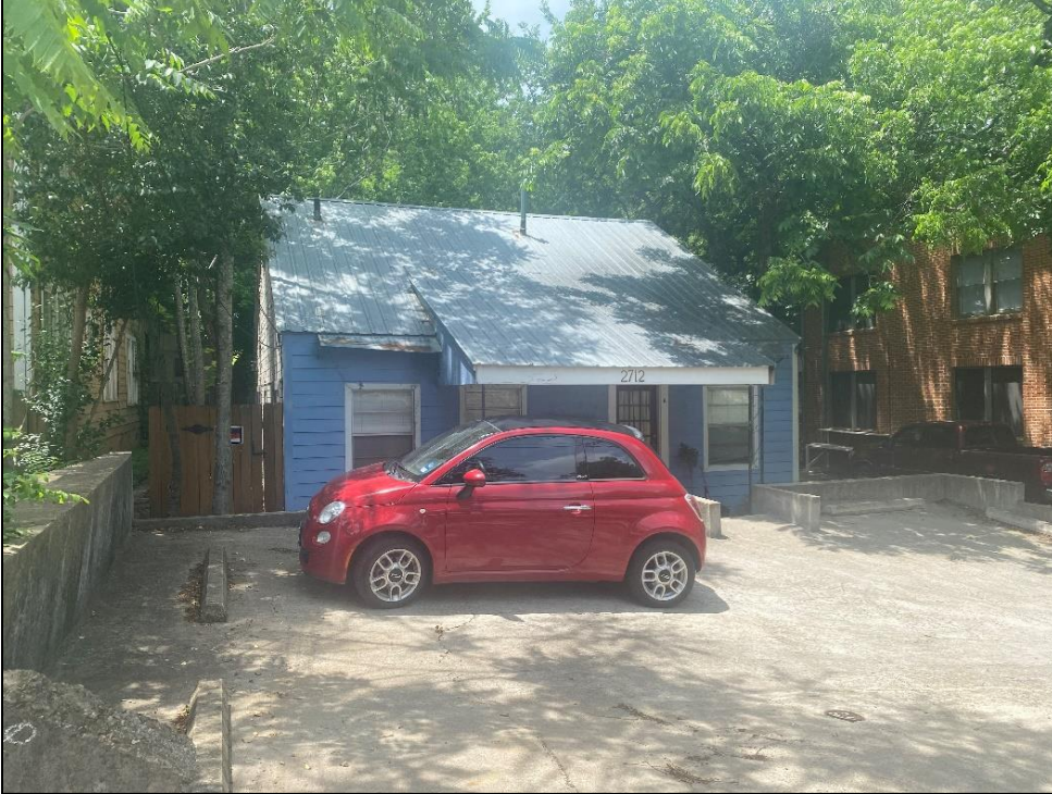
Oblique view of the south elevation and façade of Resource S139a, looking west.
