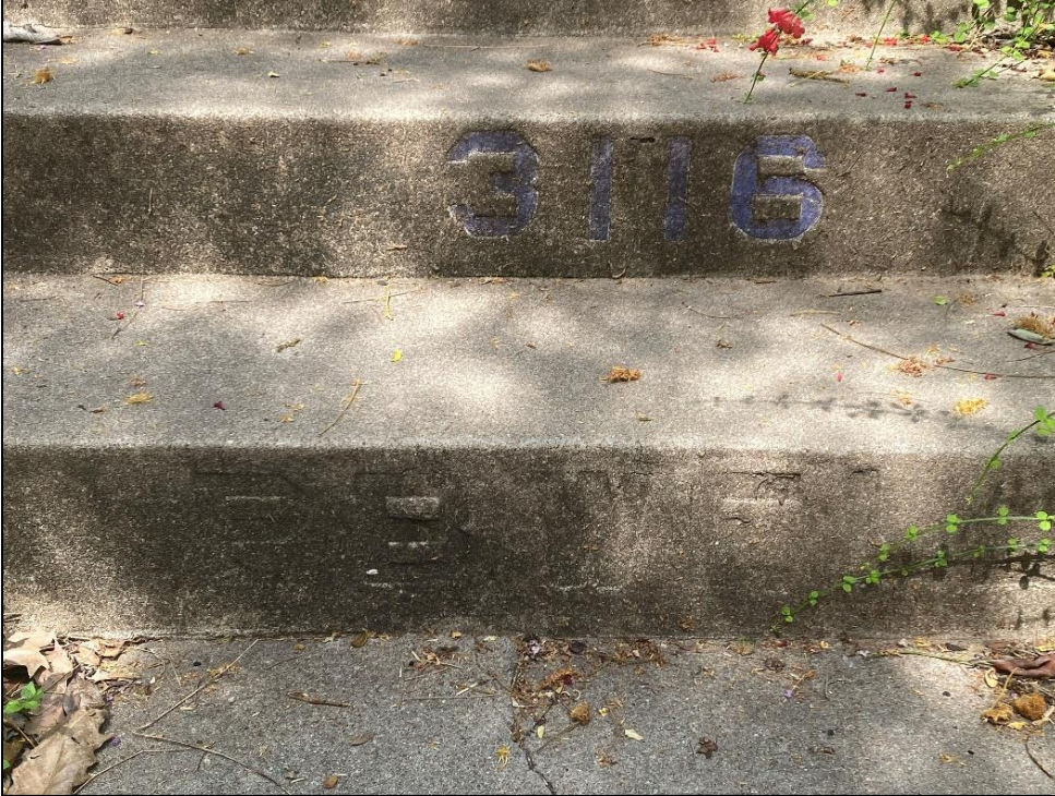
Detail of front steps, Resource S111, looking west.
