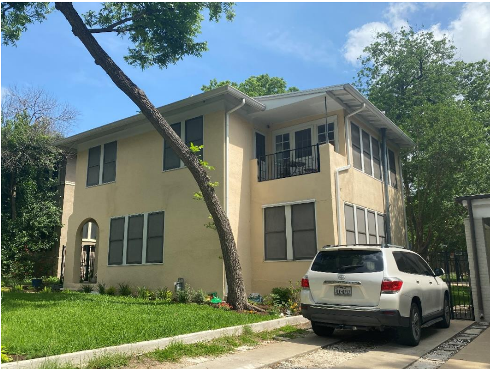
Oblique view of the façade and southeast elevation of Resource S107, looking north-northwest.
