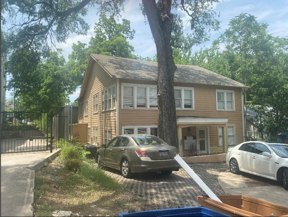
Oblique view of the south elevation and façade of Resource S141, looking northwest.
