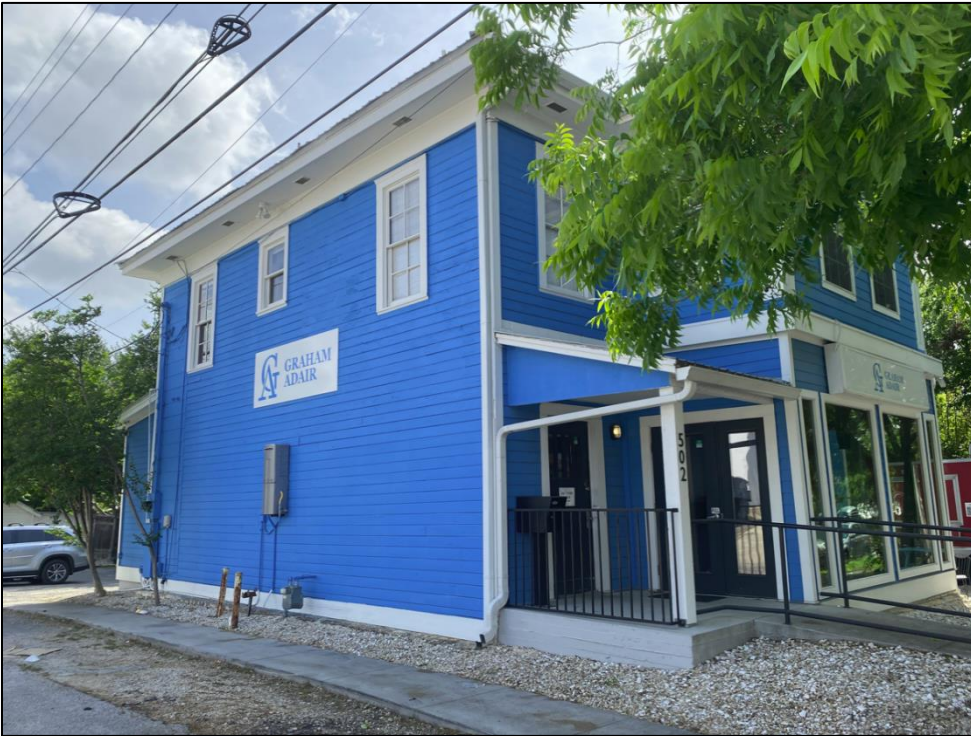
Oblique view of the northwest elevation and façade of Resource S117, looking northeast.
