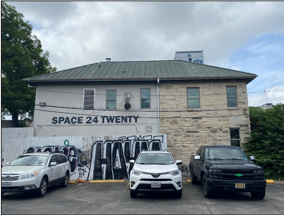
View of the north elevation of Resource S150, looking south.
