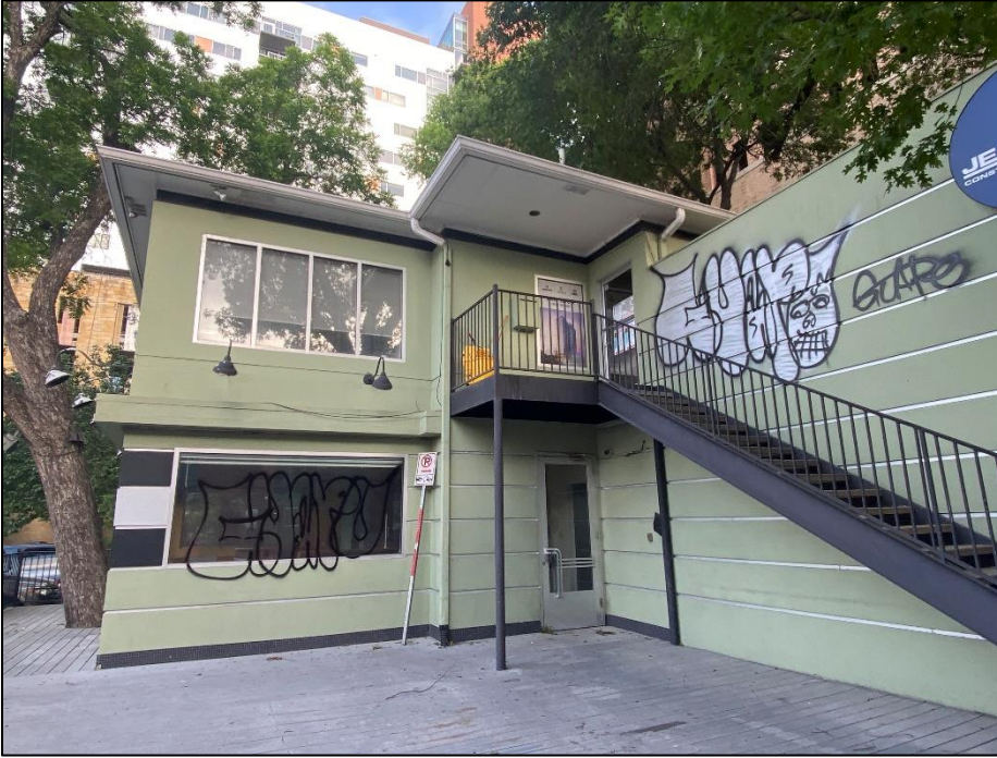
View of the east elevation, looking west.
