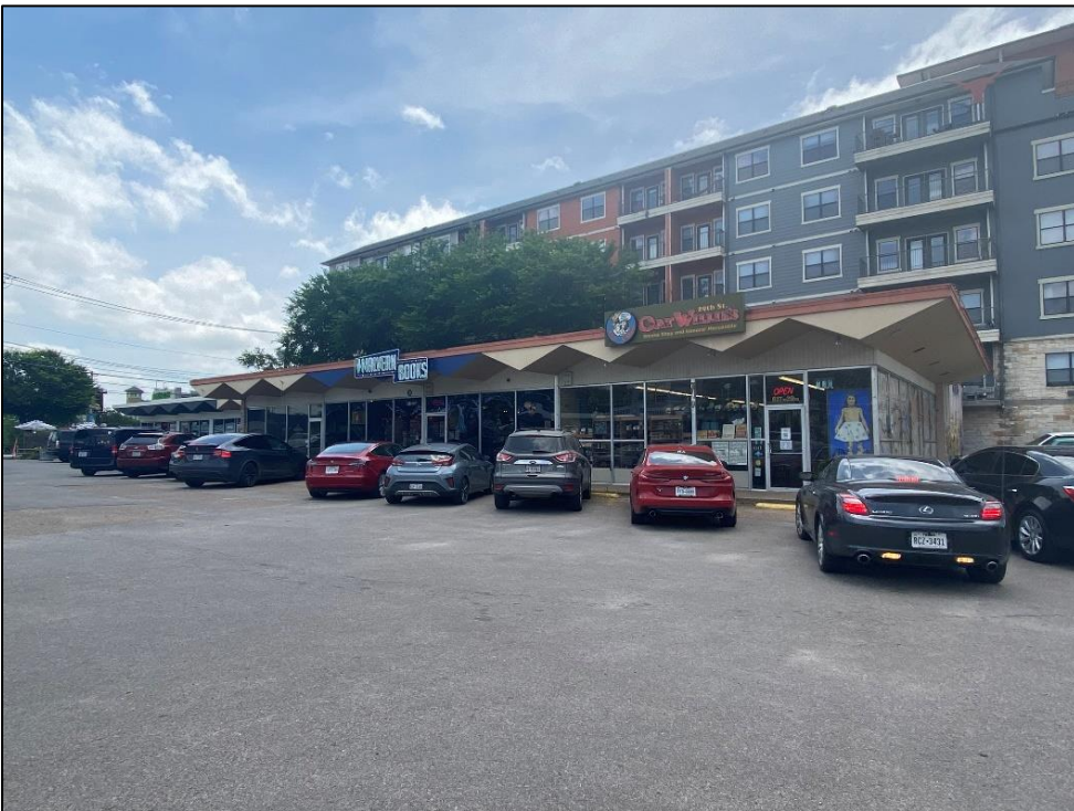
View of the west end of the façade and the west elevation of Resource S124, looking southeast.
