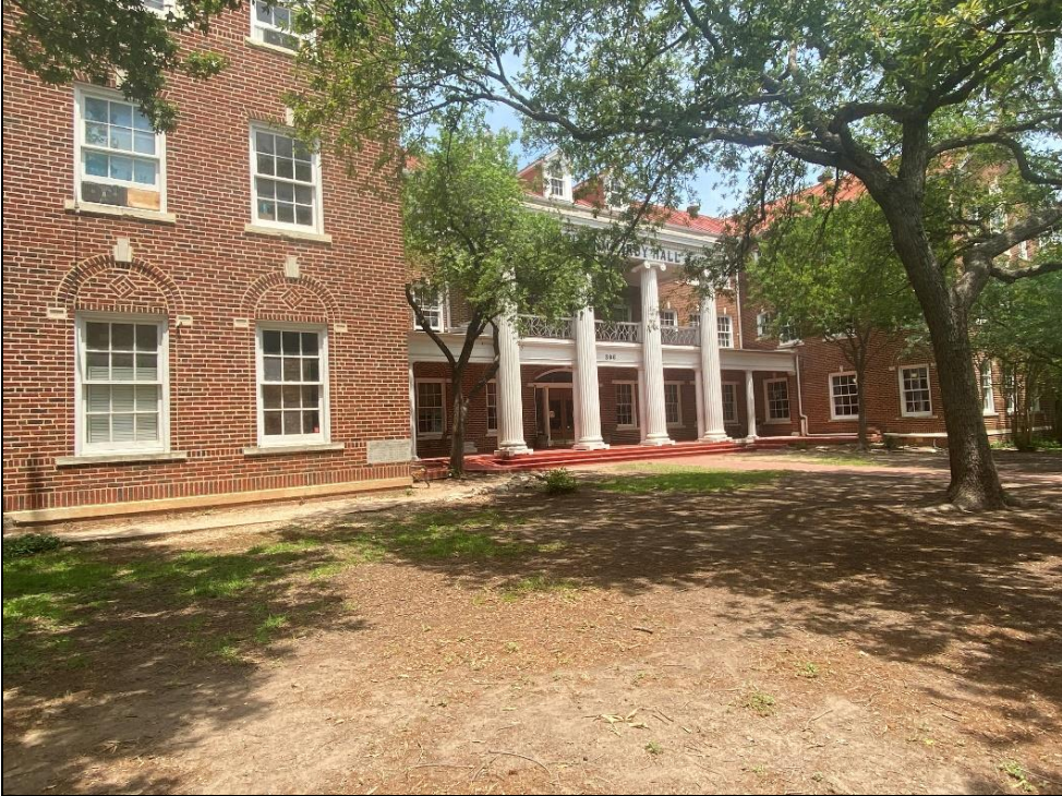
Oblique view of the façade and northwest elevations of Resource S126, looking northeast.
