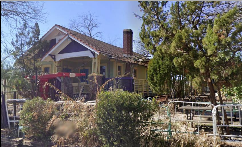
Oblique view of the façade and northeast elevation of Resource S123a, looking southwest (Google Image Capture 02/2022).
