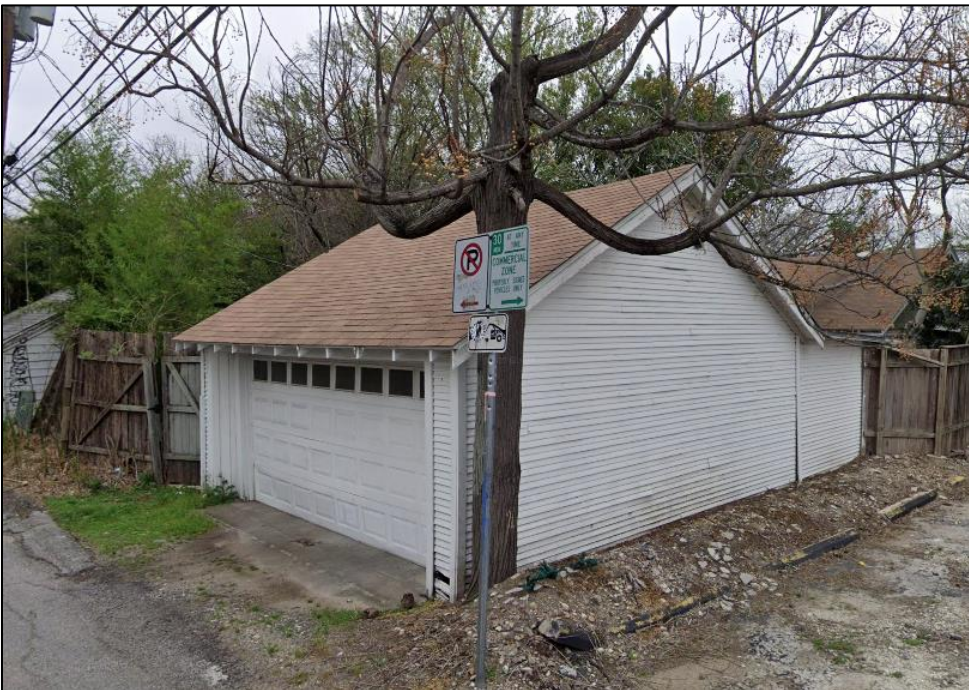
Oblique view of the current façade and southwest elevation of Resource S116b, looking northeast (Google Image Capture 03/2019).
