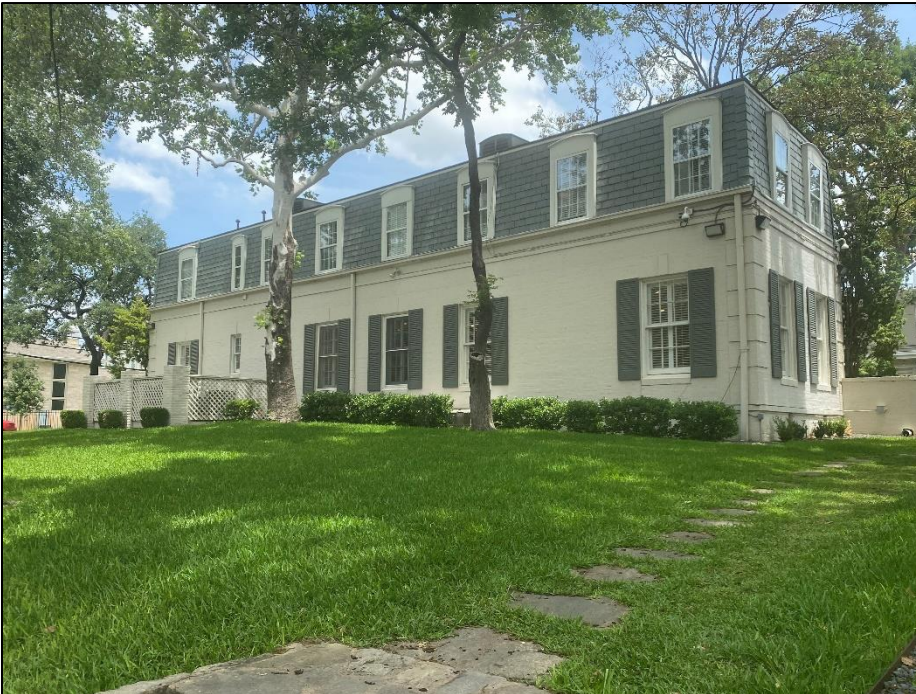
View of the west elevation, looking northeast (IMG_1312).
