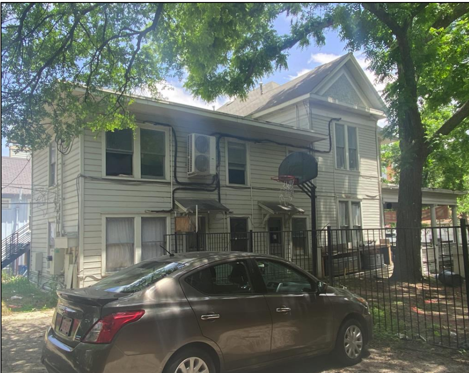
Oblique view of the rear (west) and south elevation of Resource S129a, looking northeast.
