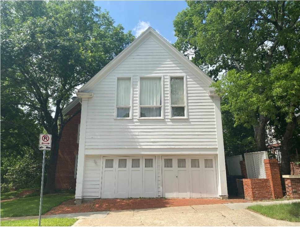
Façade view of Resource S108b, looking south-southwest.
