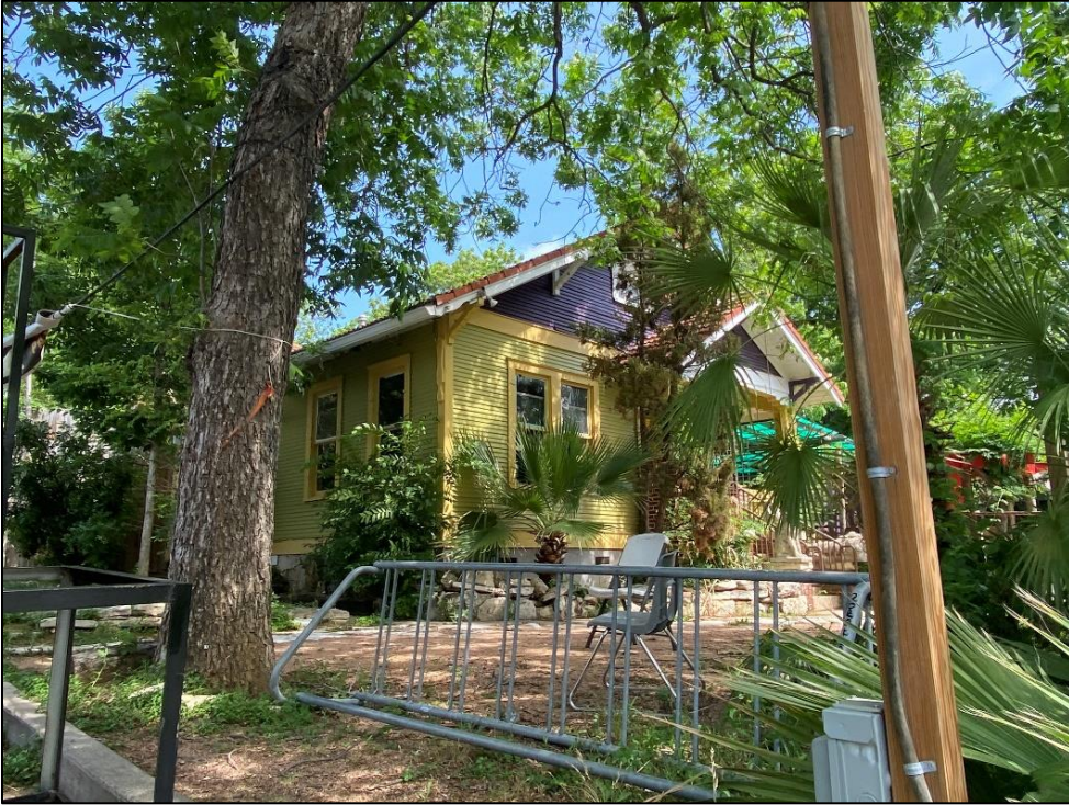
Oblique view of the southwest elevation and façade of Resource S123a, looking north-northwest.
