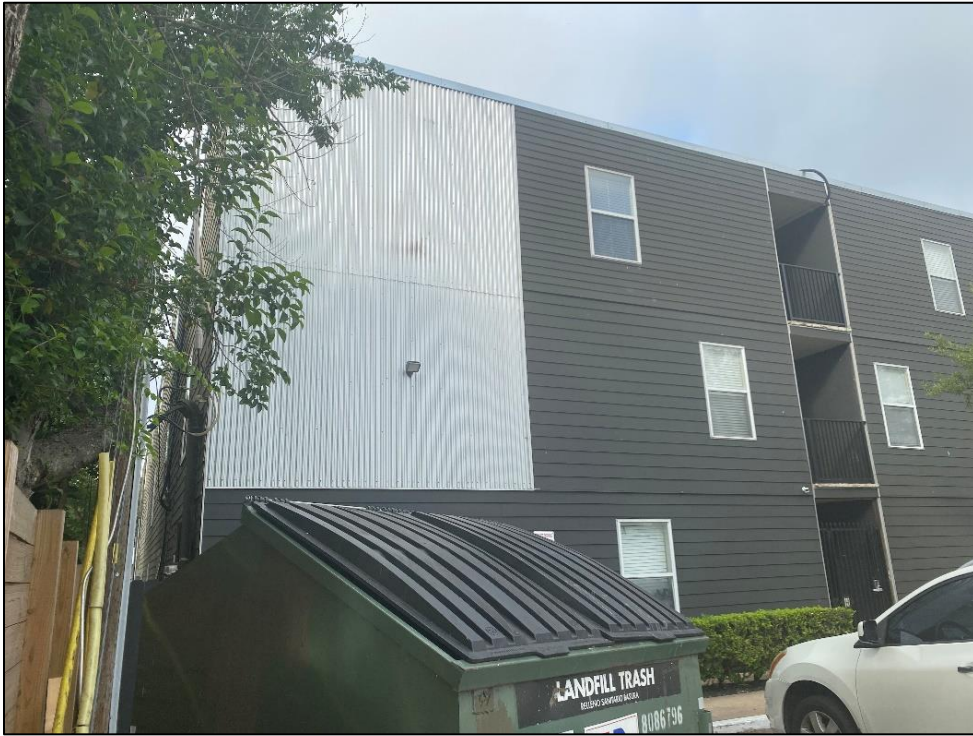
View of the southeast end of the façade of Resource S086, looking southwest.
