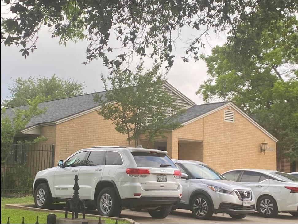
Oblique view of the southwest elevation and façade of the southwestern wing of Resource S090a, looking north.
