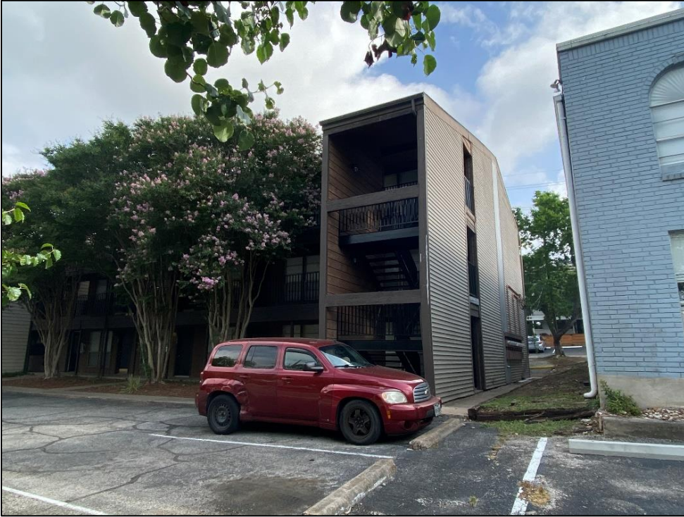
View of the southeast end of the façade and the southeast elevation of Resource S095, looking north-northwest.
