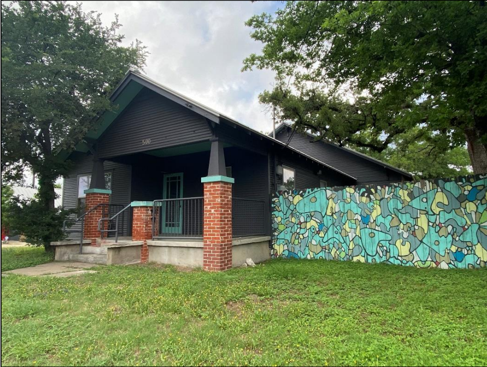
Oblique view of the façade and southeast elevation of Resource S089, looking northwest.
