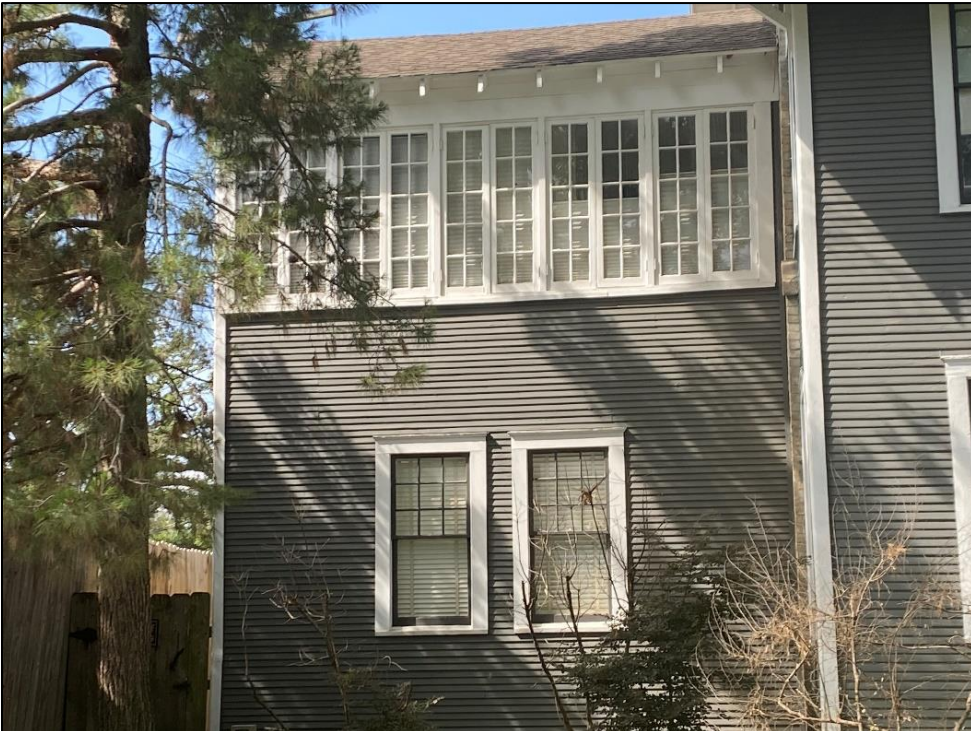
View of the southeast end of the façade, Resource S106a, looking southwest.
