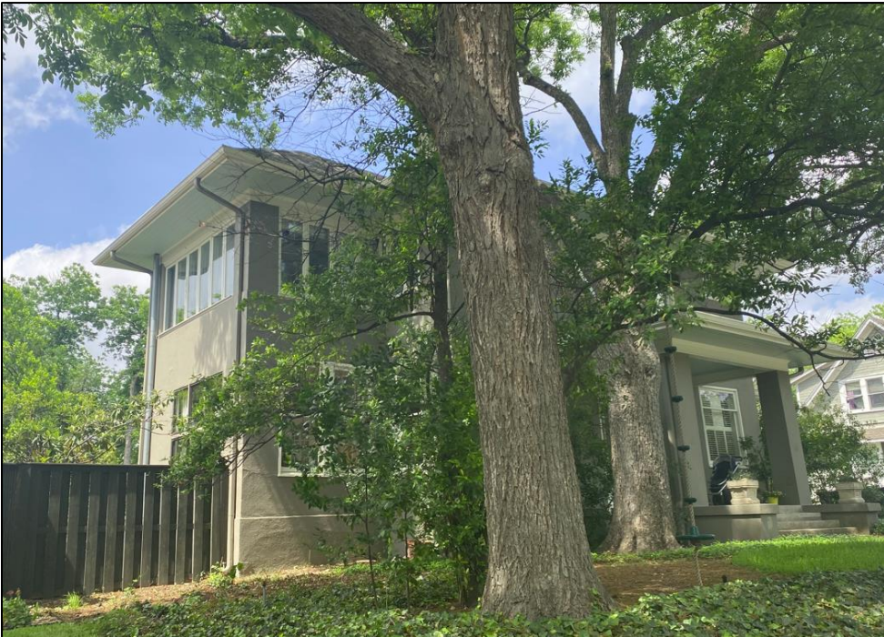
Oblique view of the southeast elevation and façade of Resource S105a, looking southwest.
