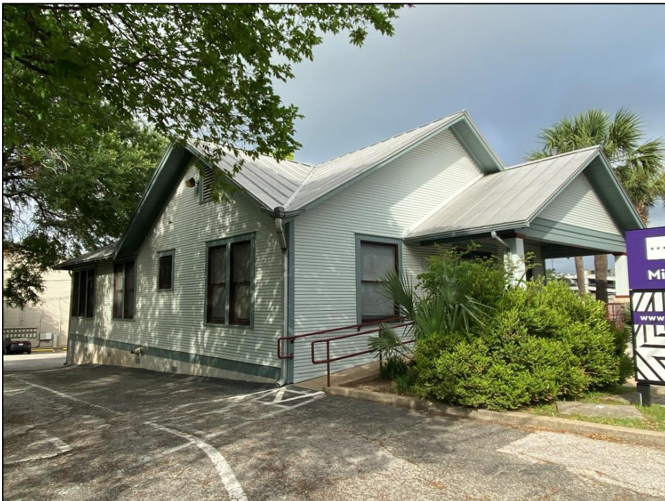
Oblique view of the southeast elevation and façade of Resource S091, looking southwest.
