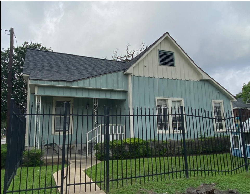
View of the northeast elevation of Resource S090b, looking southwest.
