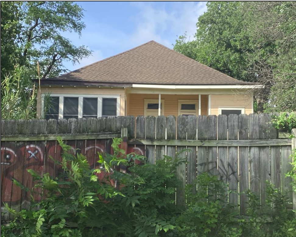
View of the rear (northeast) elevation of Resource S096, looking south-southwest.
