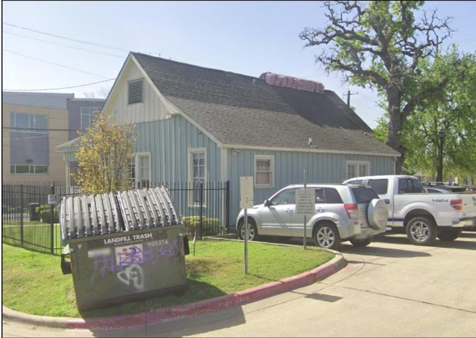
Oblique view of the northeast and rear (northwest) elevations of Resource S090b, looking south (Google Image Capture 04/2022),
