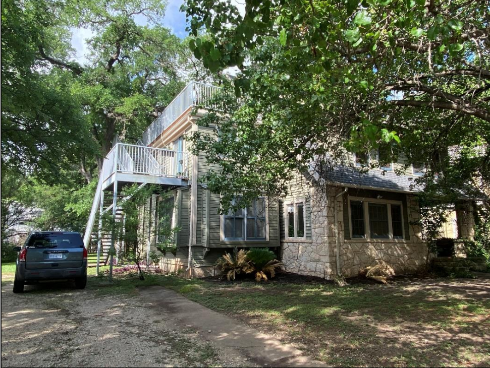
Oblique view of the southeast elevation and façade of Resource S102a, looking southwest.
