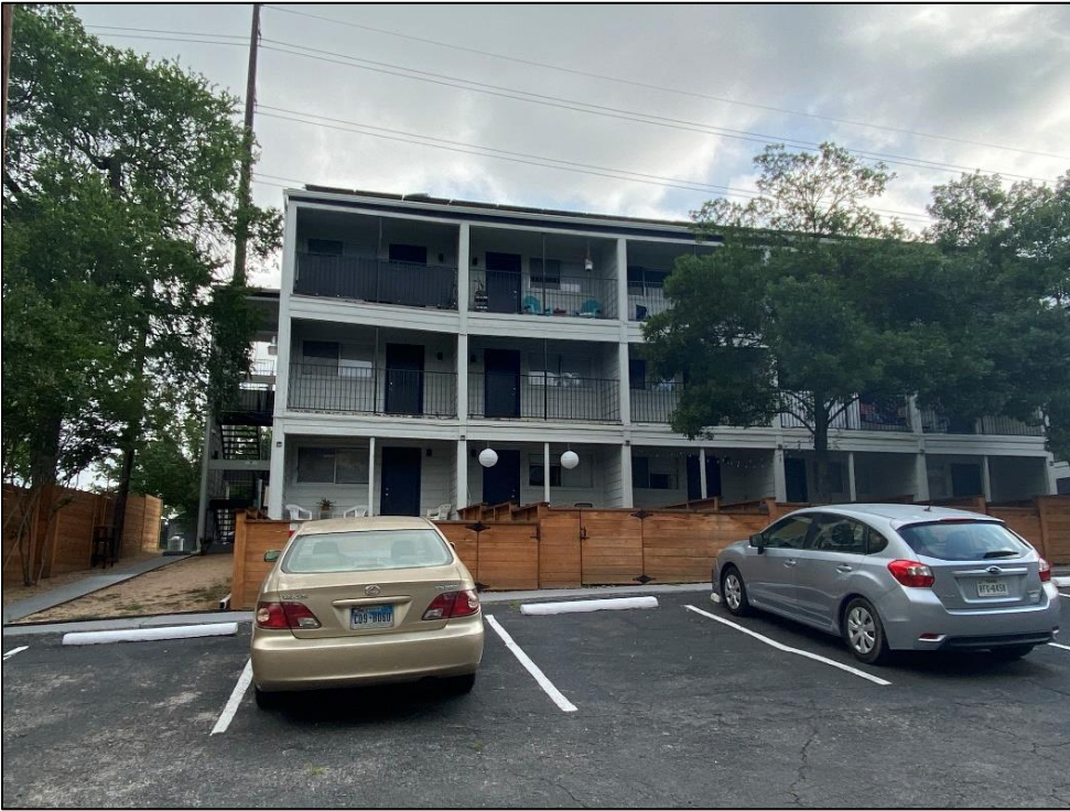
View of the rear (southwest) elevation of Resource S093, looking north-northeast.
