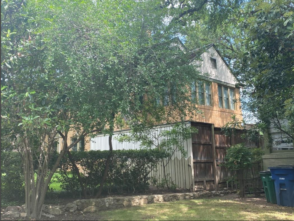
Oblique view of the façade and southeast elevation of Resource S103, looking north-northwest.
