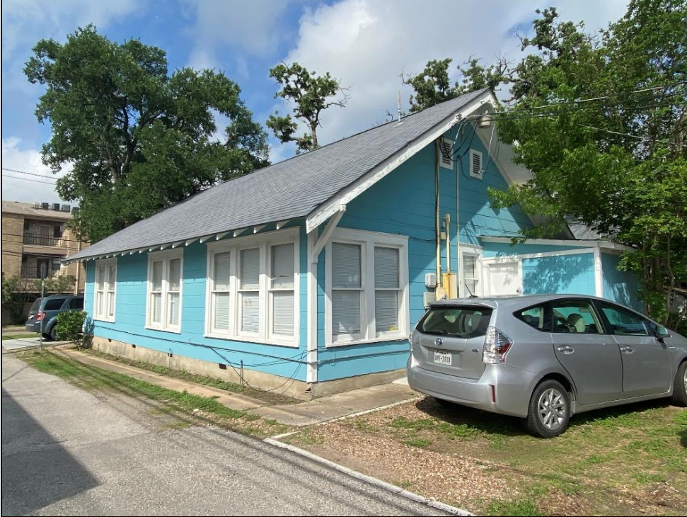
Oblique view of the southeast and rear (northeast) elevations of Resource S101a, looking southwest.
