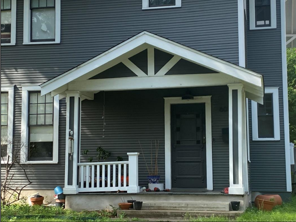
Detail of front porch, Resource S106a, looking southwest.
