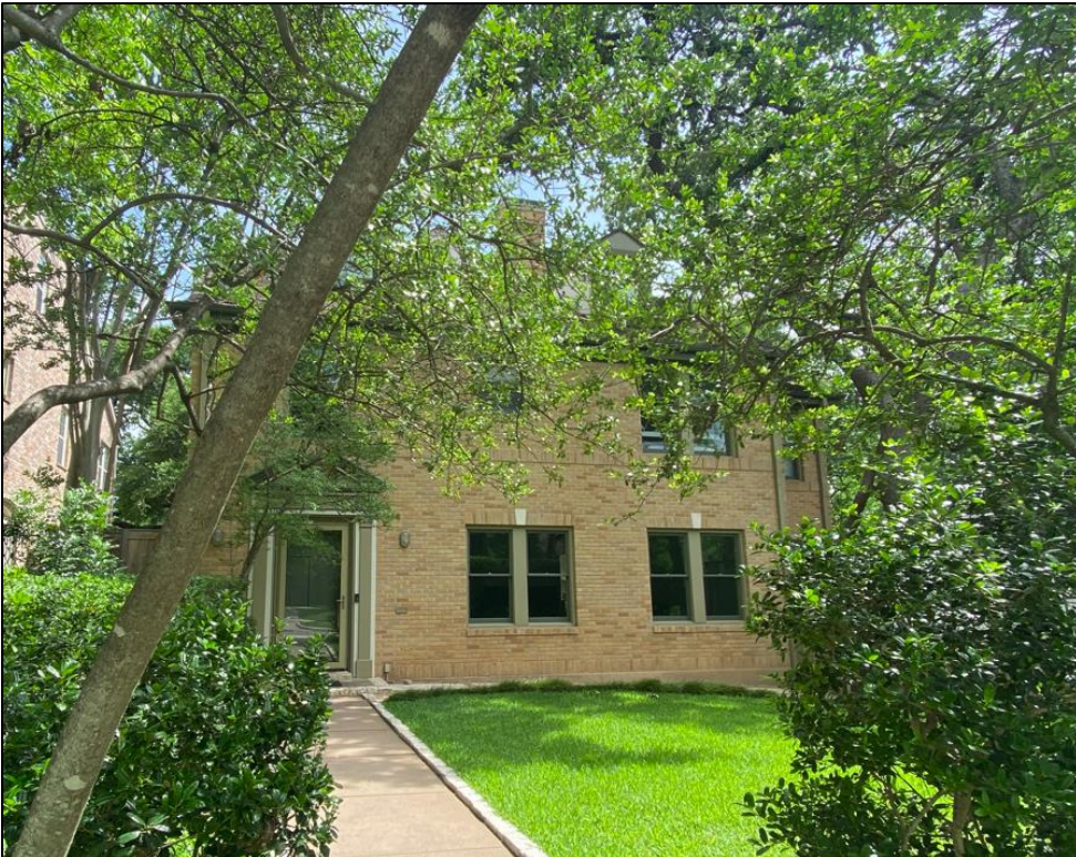
Façade view of Resource S103, looking northeast.
