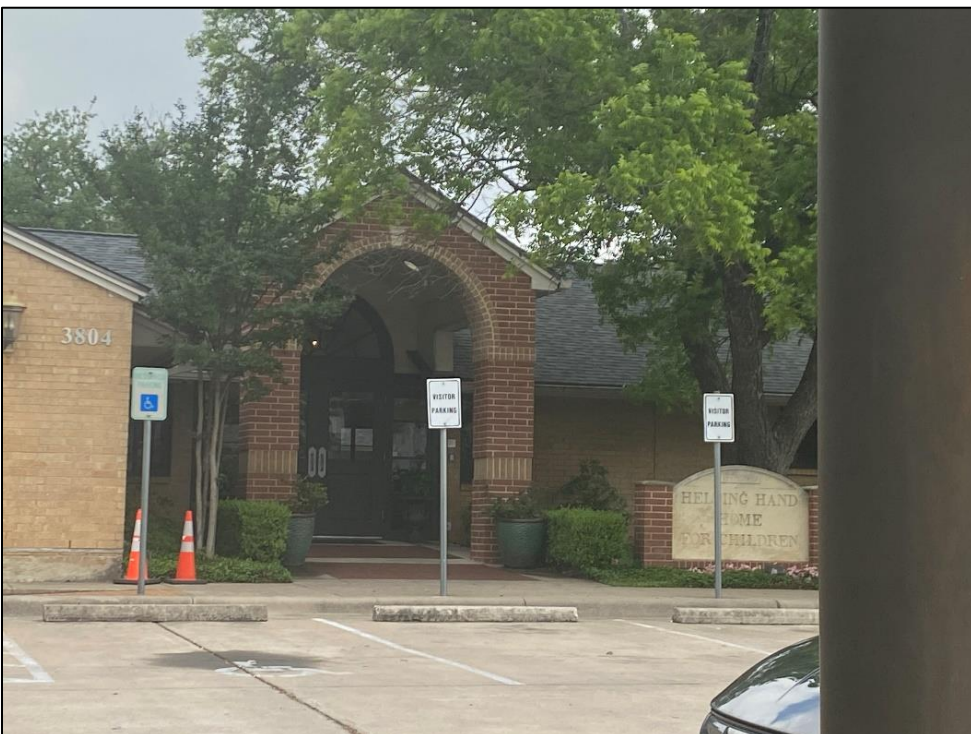
Detail of the primary entrance on the façade of Resource S090a, looking northwest.
