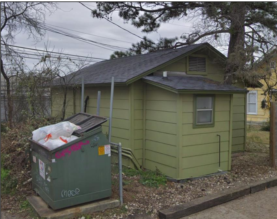
Oblique view of the rear (northeast) and northwest elevations of Resource S101b, looking southeast.
