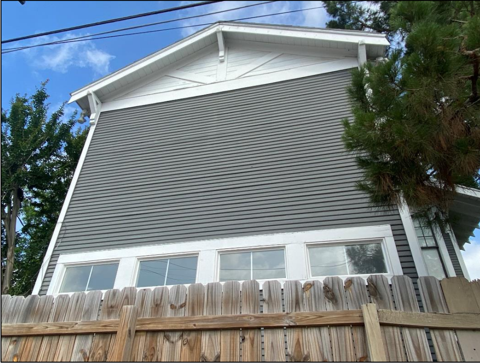
View of the southeast elevation of Resource S106a, looking northwest.
