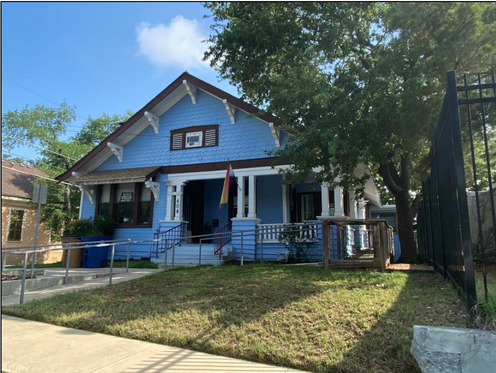
View of the façade and southeast elevation of Resource S097, looking north-northwest.
