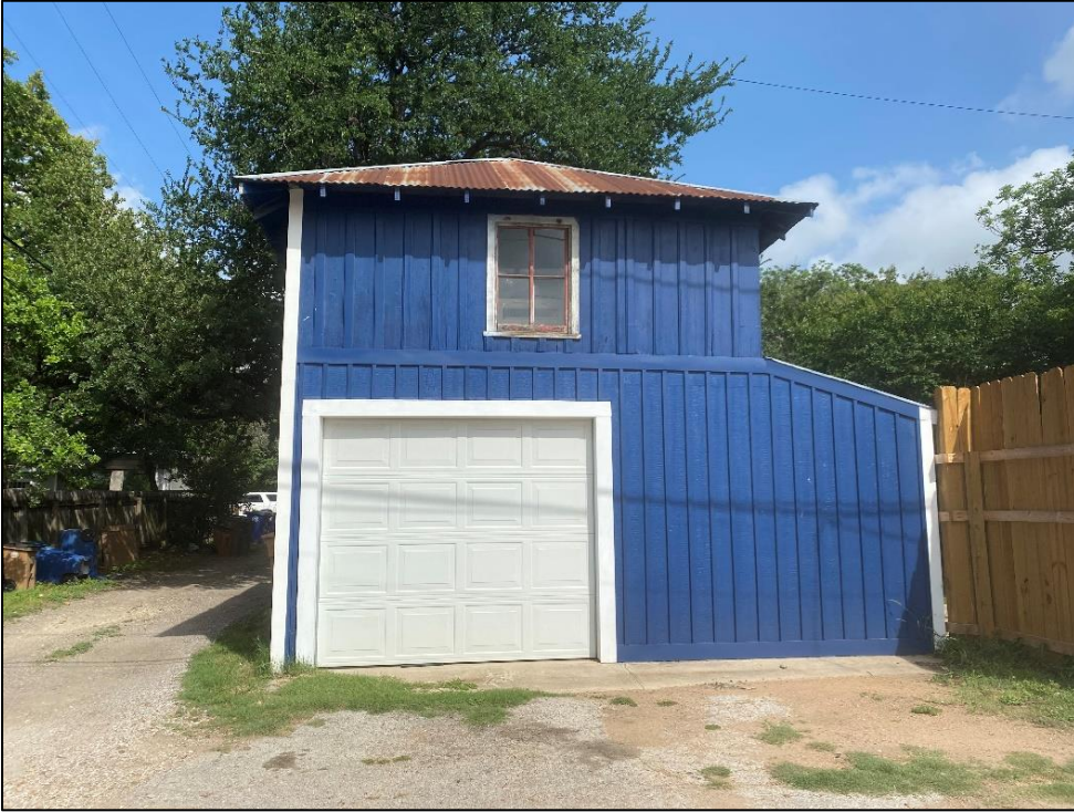
Façade view of Resource S106b, looking northwest.
