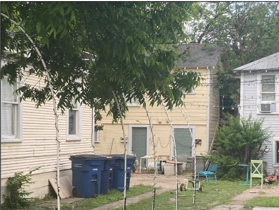
Partial view of the northwest elevation of S099a and the façade and northwest elevation of Resource S099b, looking south.
