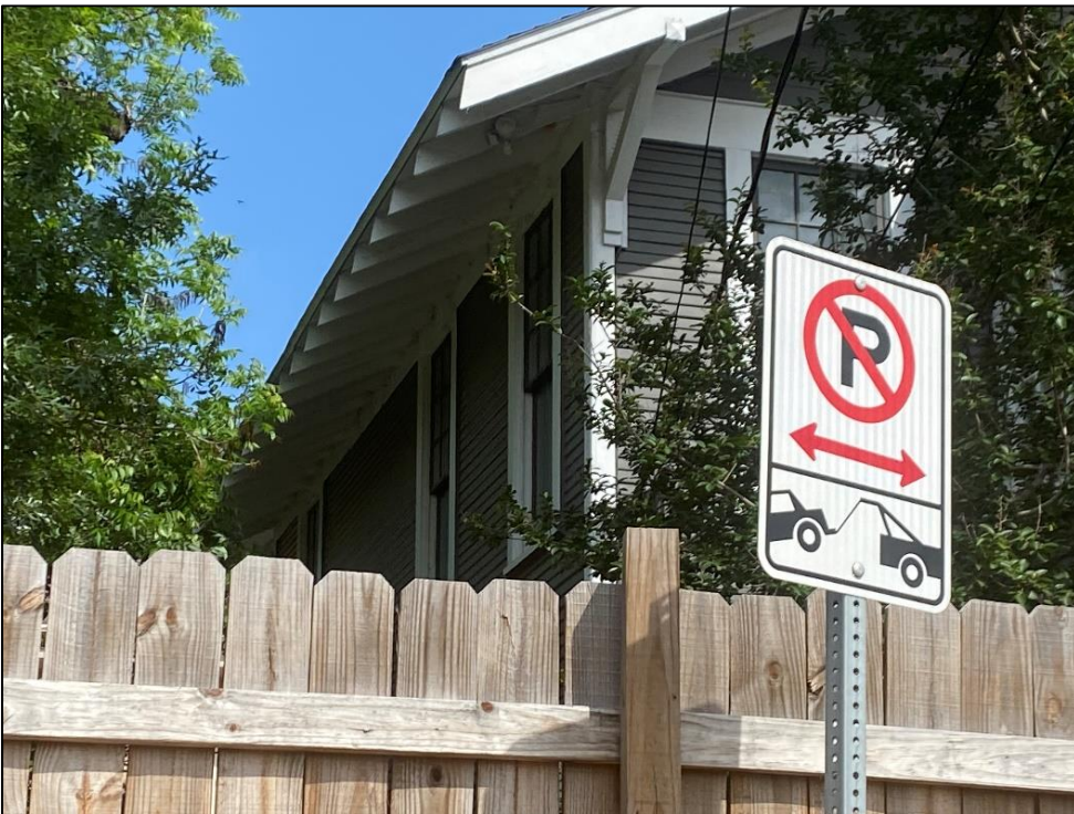
Oblique view of the rear (southwest) and southeast elevations of Resource S106a, looking northwest.
