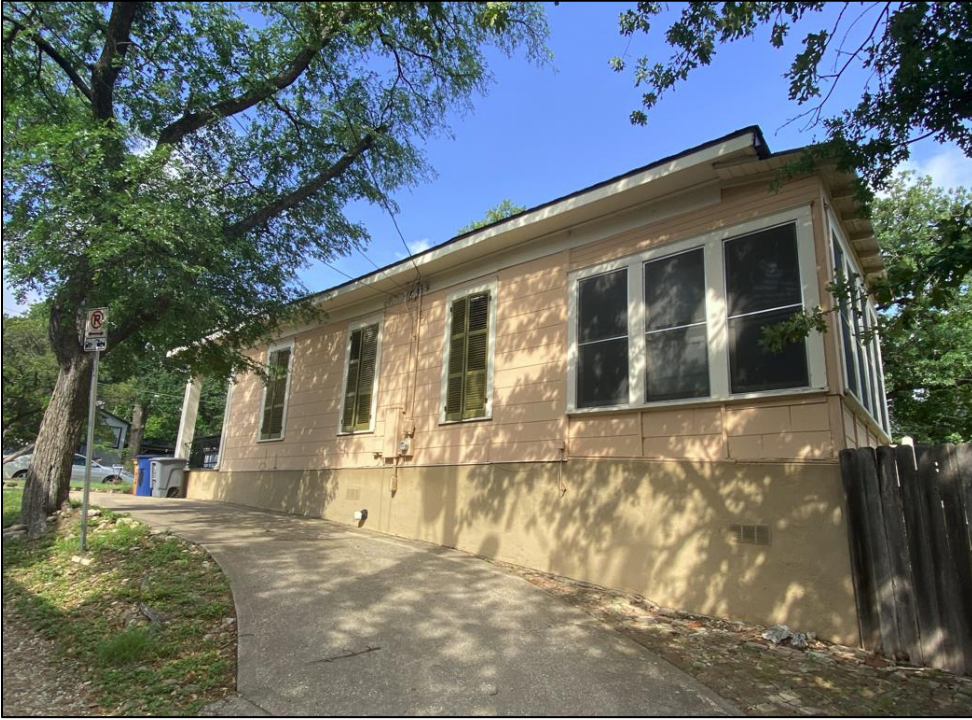
View of the southeast elevation of Resource S096, looking southwest.
