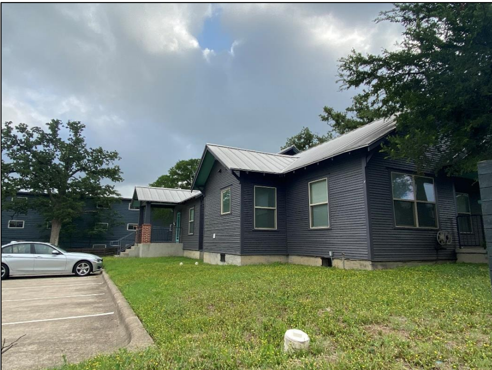
Oblique view of the northwest elevation and the façade of Resource S089, looking northeast.
