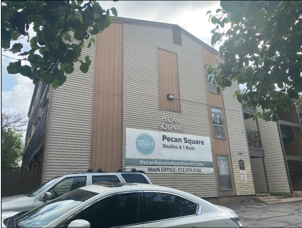
Oblique view of the northwest elevation and the façade of Resource S095, looking northeast.
