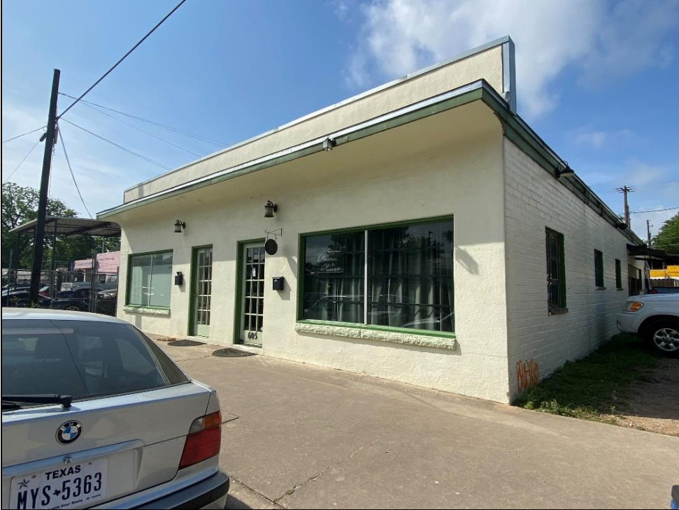
Oblique view of the façade and northwest elevation of Resource S092, looking south-southeast.
