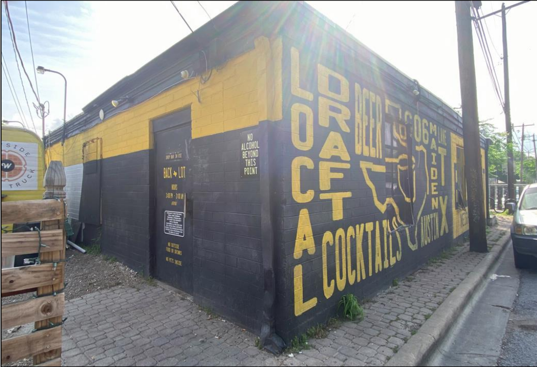
Oblique view of the rear (northwest) and southwest elevations of Resource S094, looking northeast.
