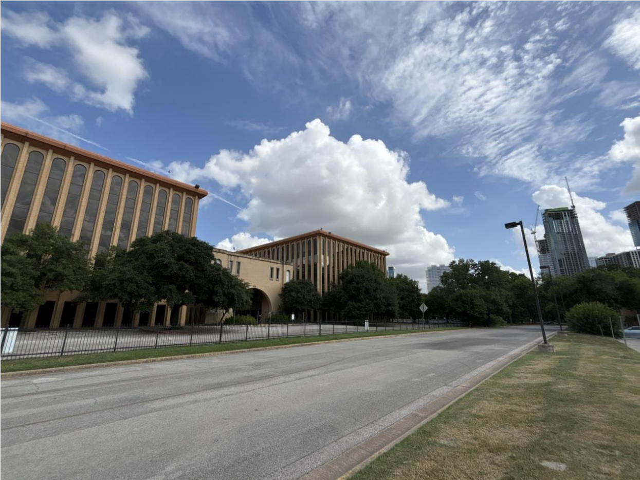
Figure 8: Existing Conditions of Area of Proposed Waterfront Station on East Riverside Drive Extension, Facing Northwest
